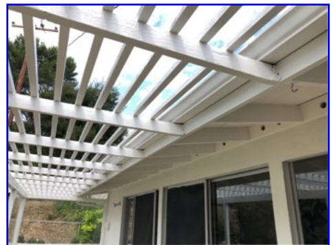
Attached to fascia
