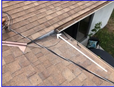
Missing flashing
