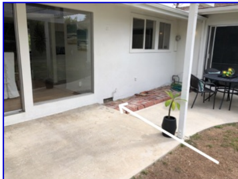
Grade above vents
