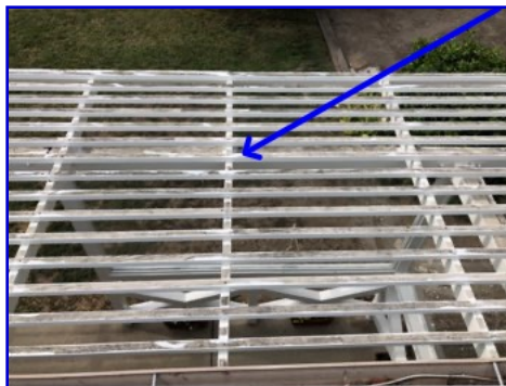
Deteriorated wood
