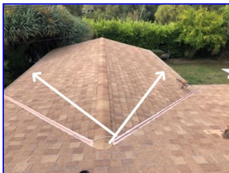
Poor drainage
