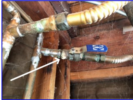
Shutoff corroded
