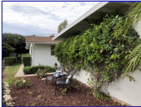
Vegetation too close
