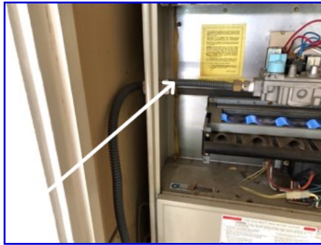
Flex through sheet metal
