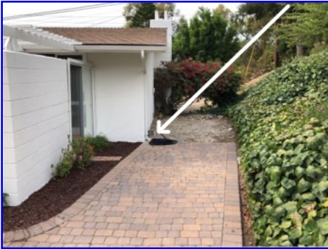
MAIN WATER VALVE LOCATION
