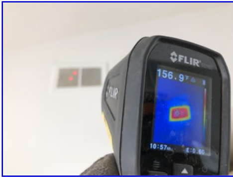
Thermal Image View
