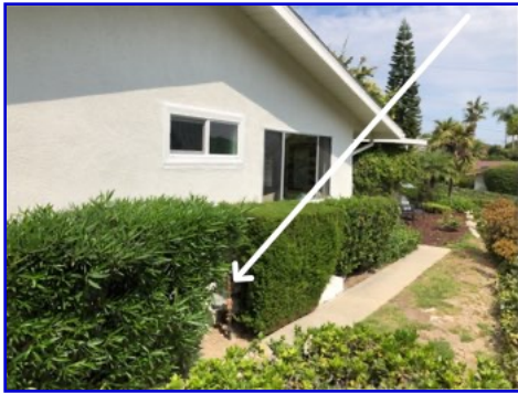
MAIN GAS VALVE LOCATION
