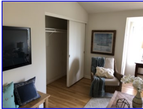
Missing base guides
