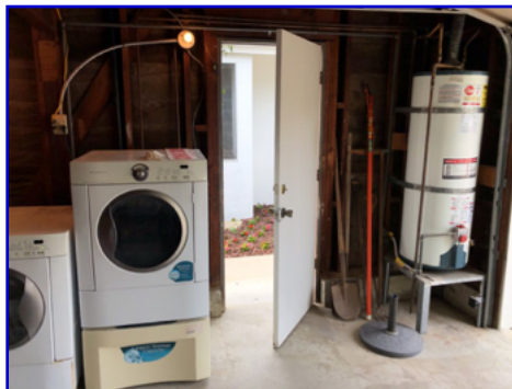
Weatherstripping, threshold missing; Attempted forced entry; Not latching
