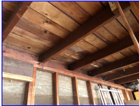
Moisture stains/damage
