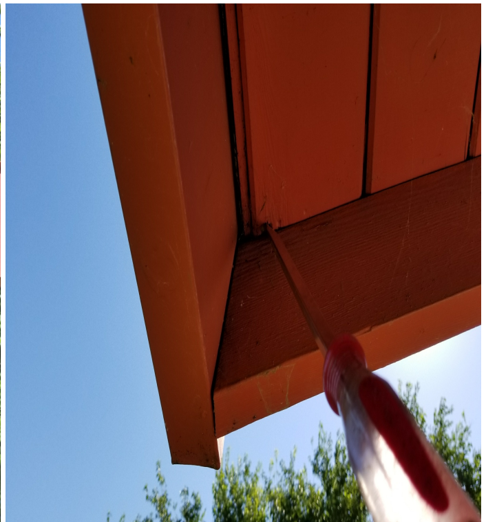
3 D - Damaged eaves.
