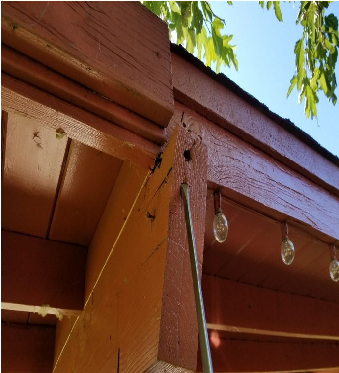
3 C - Damaged beam.
