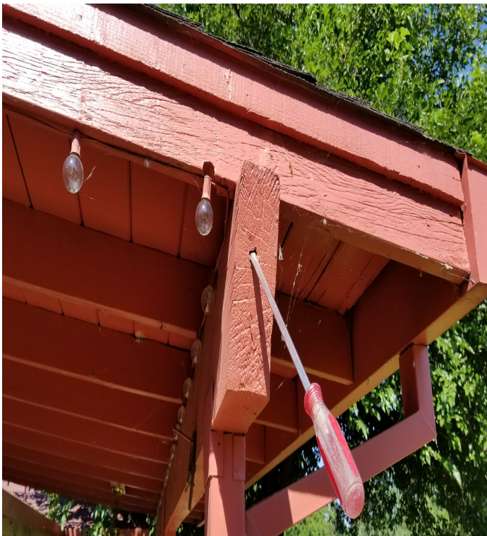
3 C - Damaged beam.
