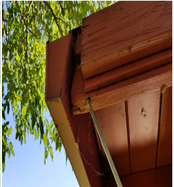
3 C - Damaged joist.
