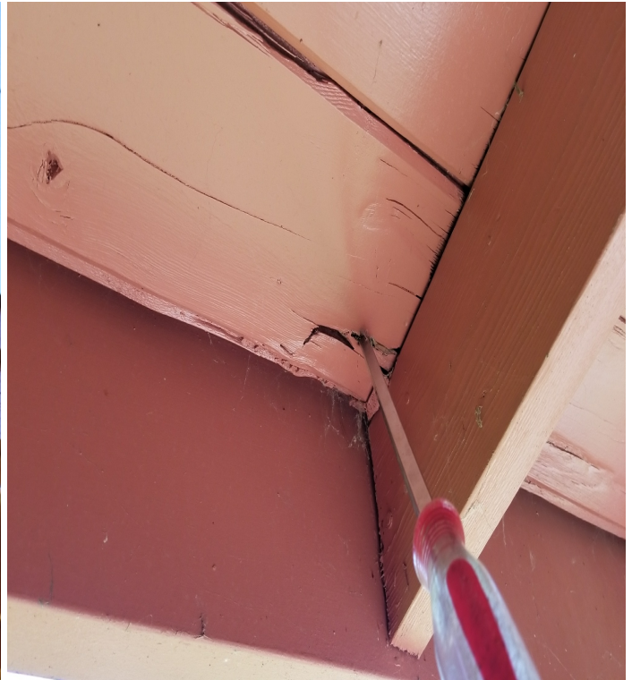
3 C - Damaged decking.
