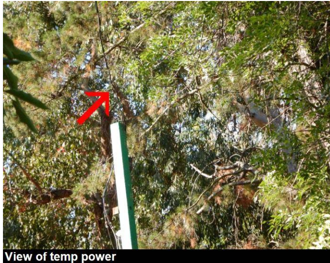
View of temp power
