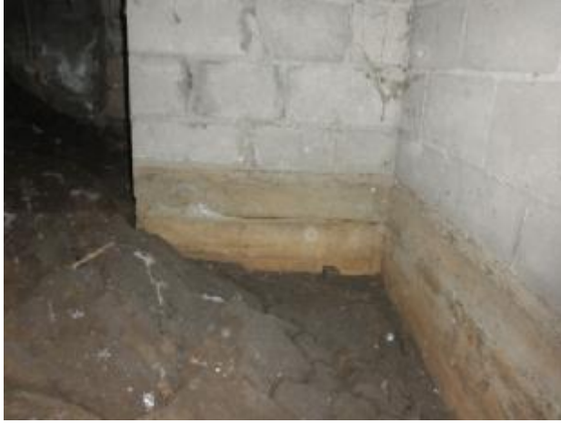
Evidence of past standing water in the substructure area to 12 inches deep.
