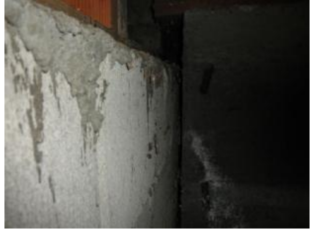
Gap between the concrete stem wall and the block stem wall at the NW corner of the substructure.
