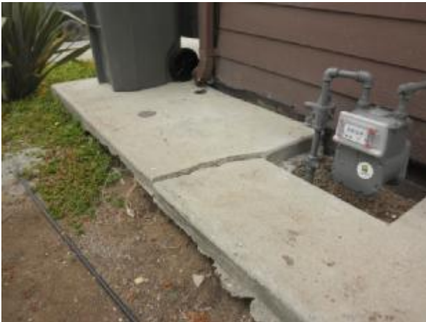
Settlement cracks with tripping hazards at the concrete walk along the south side of the home.
