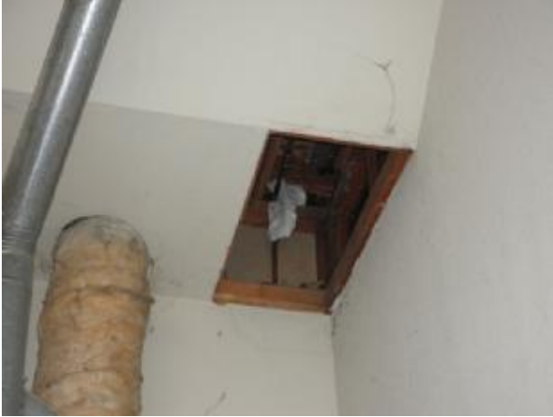
Hole cut through the ceiling in the garage compromises the integrity of the firewall.
