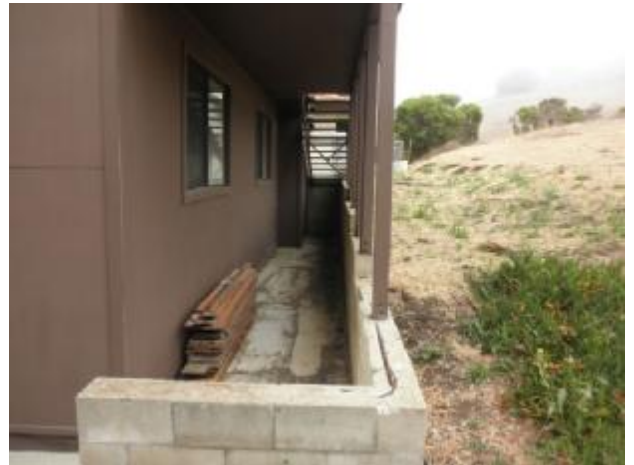
The CMU block retaining wall along the east side of the home is leaning.
