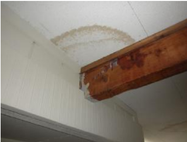
Evidence of roof leak in the upstairs NE bedroom addition.
