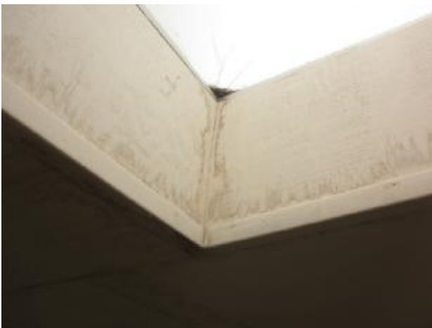
Evidence of leaks at the skylight above the enclosed deck.
