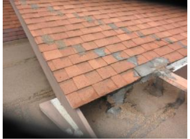
Amateur patching on the roof.
