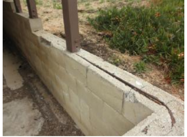
Damaged blocks and exposed rebar at the top of the CMU retaining wall.
