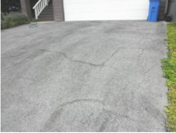
General deterioration and cracks in the asphalt driveway.
