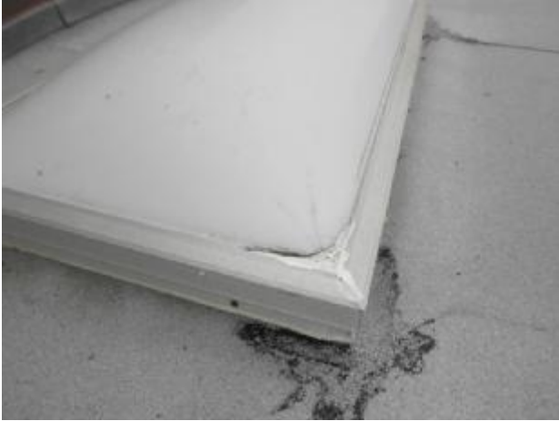
Cracks in the skylight dome.
