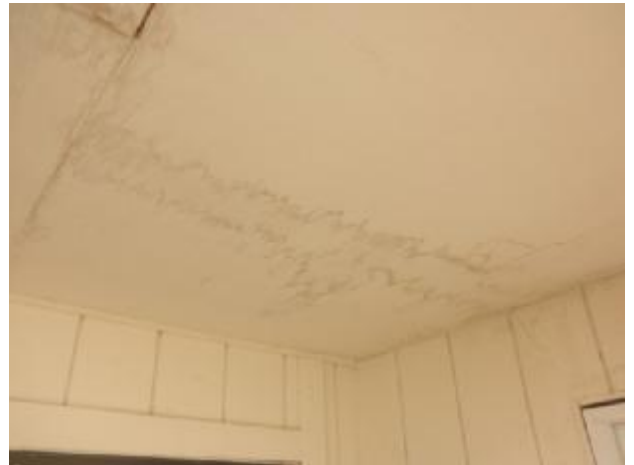
Evidence of roof leaks inside the enclosed deck.
