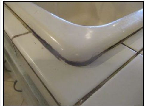
Gaps present between sink and countertop - potential for leakage - needs to be serviced
