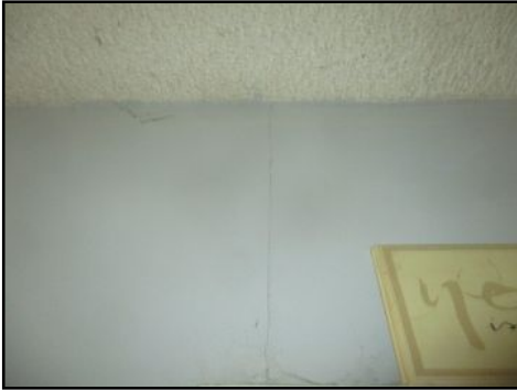
Large cracking present – larger than typical - needs to be further evaluated/serviced
