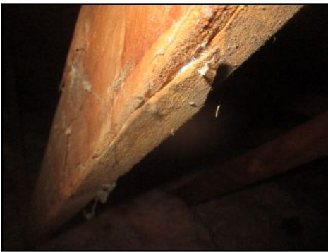
Cracked wood/rafters- needs to be serviced
