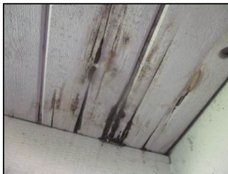
Evidence of patio roof leaking - stained/moisture damaged/fungus present at under side - needs to be serviced
