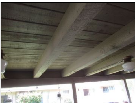
General view - underside
