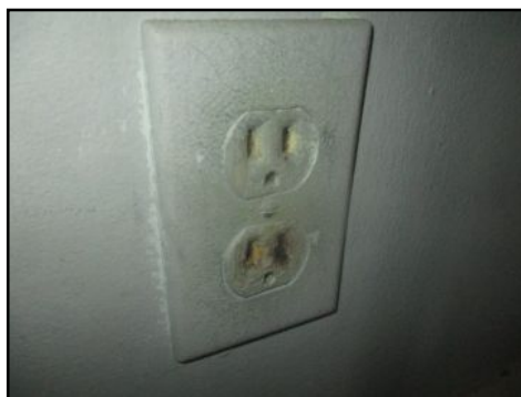
Burnt outlet - needs to be serviced/evaluated - at master bedroom
