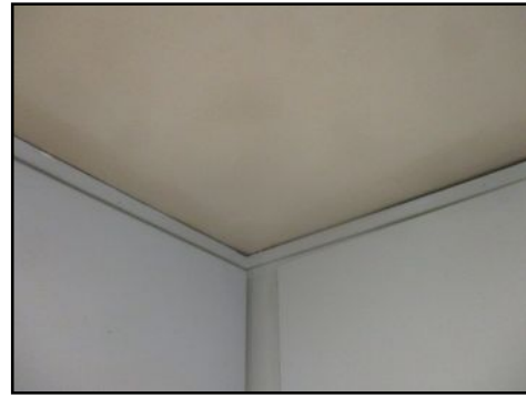
Cabinets gapped at ceiling
