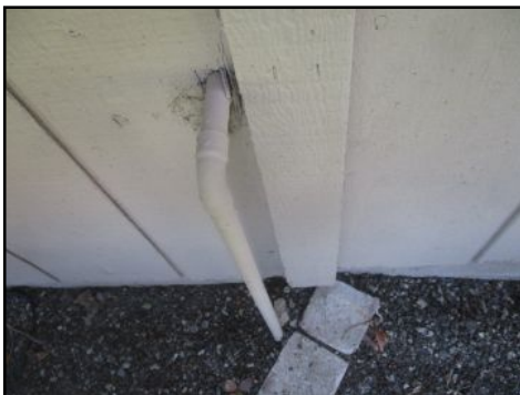
Exterior plumbing is present and not original to the structure - check all installation permits to ensure installation to building code
