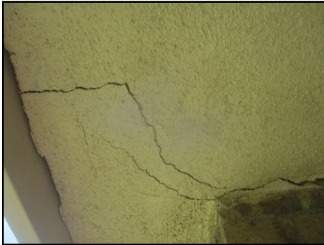
Large cracking at soffit area(s) by chimney - needs to be serviced
