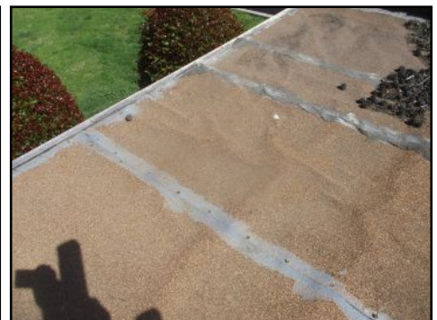
Wrinkled/worn/weathered rolled materials
