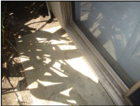
Exterior door landing/pad slopes toward structure
