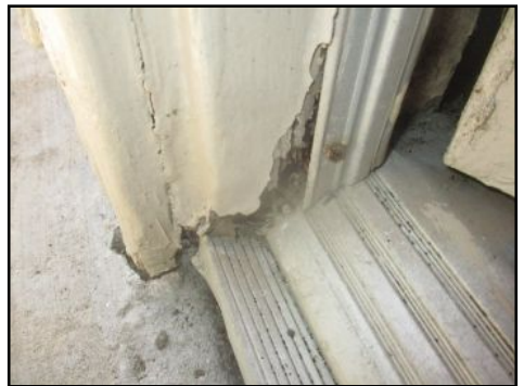
Damaged jamb/trim - needs to be serviced - consult termite report
