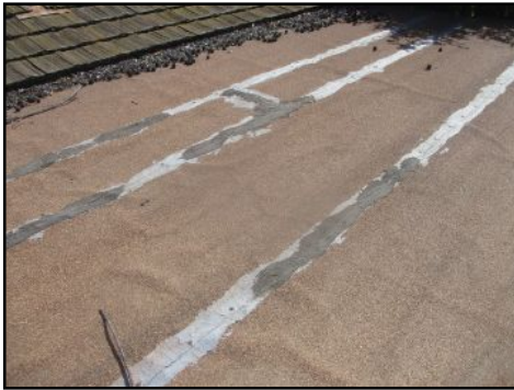
Improper installation of rolled materials/fasteners/flashing(s)
