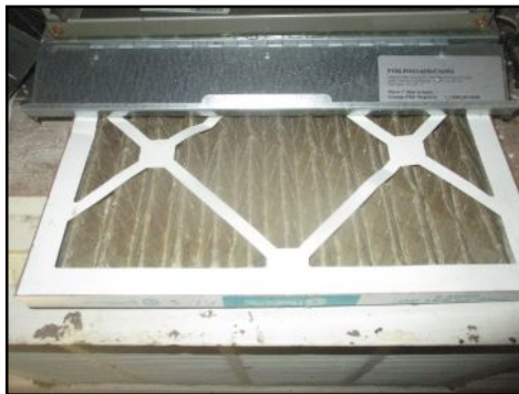
Filter is worn/dirty - needs replacement
