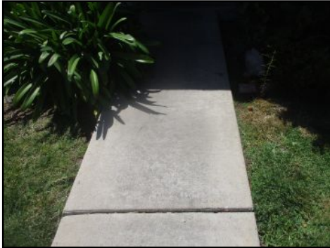
Walkway/concrete displacement/uneven areas - needs to be serviced
