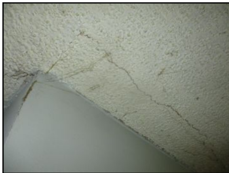
Large cracking present – larger than typical - needs to be further evaluated/serviced
