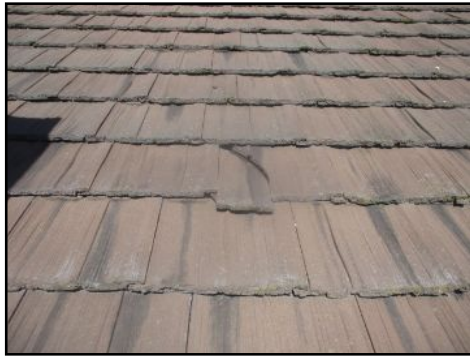
Cracked/broken/loose tiles in areas - needs to be serviced
