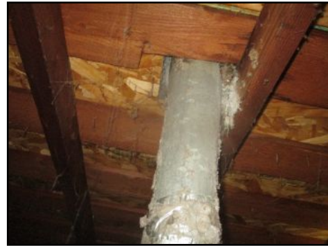
Dryer vent appears to need cleaning/serviced - dryer lint escaping vent in attic - needs to be serviced
