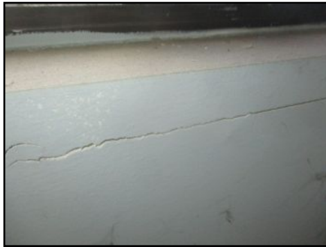
Large cracking present – larger than typical - needs to be further evaluated/serviced
