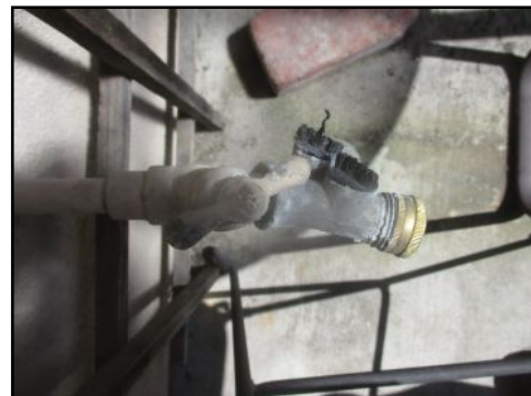
Capped at exterior hose bibb - could not test - N/A
