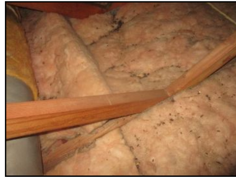
Evidence of rodent/bird/pest activity in the attic - recommend further evaluation by pest services company
