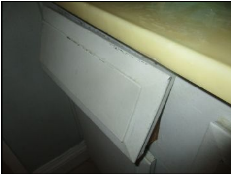
Broken drawer(s)/hardware
