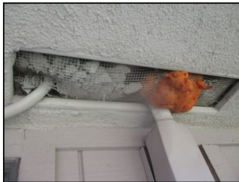
Torn mesh/screens - needs to be serviced to prevent pest entry
