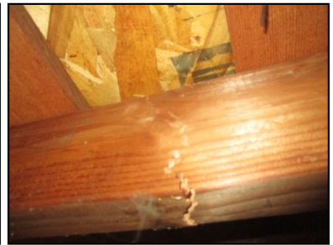
Cracked wood/rafters- needs to be serviced
