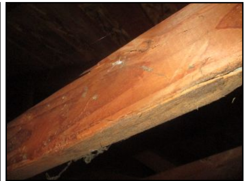
Cracked wood/rafters- needs to be serviced
