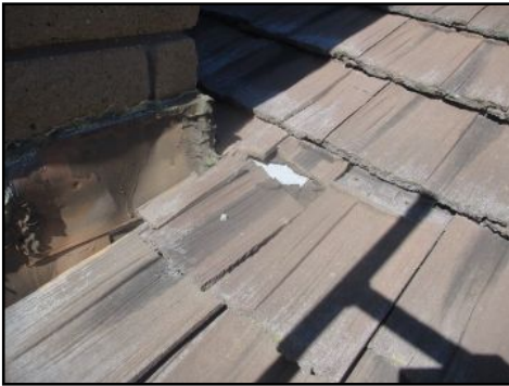
Cracked/broken/loose tiles in areas - needs to be serviced
