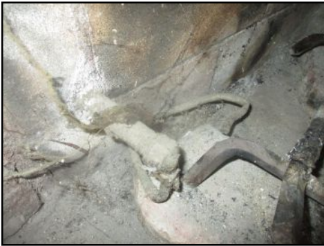
Gas log lighter/connector damaged/cut - needs to be serviced
