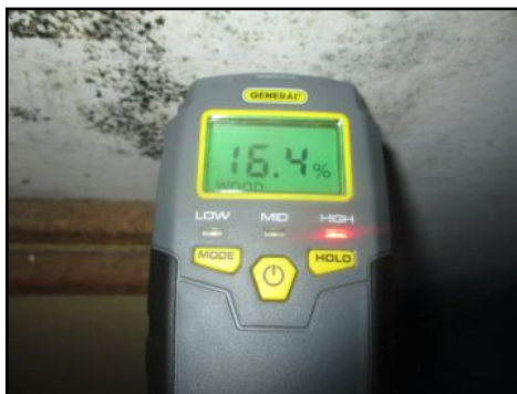
Moisture damaged/blistered area(s) - moisture present at time of inspection - evidence of past moisture intrusion and/or roof leaking - needs to be serviced
