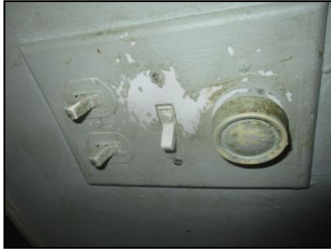
Loose/worn outlets/switches - typical for age consider upgrading
