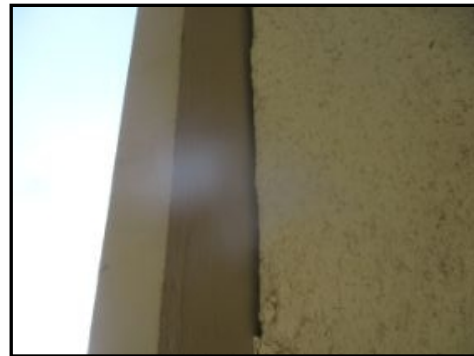
Small gaps at wood trim/stucco junctures - needs to be sealed to prevent pest intrusion
