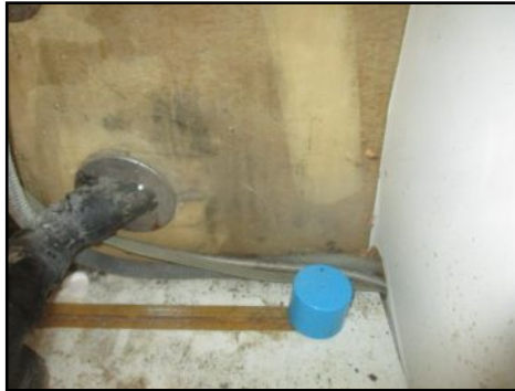
Microbial growth/irregular staining present - further evaluation is recommended
