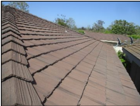
Cracked/broken/loose tiles in areas - needs to be serviced
