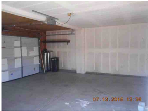
Interior of the garage
