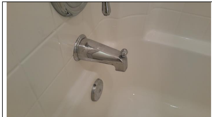
Diverter not operate properly during shower cycle
