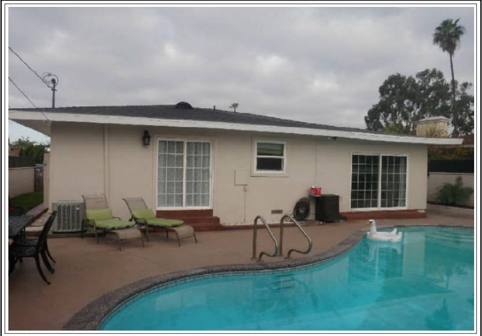
REAR VIEW OF SUBJECT PROPERTY
