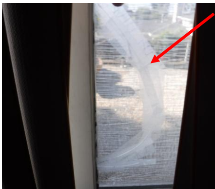
The master bedroom has a cracked window pane
