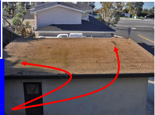
The garage rock roof has bare areas as well
