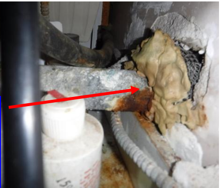
The kitchen sink waste pipe is prone to leaks
