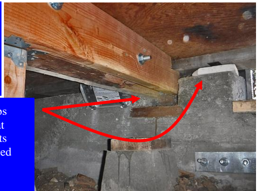
The kitchen floor assembly was lifted, leveled and re-supported...
