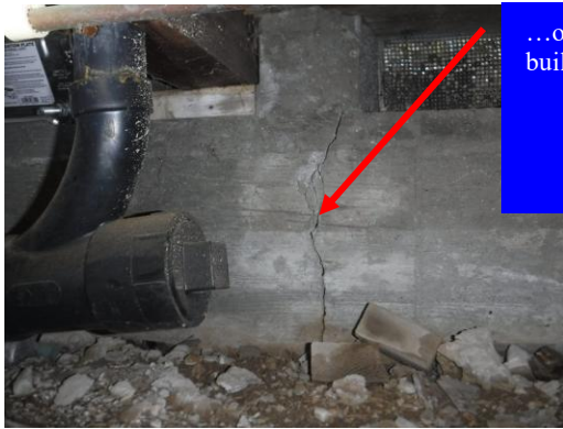
...when these cracks appear to be candidates for epoxy filler...
