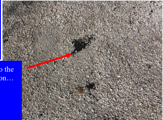
The home's rock roof has a number of bare areas...
