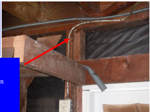
...is provided power with indoor strand wiring routed outdoors...
