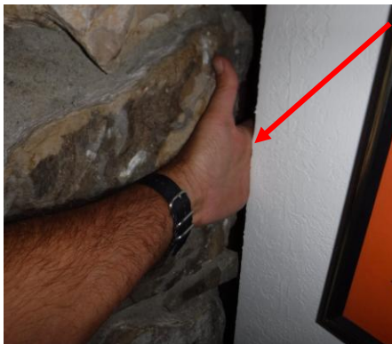
...and the chimney has settled resulting in a large opening where abutting the W-wall...
