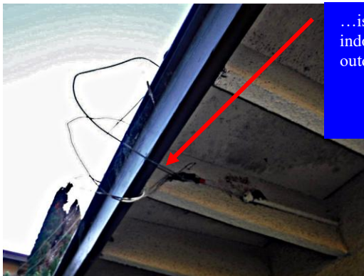
...as well as having exposed cloth-wrapped distribution cable within the garage
