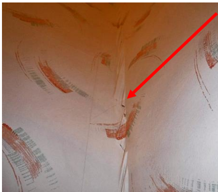
...of which some are masked by wall paper where rippled finishes reveal the off-sets...
