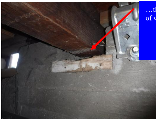
...and replacement of plastic shims...
