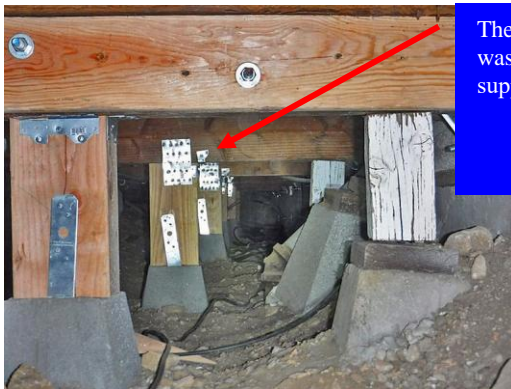
...resulting is large gaps where girders now float above their wall pockets and the sill plate is raised above the foundation wall...
