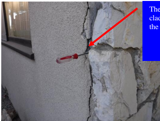
Many areas of the home's perimeter have patched areas at the foundation where blistered finishes and re-occurring cracks have emerged...
