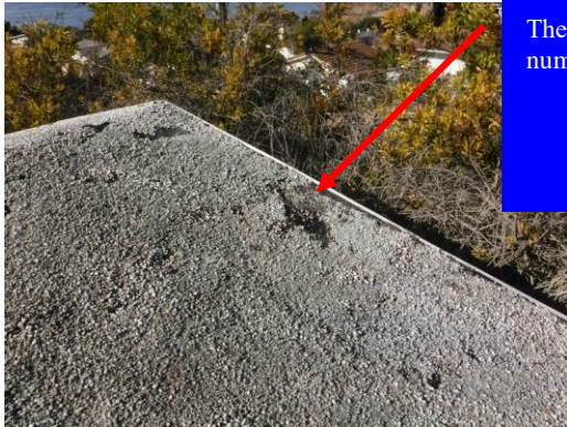
...where UV damage to the system requires attention...
