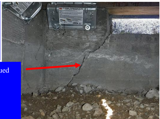
...at the numerous foundation wall cracks that have been left untouched...
