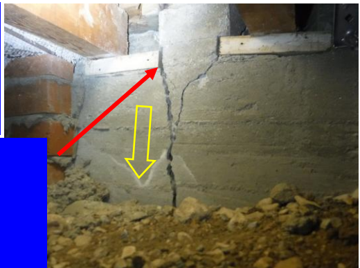
...and the chimney has settled resulting in a large opening where abutting the W-wall...
