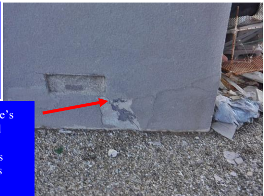
The N-exterior wall's stone cladding has detached from the structure
