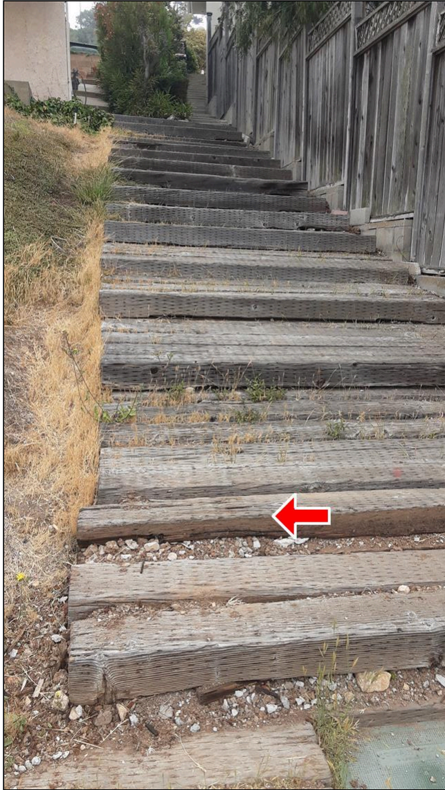
1.6 Item 1(Picture) Steps leading to west side
