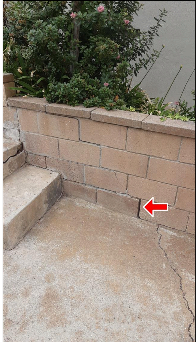
1.9 Item 2(Picture) Retaining wall
