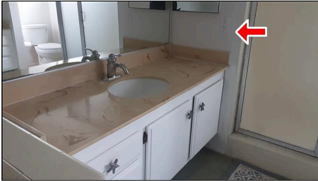
5.5 Item 6(Picture) Master bath outlet
