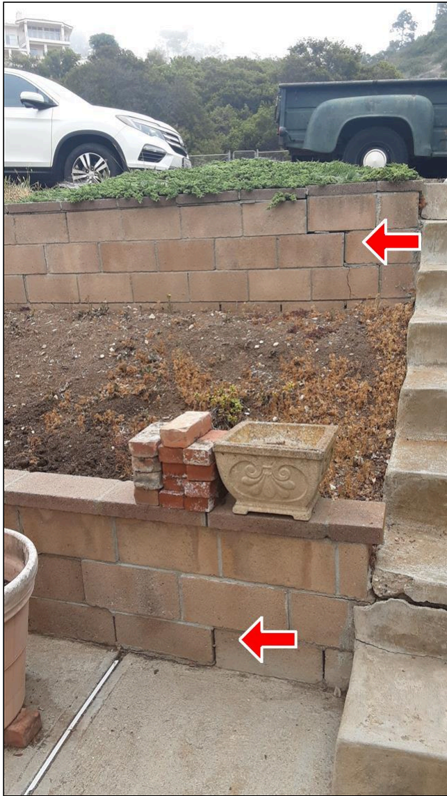
1.9 Item 1(Picture) Retaining walls
