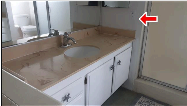
5.5 Item 6(Picture) Master bath outlet
