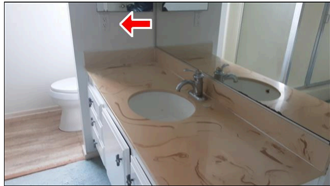
5.5 Item 5(Picture) Master bath outlet
