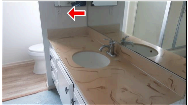
5.5 Item 5(Picture) Master bath outlet
