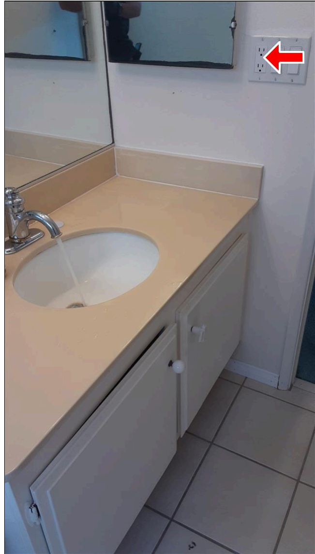
5.5 Item 7(Picture) hall bathroom outlet
