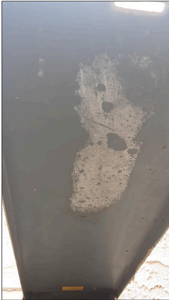
5.2 Item 1(Picture) Missing panel information
