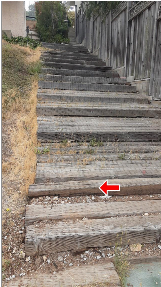
1.6 Item 1(Picture) Steps leading to west side
