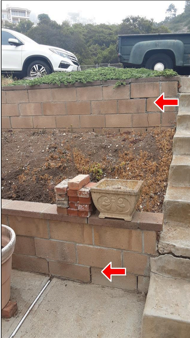
1.9 Item 1(Picture) Retaining walls
