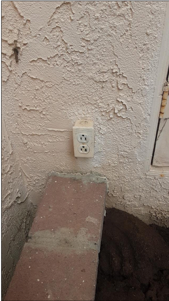
5.5 Item 2(Picture) Exterior outlet, front patio
