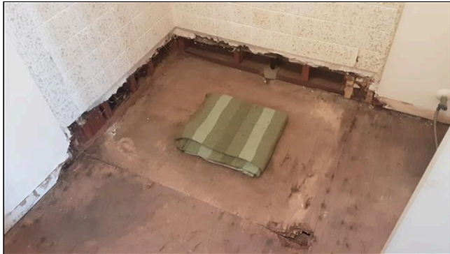
6.4 Item 1(Picture) Removed shower pan, lower level hall bathroom
