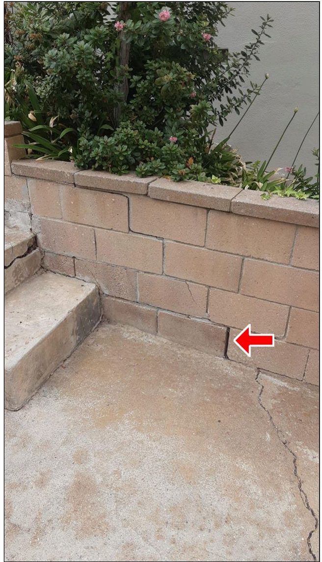
1.9 Item 2(Picture) Retaining wall
