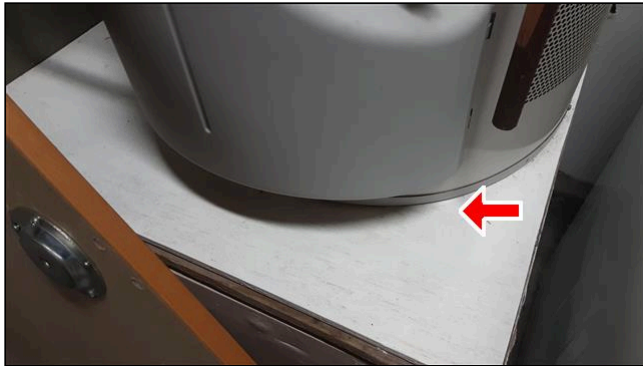
6.2 Item 4(Picture) Missing drip pan
