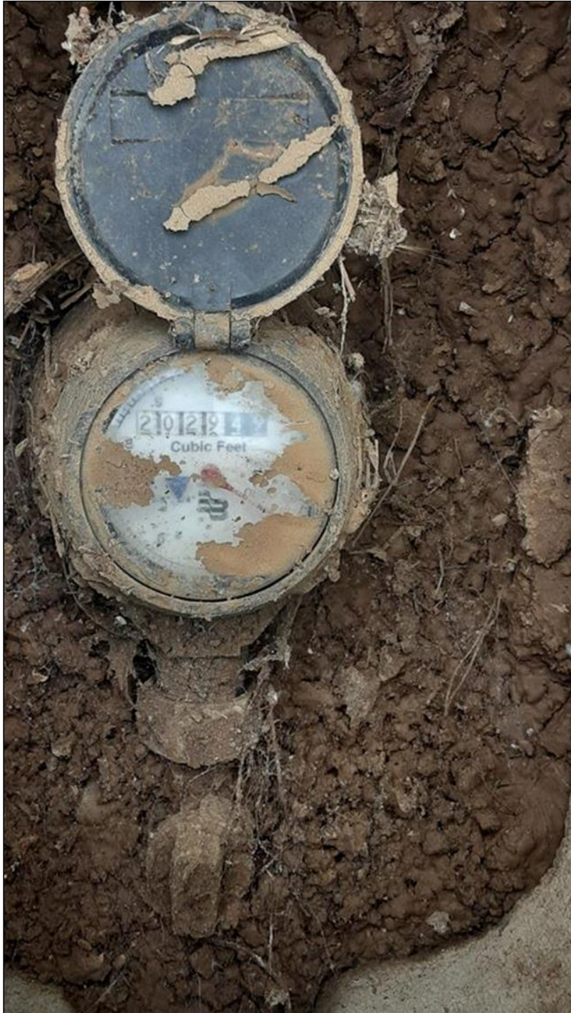
6.0 Item 1(Picture) Water meter
