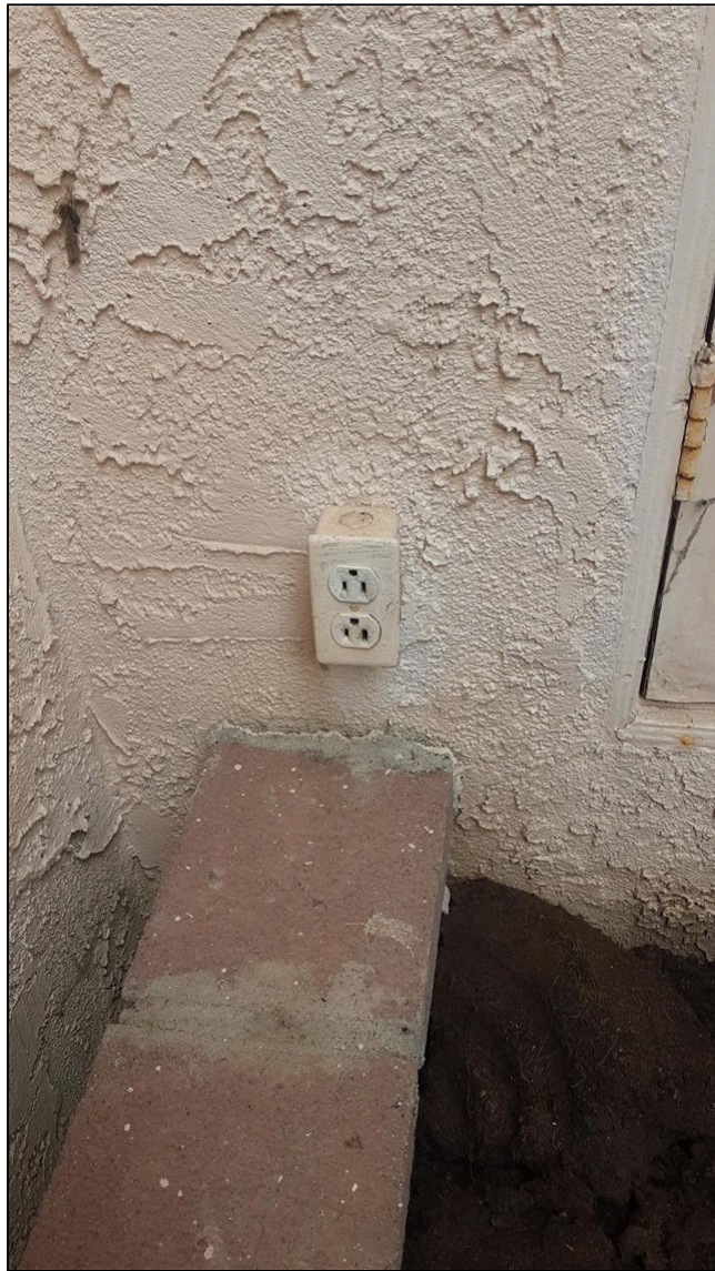
5.5 Item 2(Picture) Exterior outlet, front patio
