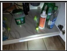
There is ponding water on the base of the cabinet under the sink. No moisture to the walls.
