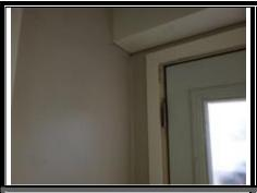
There is patchwork, nails popping, and ripping to visible seams throughout the home. No signs of damage or moisture to these areas today. Image of the laundry room seam between the south and west walls.
