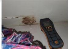
elevated moisture on the north built-in cabinet. This cabinet and wall back up to the hallway bathroom tub.
