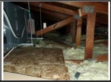
There is insulation present in the attic space. The insulation is covering the backside of the ceiling throughout the home.
