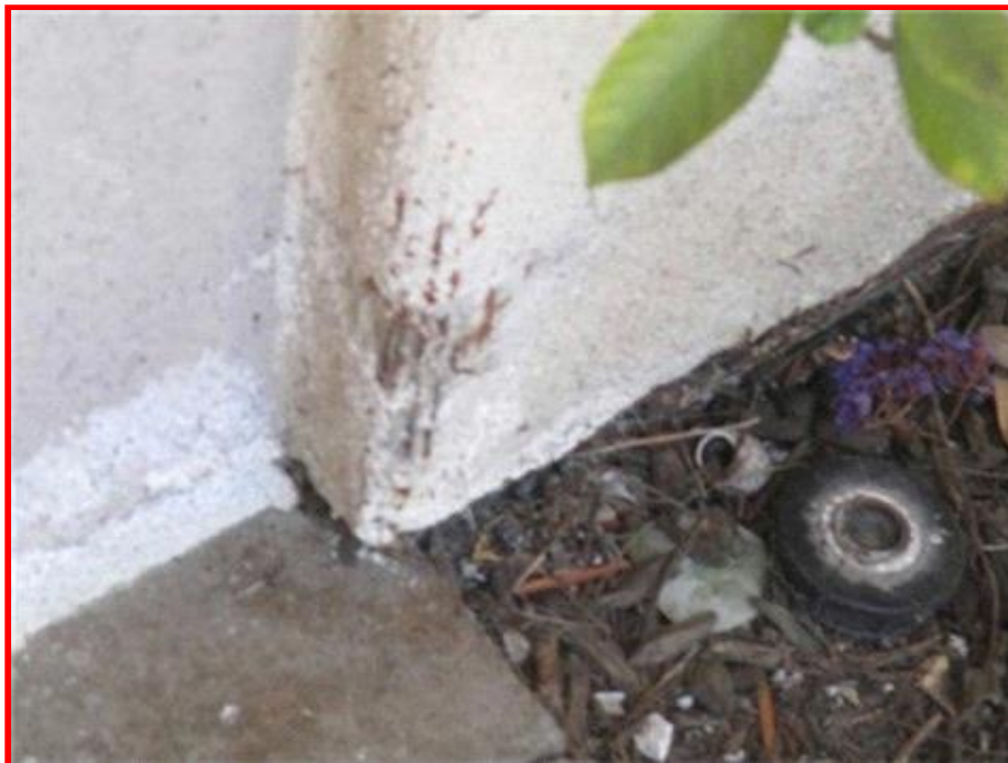
Exposed Corner / Damage at Rear Door
