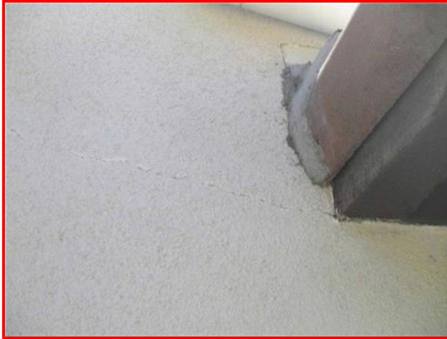
Cracks in Stucco at Front
