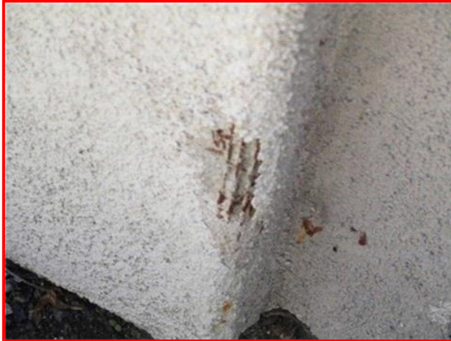
Exposed Corner / Damage at Atrium
