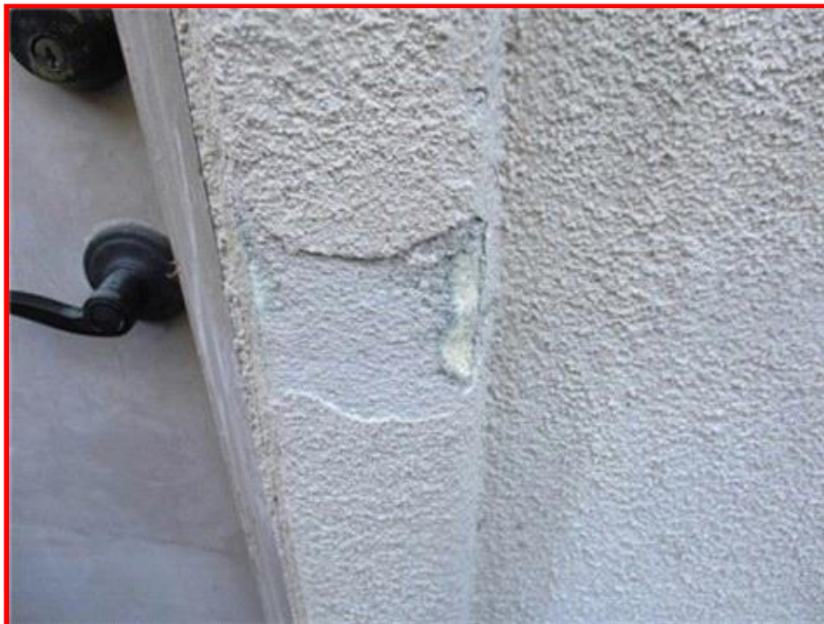
Damaged Garage Door Trim
