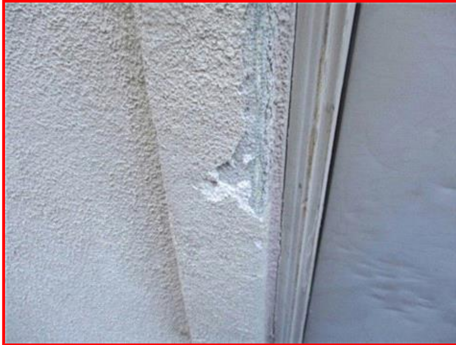
Damaged Garage Door Trim
