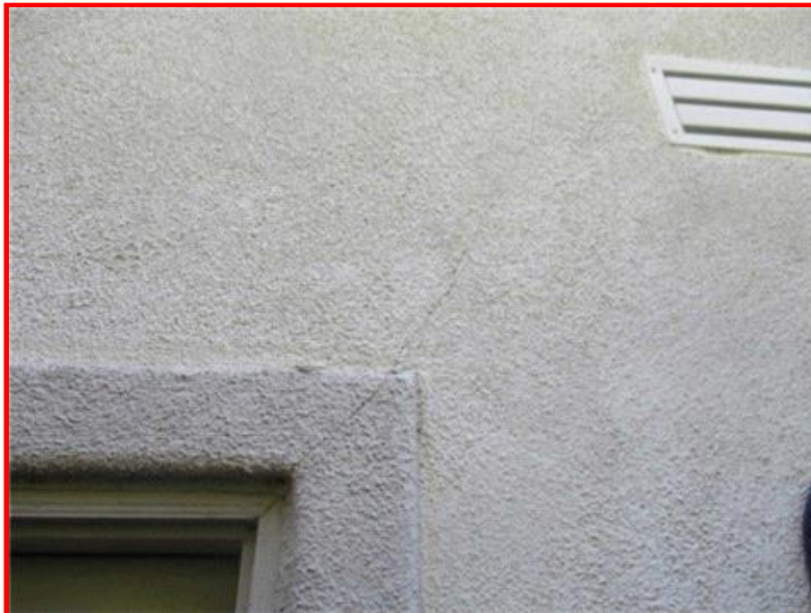
Cracks in Stucco at Garage
