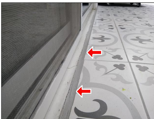
4.4 Item 2(Picture) Area of drainage concern. Negative slope noted by patio sliding doors
