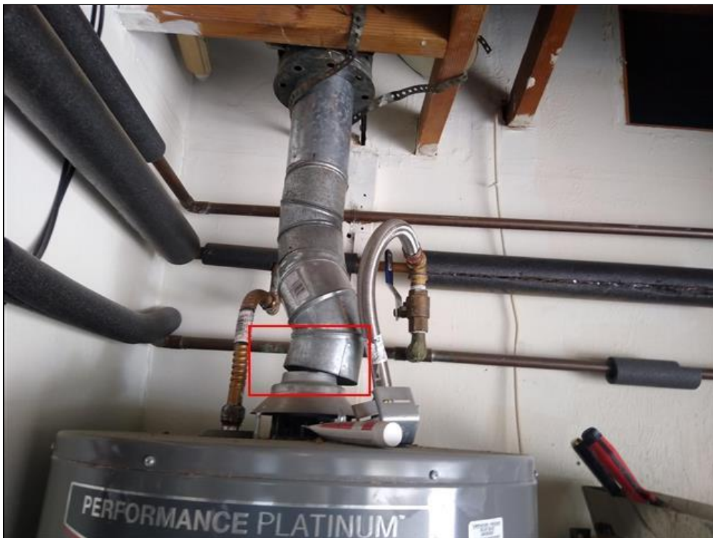
6.7.A Item 1(Picture) No screws noted and gaps observable, which are a safety concern
