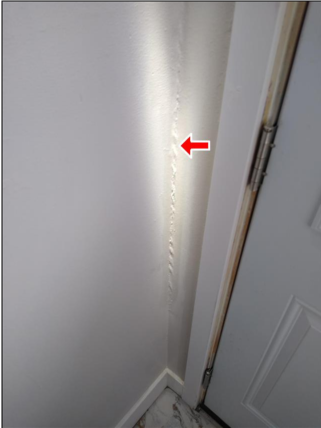
4.0 Item 1(Picture) Blistering noted at corner near laundry area. Ask seller for history.
