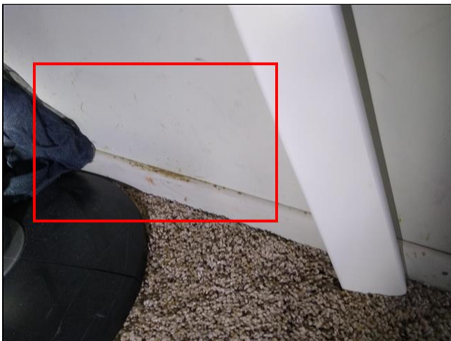
4.0 Item 7(Picture) SE front bedroom - Area of concern - Discoloration, possible mold growth noted.
