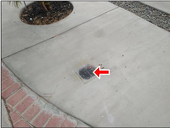
2.4 Item 1(Picture) Subsurface drainage noted.
