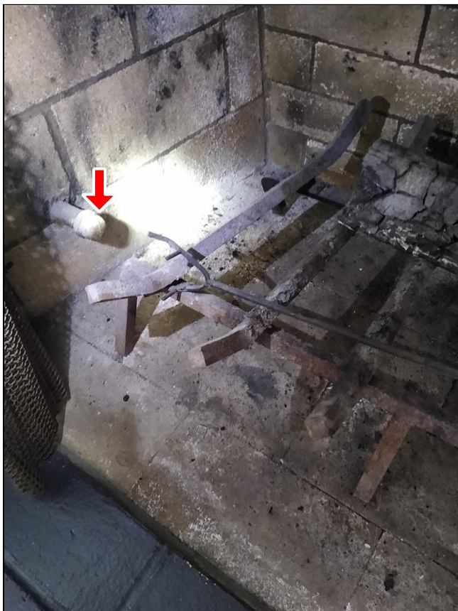
4.6 Item 1(Picture) Gas piping was capped
