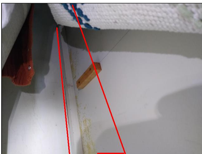
4.0 Item 10(Picture) SE front bedroom - Area of concern - Discoloration, possible mold growth noted.
