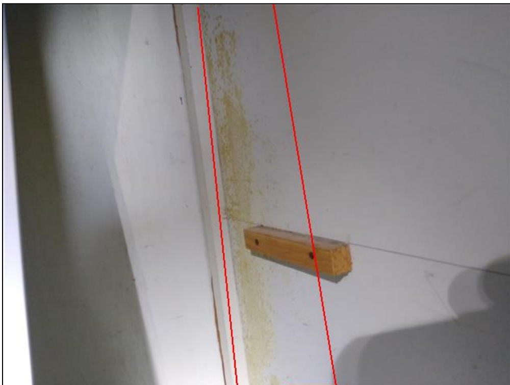
4.0 Item 9(Picture) SE front bedroom - Area of concern - Discoloration, possible mold growth noted.
