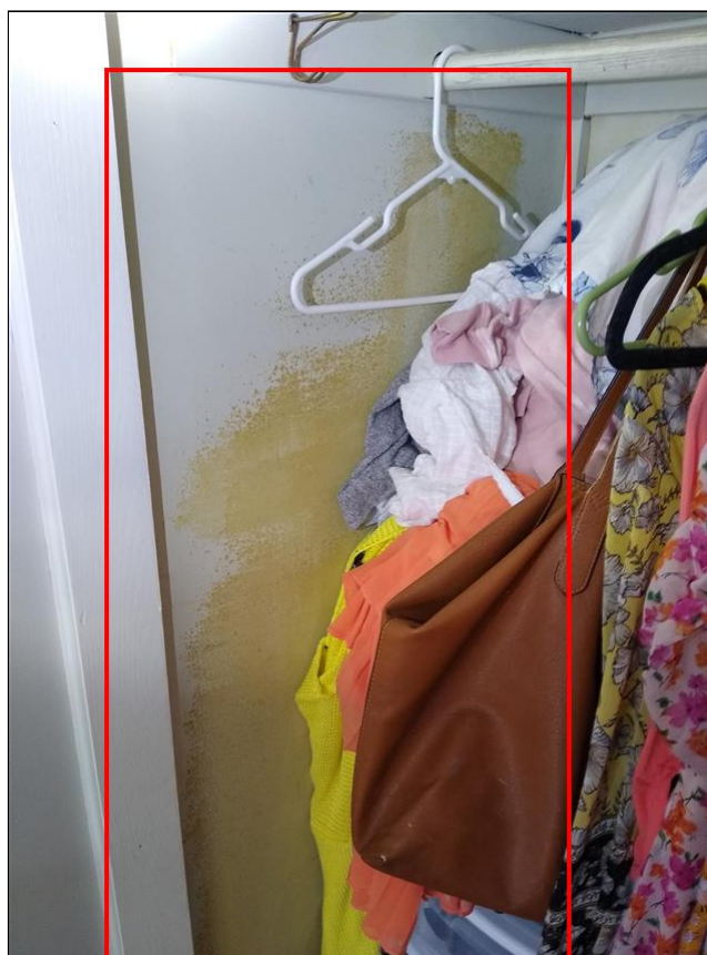
4.0 Item 11(Picture) NE rear bedroom (Master) - Area of concern - Discoloration, possible mold growth noted.
