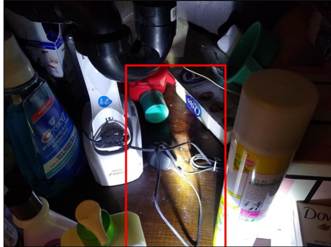
6.0.B Item 2(Picture) Staining/moisture damage noted
