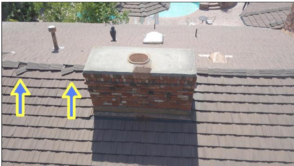
7.0 Item 3(Picture) There are several roof tiles that are loose and should be serviced.
