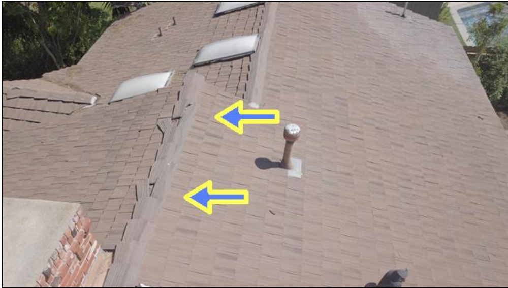
7.0 Item 1(Picture) There are several roof tiles that are loose and should be serviced.
