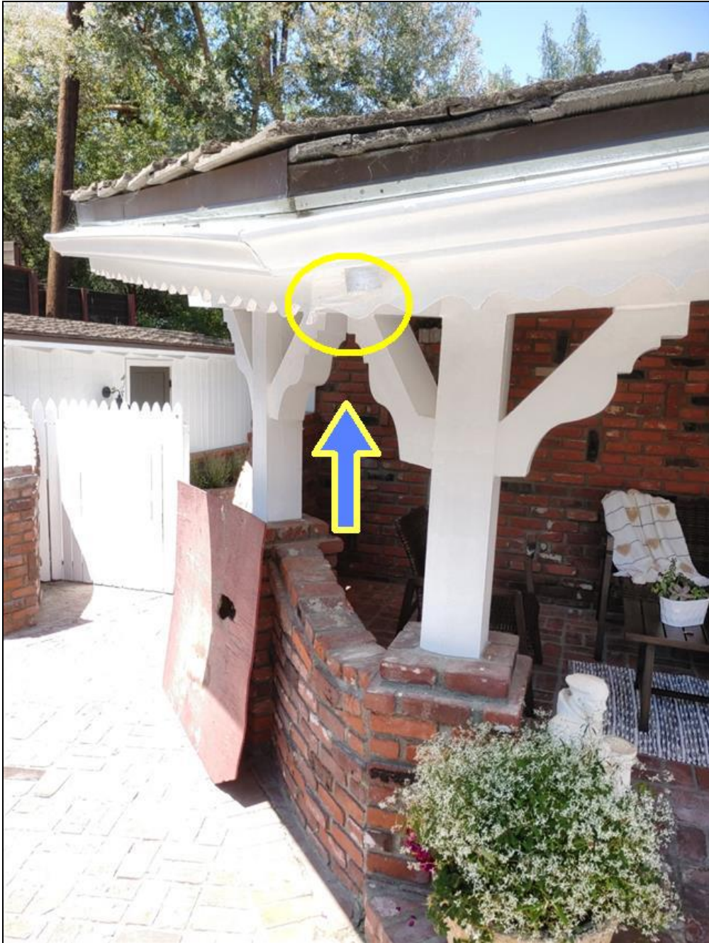
2.3 Item 1(Picture) The rain gutter at the rear of the house is missing a downspout. We recommend further evaluation and services necessary.
