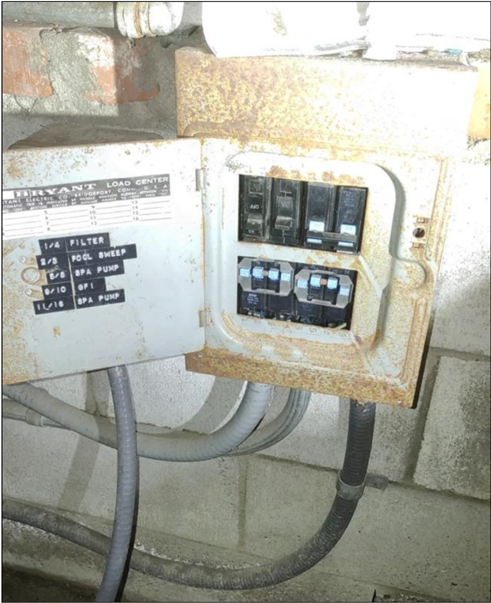
6.2 Item 1(Picture) sub panel in pool equipment room.
