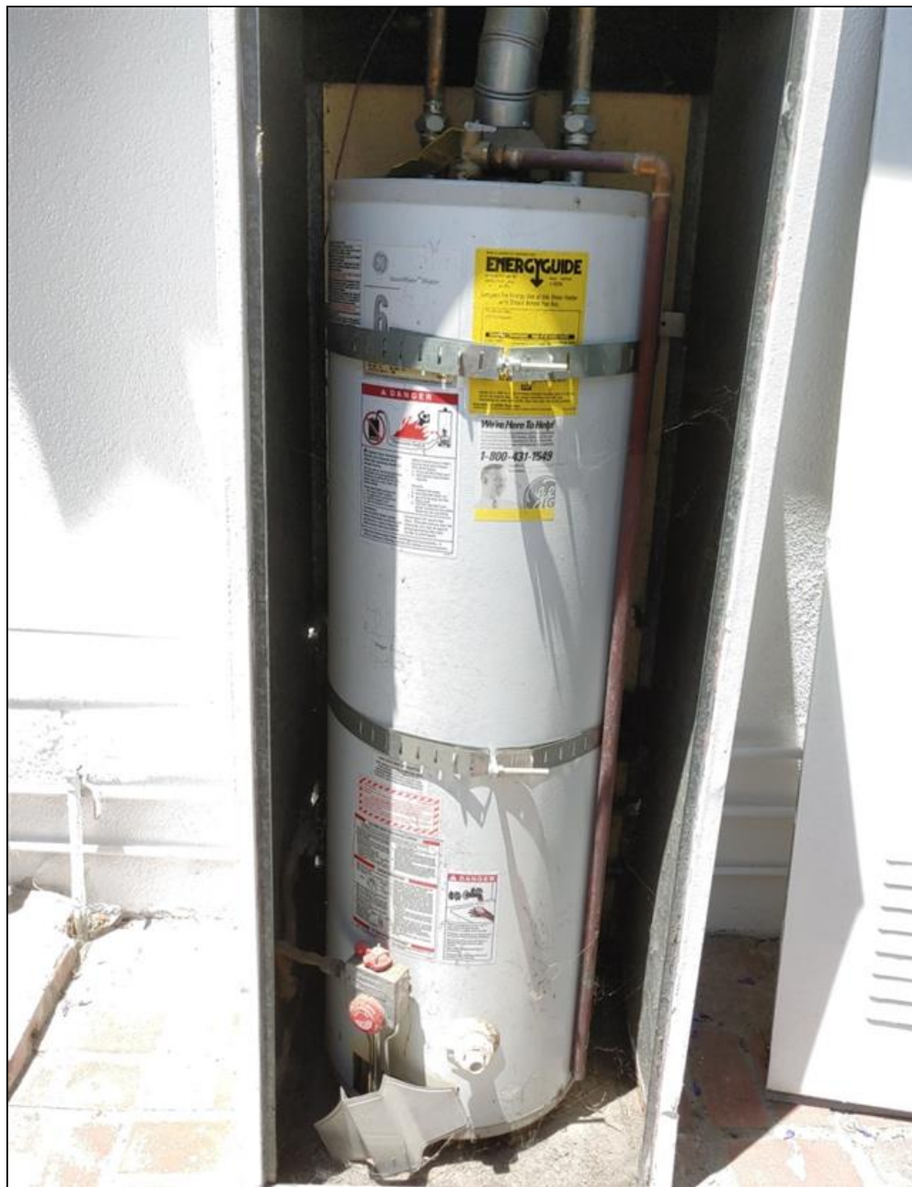
5.2 Item 1(Picture) The water heater in the exterior closet is 16 years old in 40 gallons.
