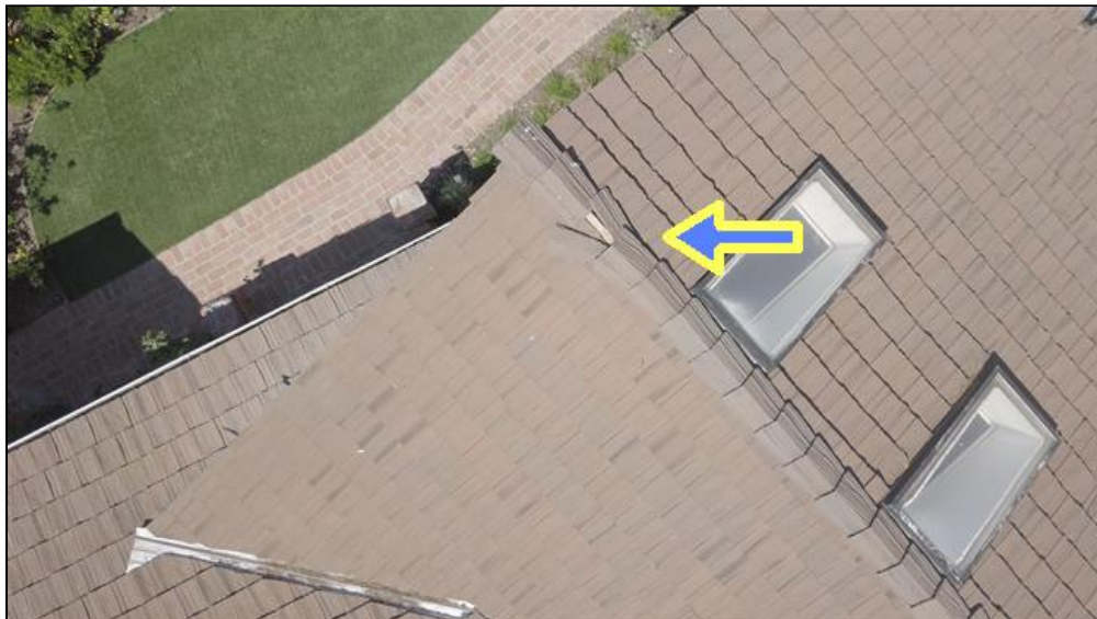
7.0 Item 2(Picture) There are several roof tiles that are loose and should be serviced.
