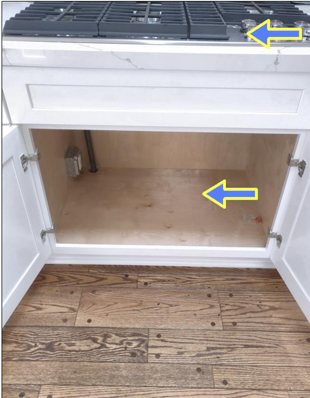
11.9 Item 1(Picture) The cooktop was not fully installed. The down-draft was missing too.
