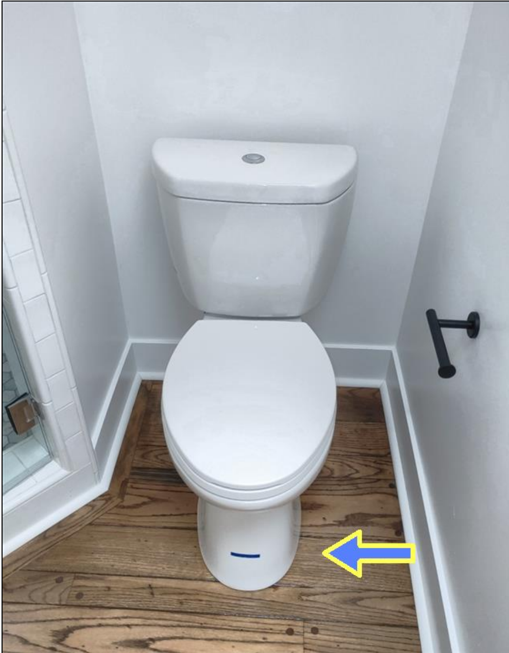
15.6.B Item 1(Picture) The hallway bathroom toilet is loose and should be serviced.
