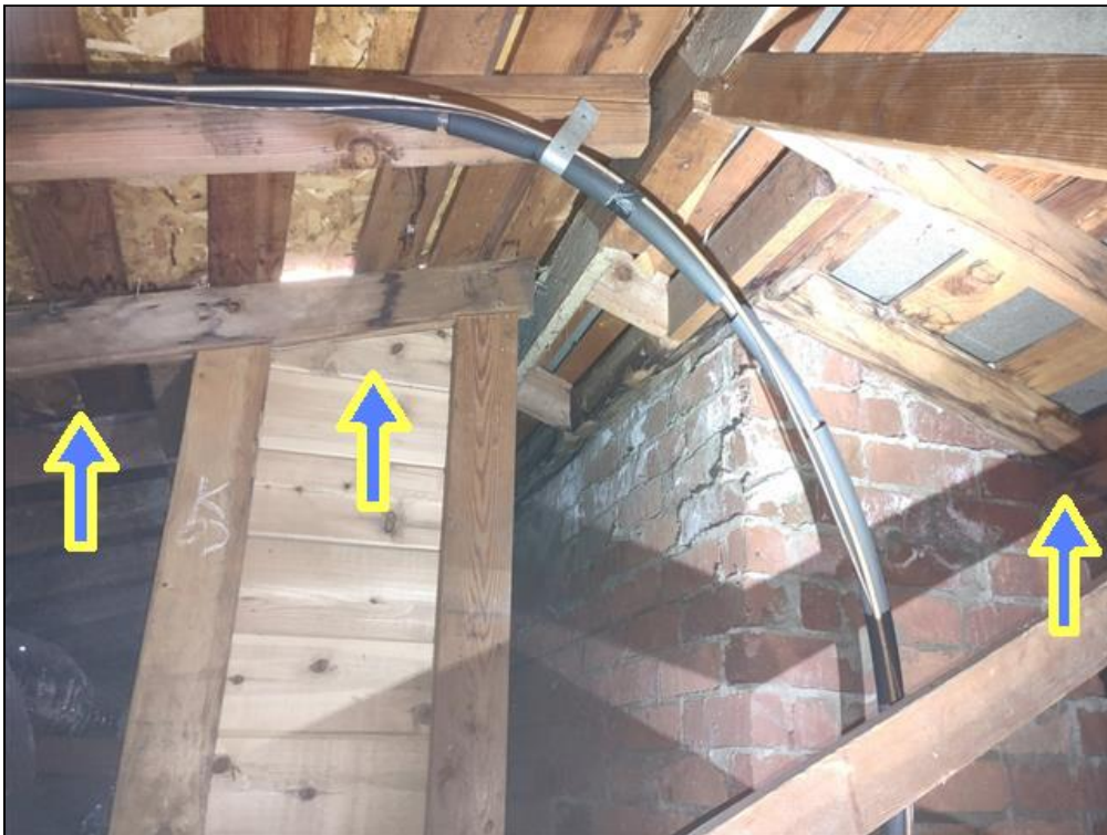
7.5 Item 1(Picture) There are several areas in the Attic that have moisture stains. We are unable to confirm these as active. We recommend further evaluation and service as necessary.
