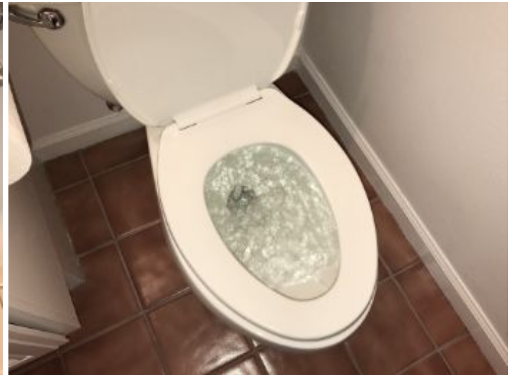
Appeared functional, at time of inspection.
