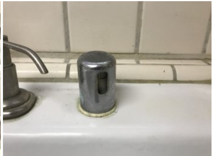
Air gap present and functional.
