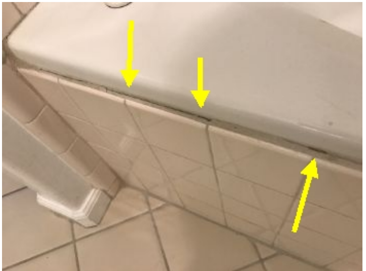
Recommend caulking around the perimeter.
