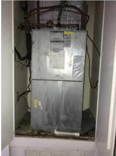
The Heater enclosure is functional.
