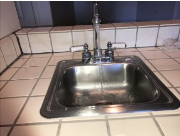
The bar sink appeared functional at time of inspection
