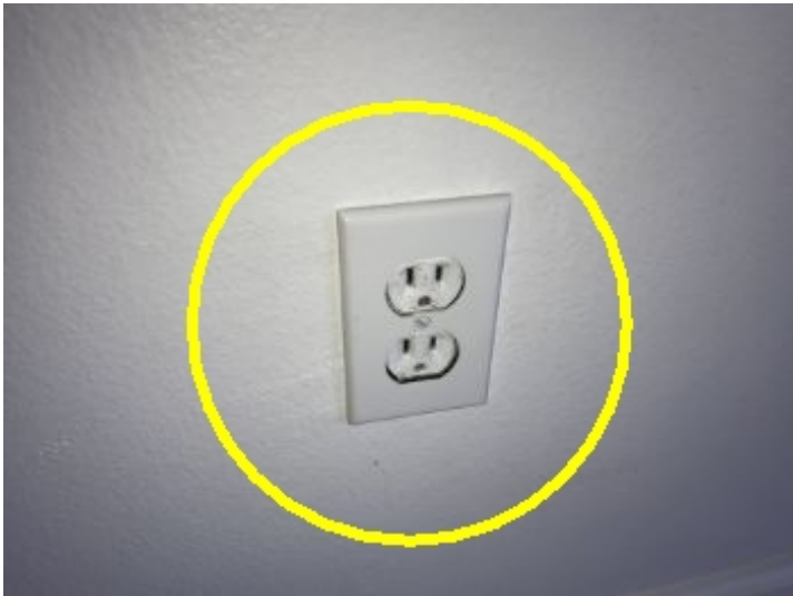
Damaged outlet observed. Suggest replacing as necessary. See photo
