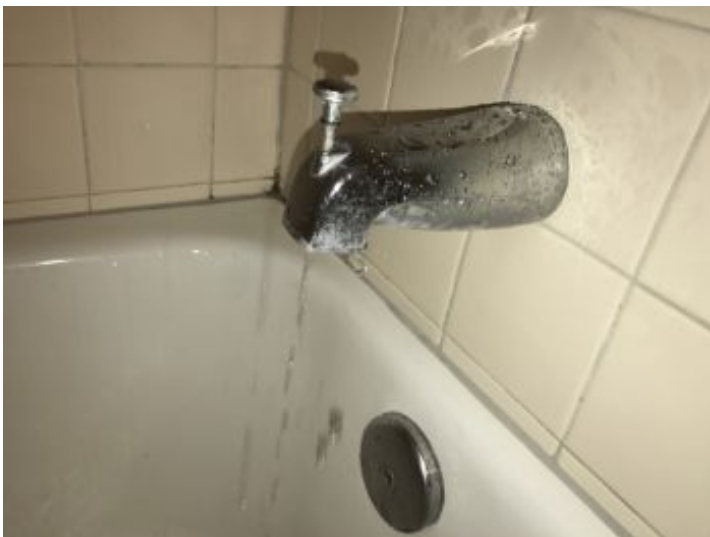
Shower diverter does not fully engage.
