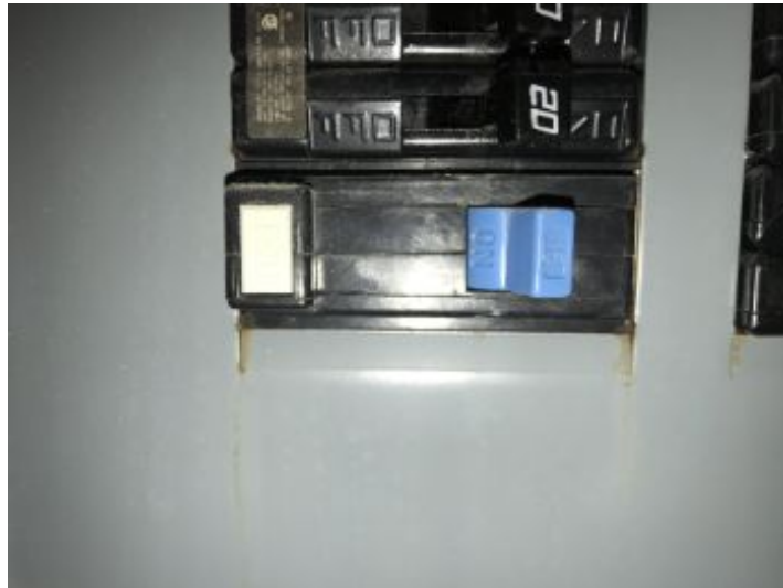
AFCI breakers installed and tested functional
