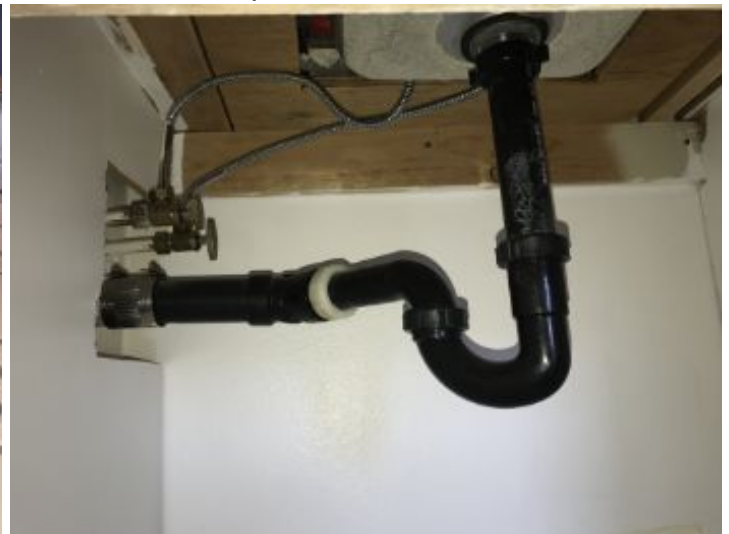
New plumbing hardware at drains noted
