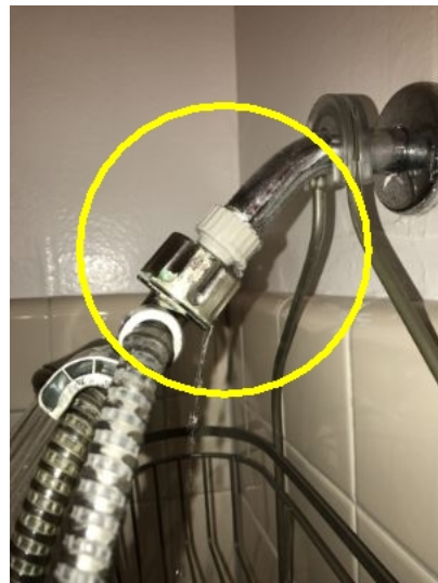
Shower head leaks.
