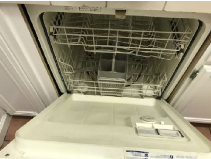
Appeared functional and in satisfactory condition, at time of inspection.
