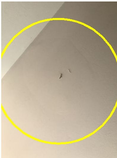
The drywall is patched in areas. The reason for the patch could not be determined.
