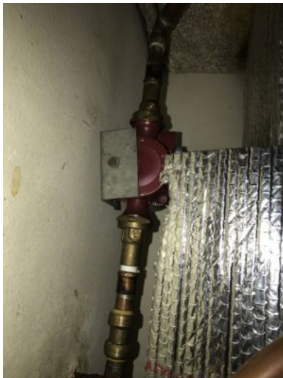
Recirculating Pump noted
