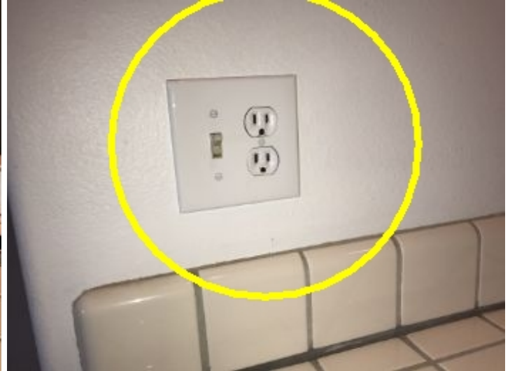
There is a non GFCI protected outlet next to the bar sink. Recommend installation of a GFCI protected outlet.
