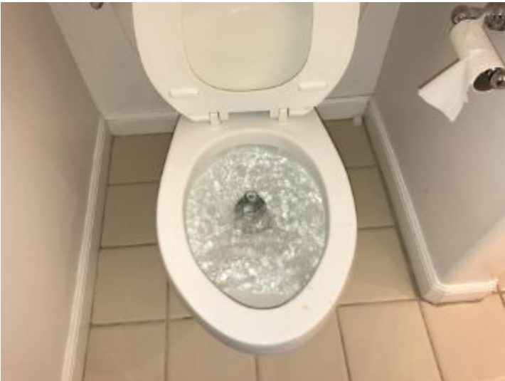
Appeared functional, at time of inspection.
