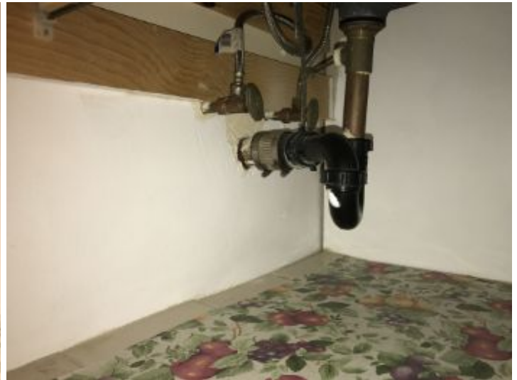
Appeared functional, at time of inspection. Drains were tested, no leaking and no indication of stoppages at time of inspection.
