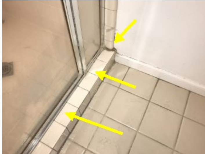
Caulking needed around perimeter.
