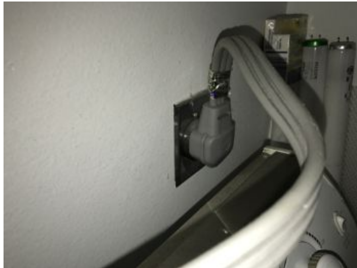
Appeared functional, at time of inspection.
