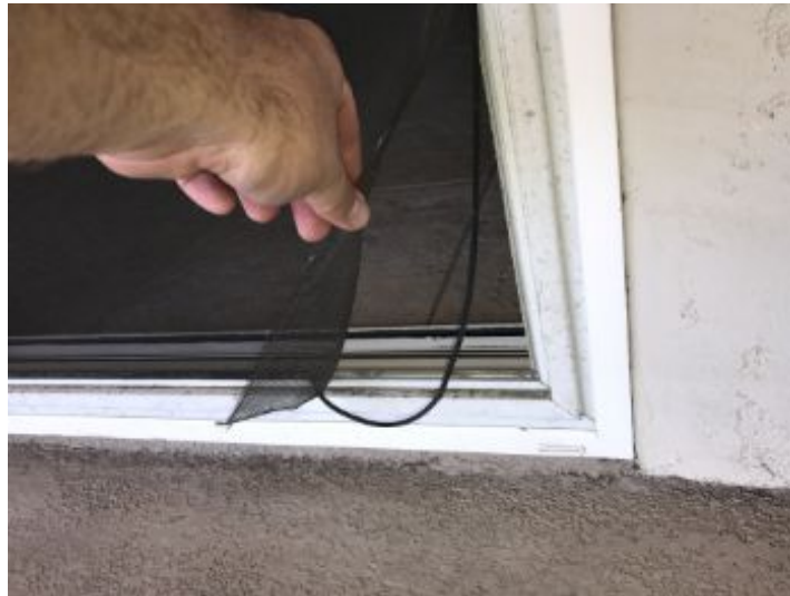
Sliding door screen is damaged
