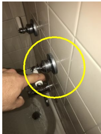
Faucet is not flush to the wall, which may result in water penetration to the interior structure and deterioration of the wall.
