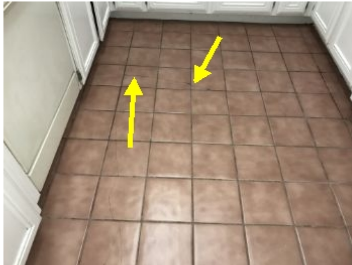
Common cracks noted.
