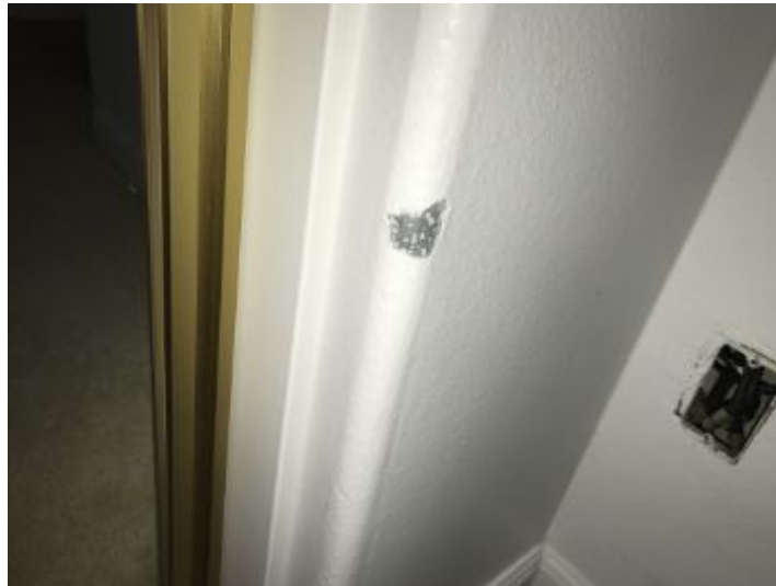
Minor drywall damage noted.
