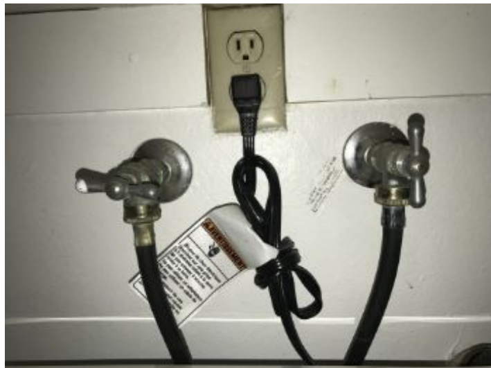
Due to the washer connected at plumbing fixtures, inspector could not properly test plumbing at time of inspection. N/A
