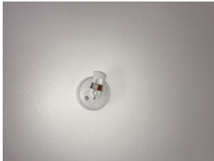
Replace all old not functioning smoke/ fire detectors with new hard wired detectors or make sure batteries are good.
