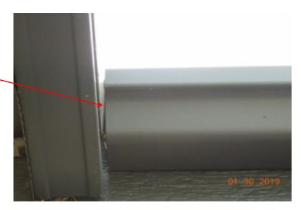
(Missing Pieces) Missing pieces were noted on the gutter. (Endcap / Drain spout)
