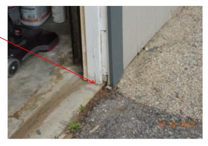
(Bottom Seal Missing / Damaged) The Garage door bottom seal was noticed as missing / damaged.
