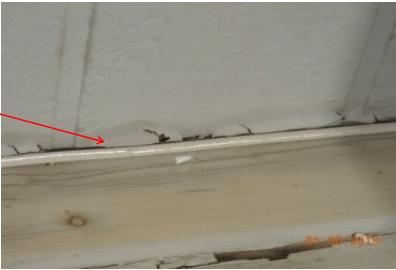
(Holes) Holes should be repaired or sealed to prevent water damage.
