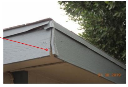
(Loose Boards) The Fascia / Eaves boards appear to be loose and should be secured.
