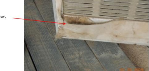
$\label{thm:continuous} \textbf{Suggest securing insulation onto door.}$
