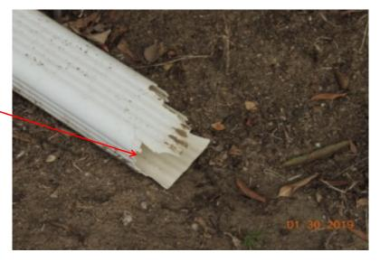
(Gutter Damage / Bent) The gutters were noted as being damaged, which could result in them not working as intended.
