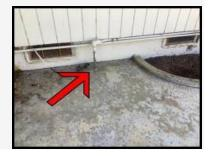
• Exposed conduit subject to damage is visible across the rear porch step. We recommend correction using appropriate methods.
