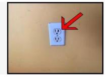
Crack damage is visible to receptacles at the family room. The condition poses an
