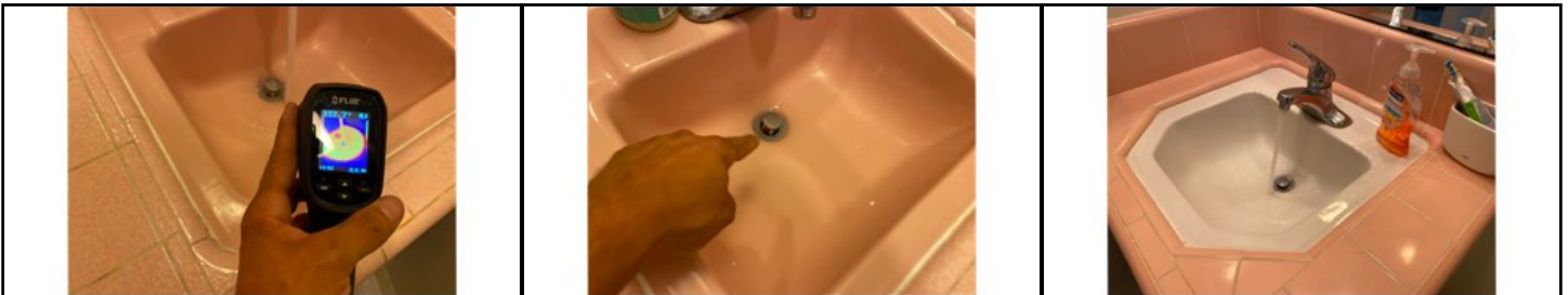
Drain stopper not operating properly - needs to be serviced
