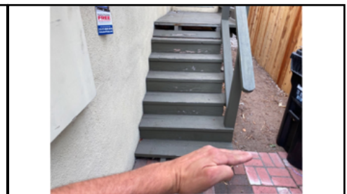
Damaged steps - unsafe - needs to be serviced- not level
