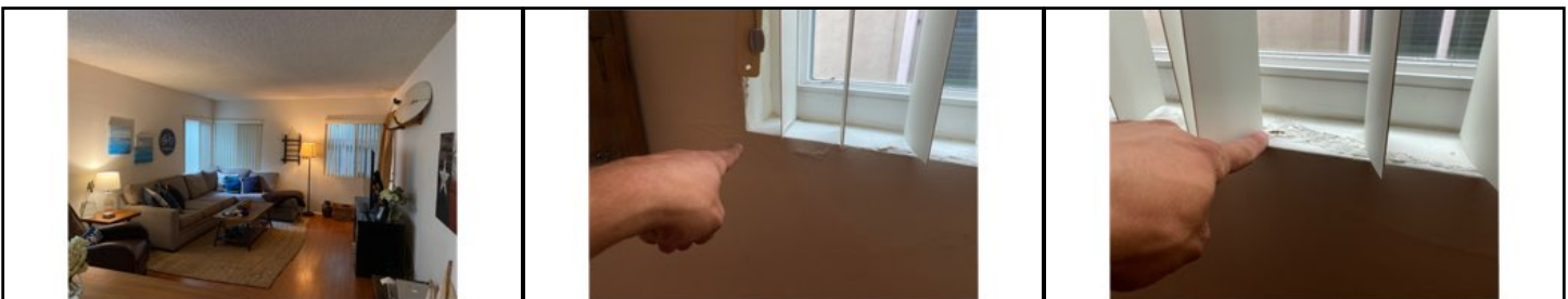
Stains/blistered areas present - tested dry with moisture meter at time of inspection
