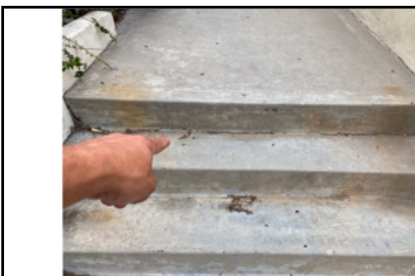
Cracks present at stairs/steps areas
