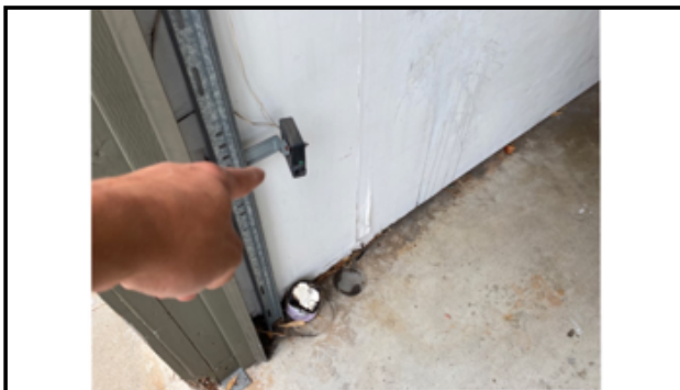
Light beam sensors are installed too high - needs to be serviced (recommended height is between 6 and 8 inches off the ground - manufacturer specifications may differ)
