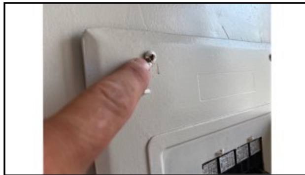
Panel screws stripped - could not remove
