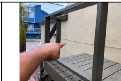
Missing vertical safety rungs - unsafe - needs to be serviced
