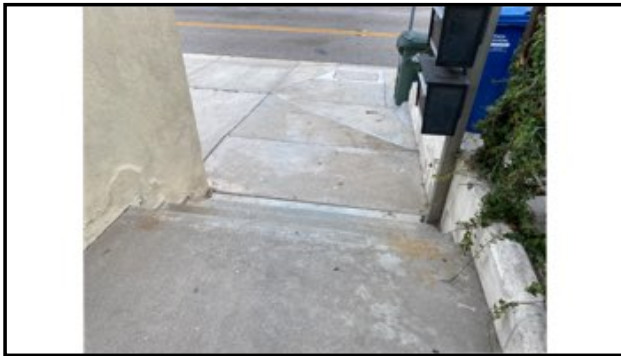
Small localized water ponding may occur in areas - monitor these areas as drains may be needed
