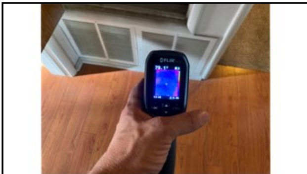
Temperature at Air Return: 80 degrees
