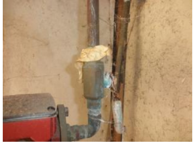
Corroded valve at the water heater.
