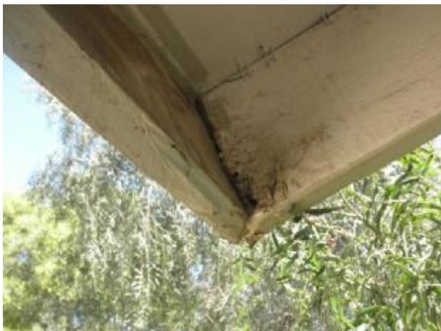
Moisture damage to the fascia board at the NE corner of the roof.
