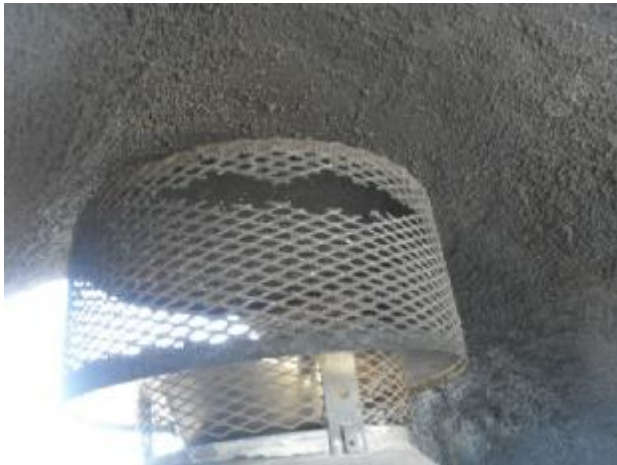
Damaged spark arrestor at the top of the living room chimney.
