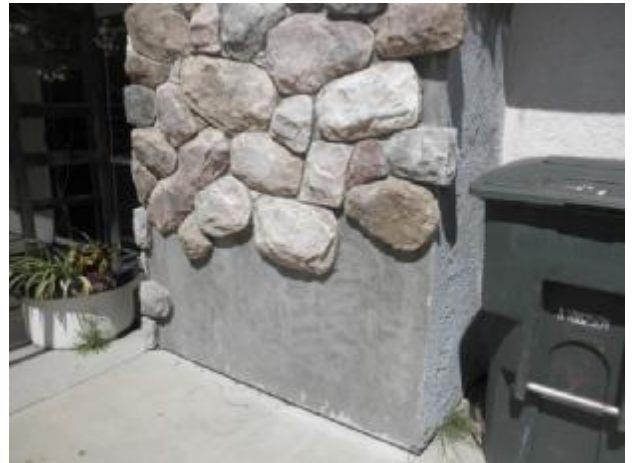
Parts of the stone veneer are missing at the family room chimney enclosure.
