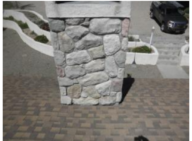
No cricket flashing installed behind the chimney enclosures.
