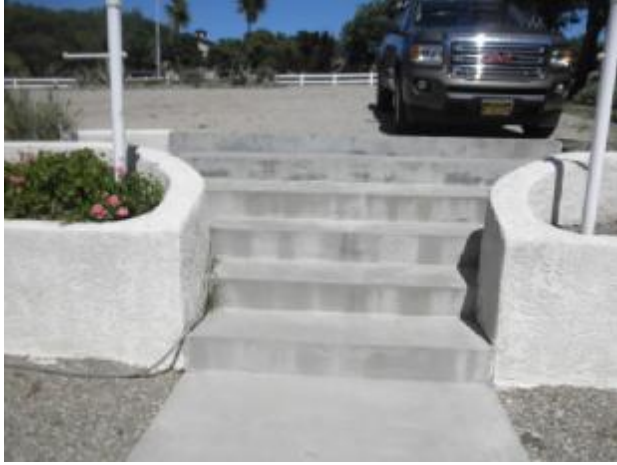
Missing railing at the front entry concrete stairs.
