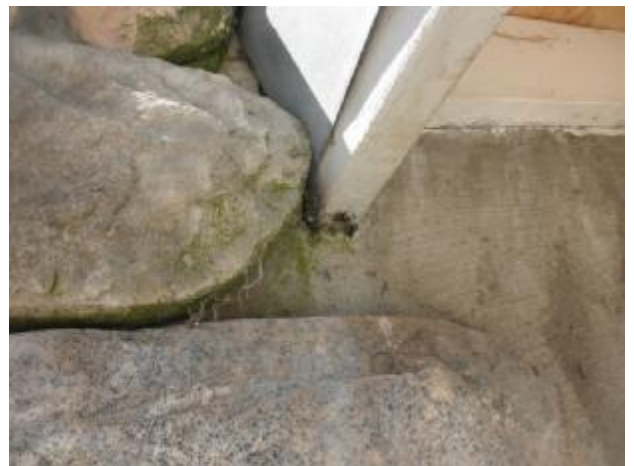
Moisture damage to the fascia board adjacent to the family room chimney enclosure.
