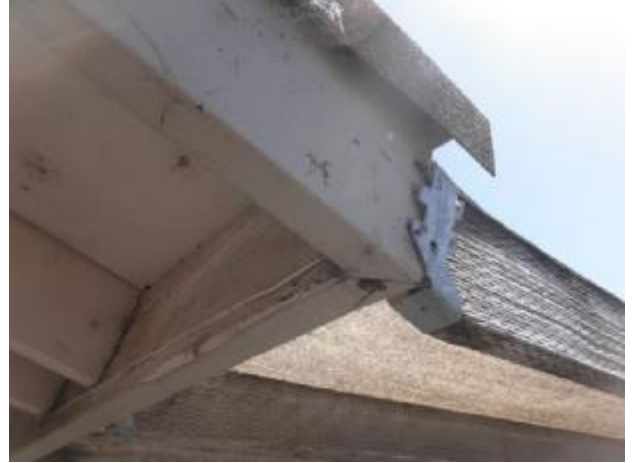
Moisture damage to the fascia board at the SW corner of the roof.
