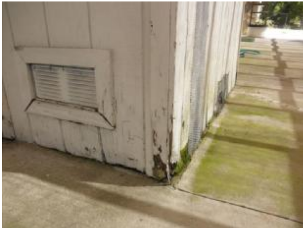
Moisture damage to the base of the water heater closet.
