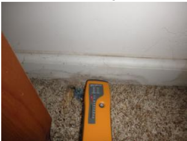
Concealed plumbing leak behind the vanity in the east hall bathroom.
