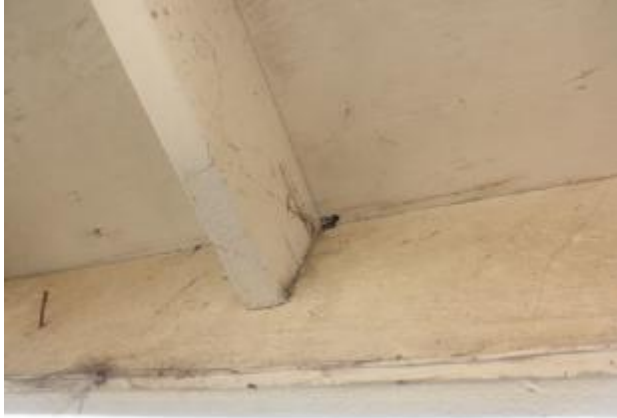
Moisture damage to the eave at the north side of the dining room.
