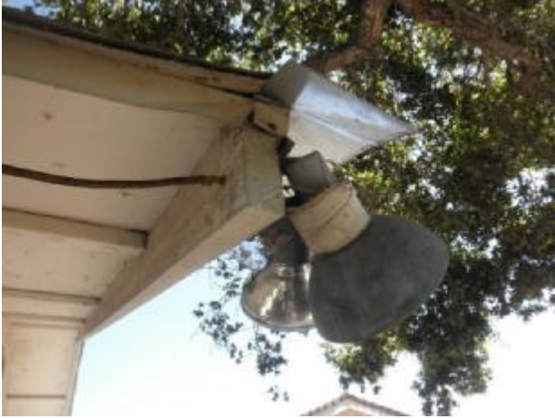
Damaged light fixture at the exterior SW corner of the garage.
