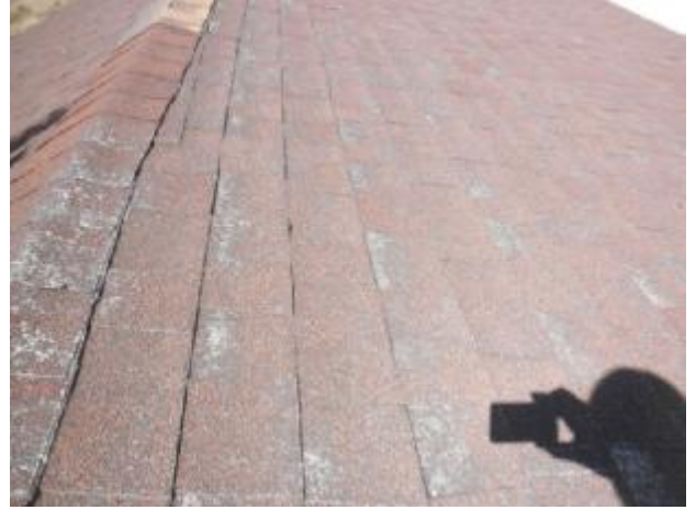
General deterioration of the garage roof shingles.
