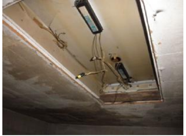
Damaged ceiling light fixtures in the garage.
