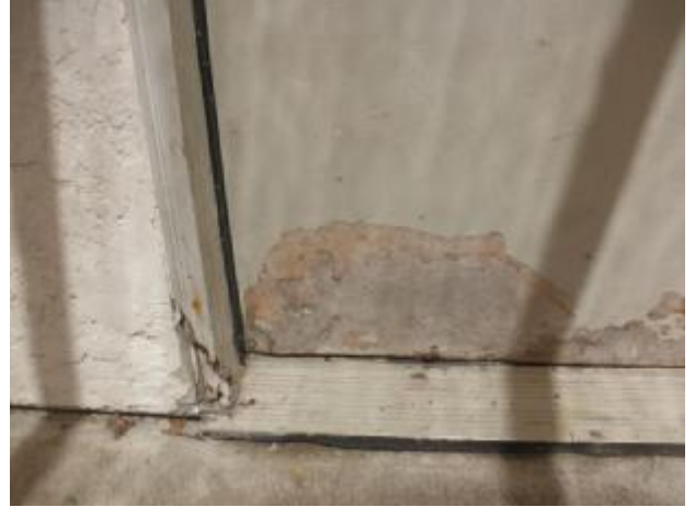
Moisture damage to the exterior door and jamb at the west hall bathroom.
