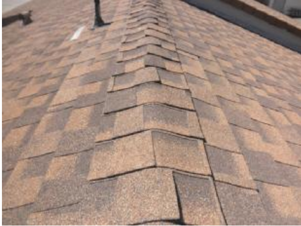
Field shingles used for ridge caps on the roof.
