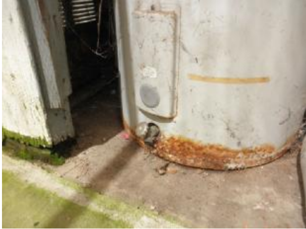
The solar hot water reserve tank is old and beyond a normal life expectancy.
