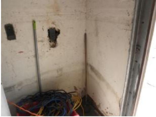
Damaged drywall at the interior SE wall of the garage.
