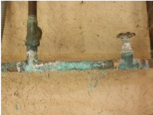
Corroded water line above the water heater.
