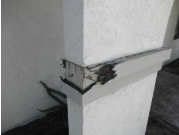
Moisture damage to the wood trim at the front entry arch.
