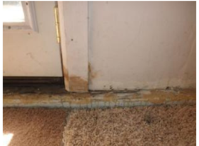
Evidence of water intrusion at the exterior door in the SW bedroom conversion.
