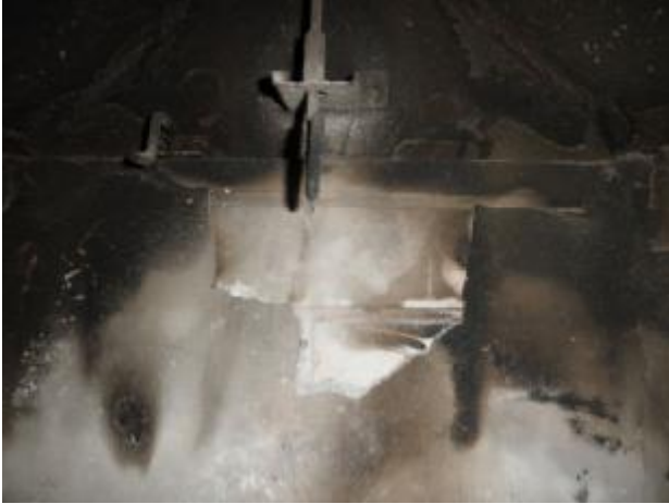
Damaged refractory plate in the living room fireplace.
