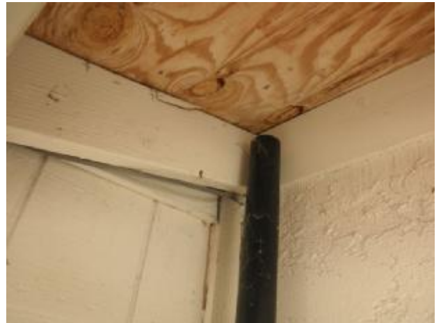
Improperly terminated vent pipe at the exterior north wall of the kitchen.
