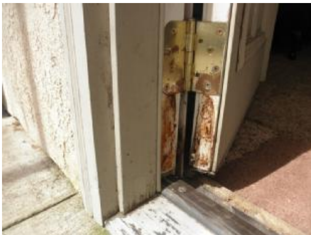
Moisture damage to the door and jamb at the exterior door in the SW bedroom.
