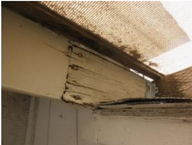
Moisture damage to the fascia board above the water heater closet.
