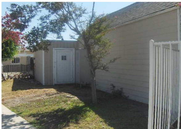
Office Building Side view
