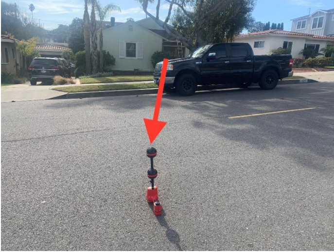
Connection to city sewer under tool.
