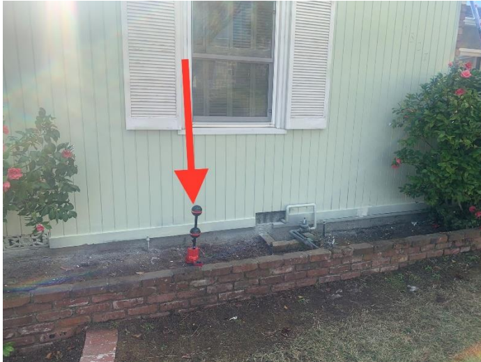
Good location for a cleanout under tool. Depth 3'
