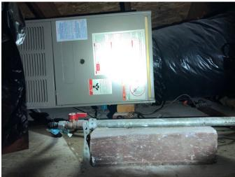
**114:** The heating system is supported by wood blocks. The manufactures required clearance to combustibles should be reviewed as typically the units are not in contact with combustible material.
