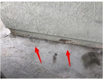
**22:** At the north backyard and west front yard walls, there are holes in the stucco cladding, which should be repaired to prevent water from entering the wall cavity and damaging the home. In addition, the holes are a potential source of entry for insects, rodents and other pests.
