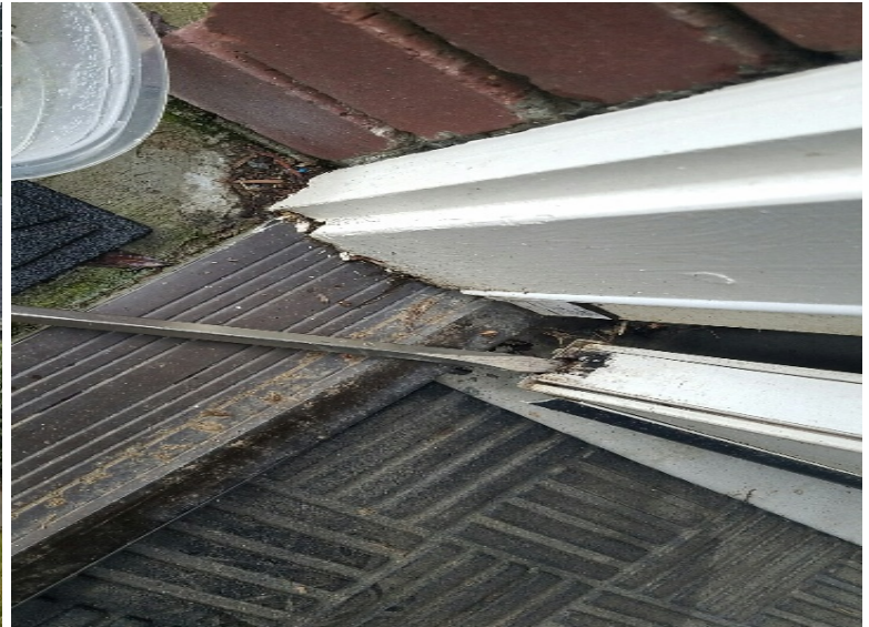
3A - Damaged to the base of the door and door jambs.
