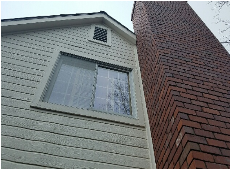
3D - Damaged upper window trim.
