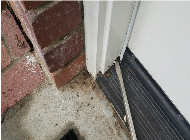
3B - Damaged to the base of the rear door jambs.
