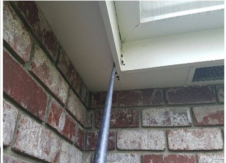
3C - Damaged eaves and fascia.
