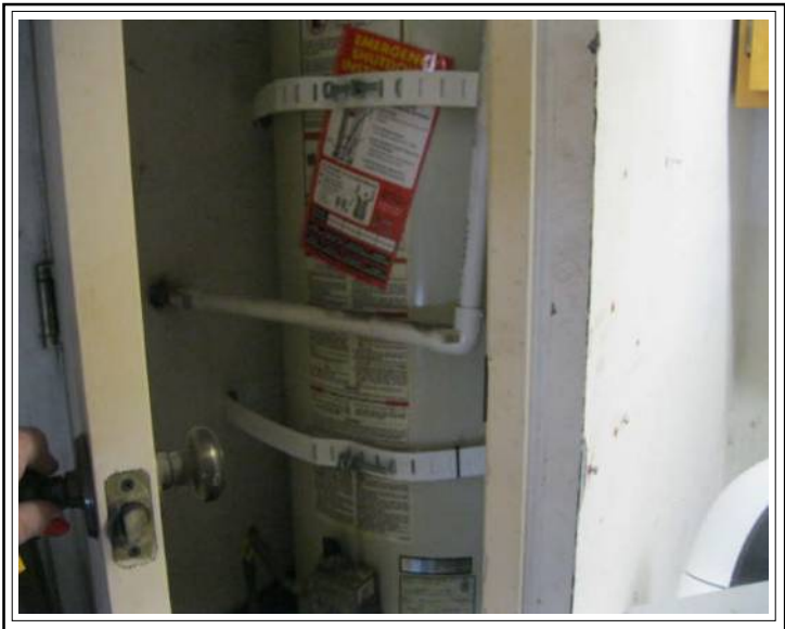
water heater double strapped
