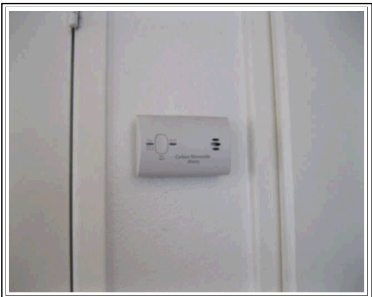
CO detectors installed
