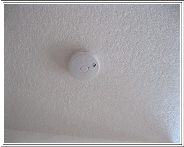
smoke alarms in place
