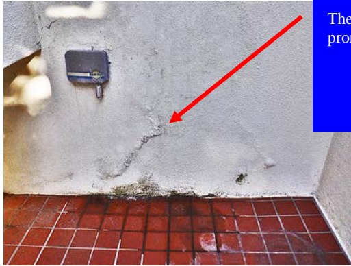
The garage NE-corner shows water damage suspected from a past water heater leak
