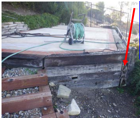
...and the upper patio wood retaining system is deteriorated while the hardscape is off-set
