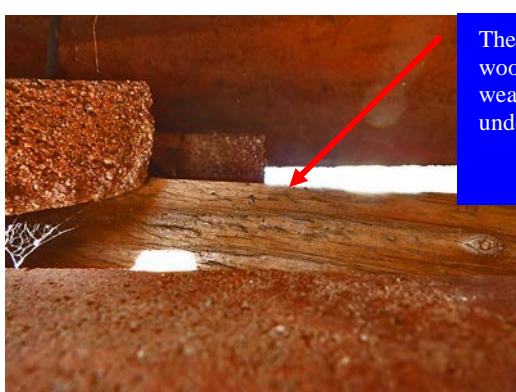
The rear patio trellis wood is weathered
