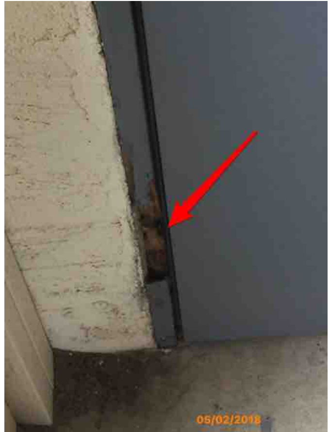
Water heater closet
