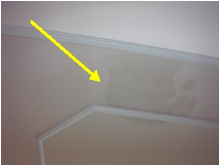
Interior Areas Walls/Ceilings/Floors Condition
