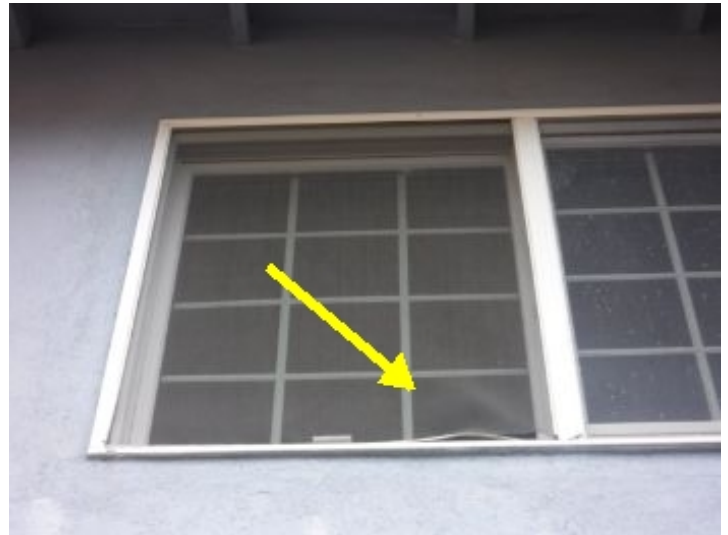
Exterior Areas Window Condition
