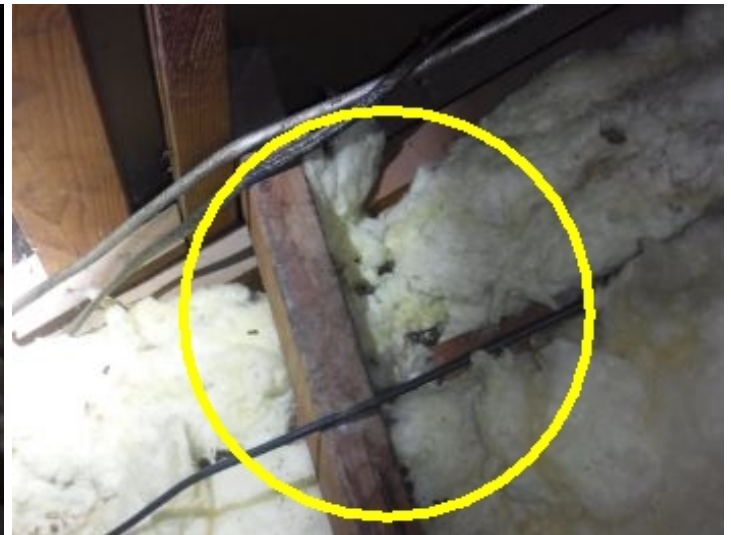
Attic Insulation Condition
