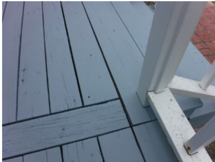
Foundations and Floors Patio and Porch Deck
