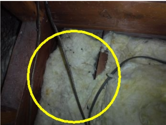
Attic Insulation Condition
