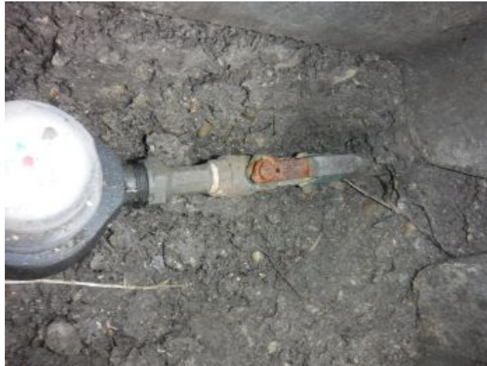
Foundations and Floors Plumbing
