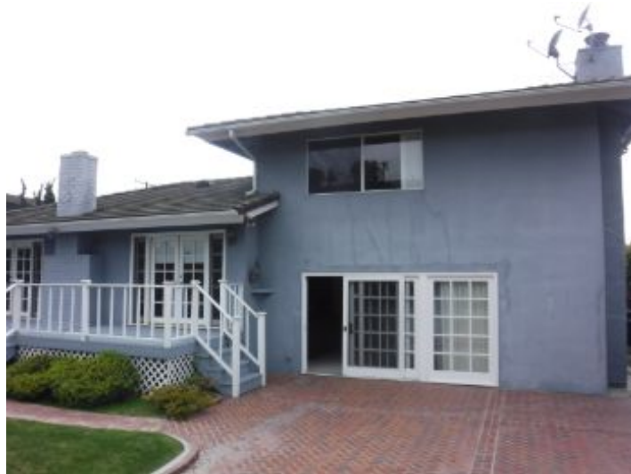
Foundation Slab Foundation
