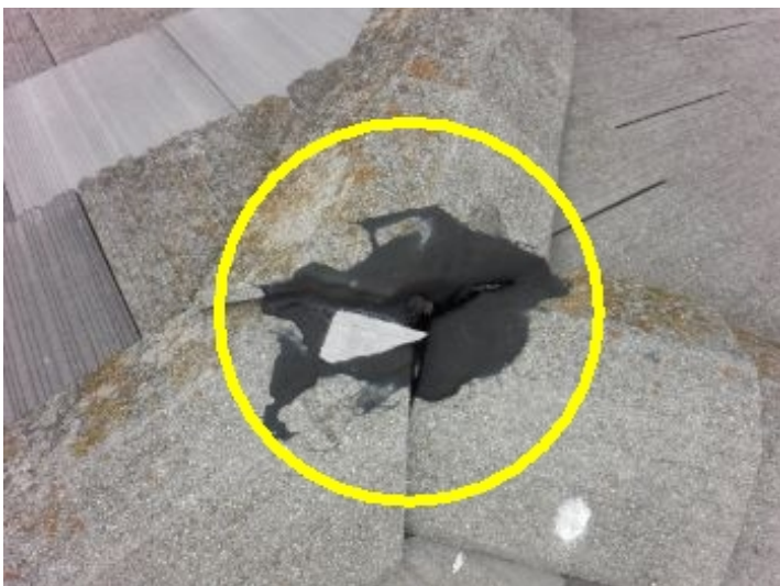
Roof Roof Condition
