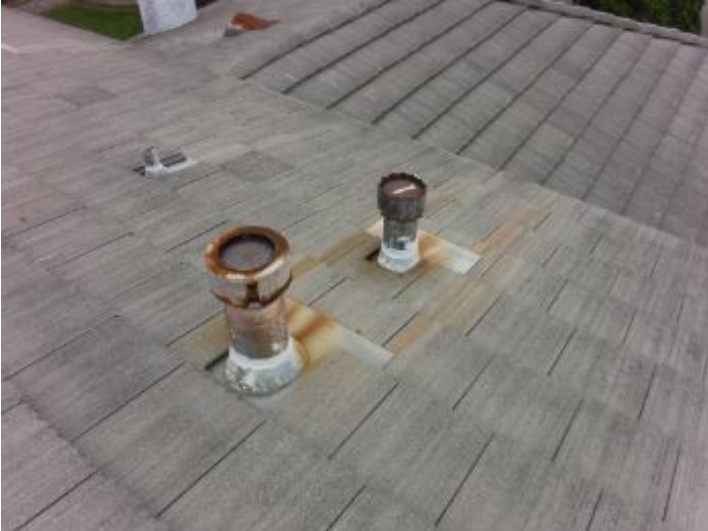
Roof Flashing
