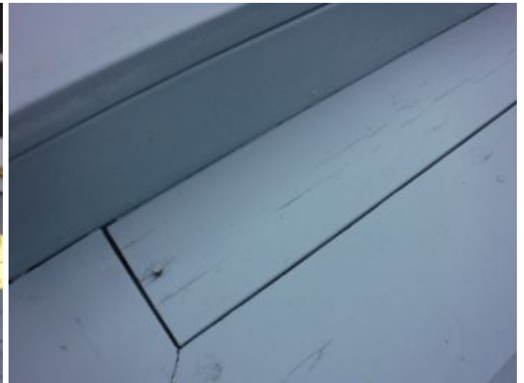
Foundations and Floors Patio and Porch Deck
