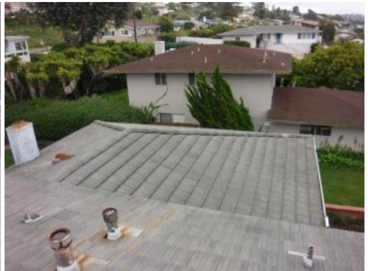
Roof Roof Condition
