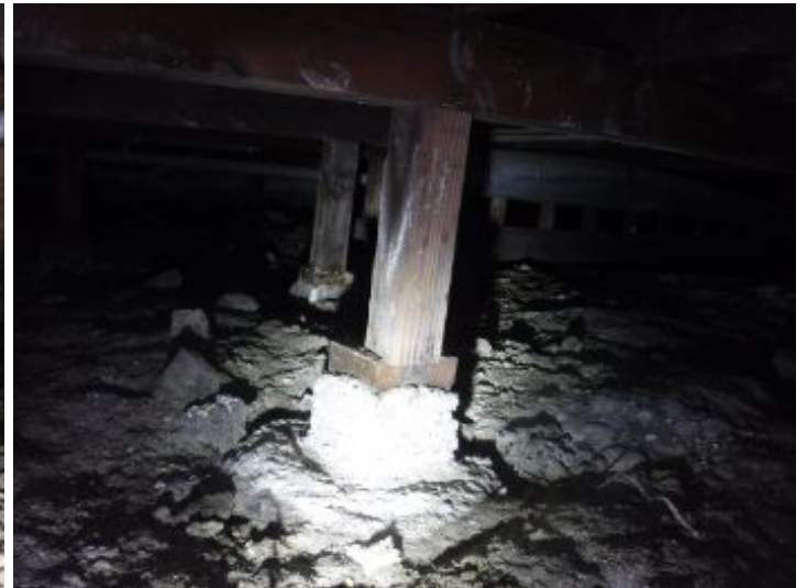
Foundation Post and Girders
