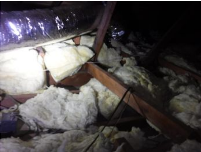
Attic Insulation Condition
