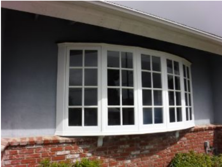
Exterior Areas Window Condition
