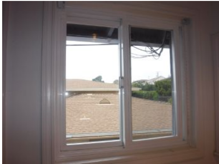
Interior Areas Window Condition
