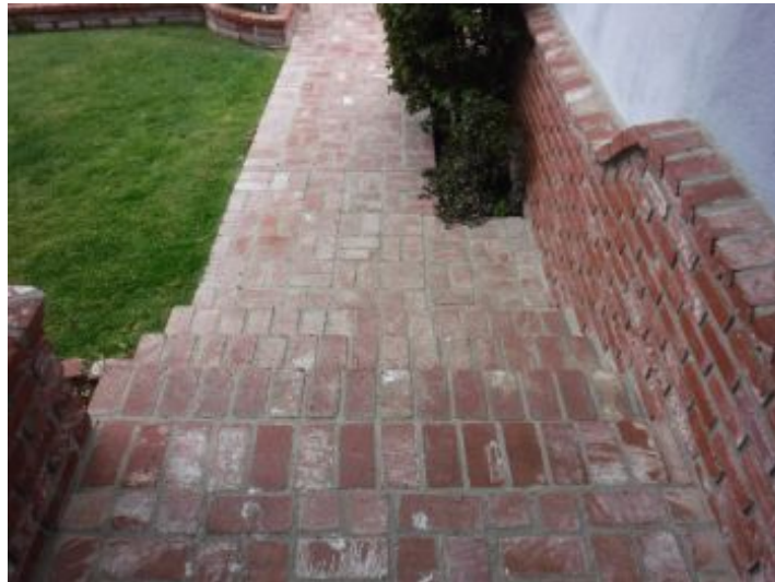
Foundations and Floors Stairs & Handrail
