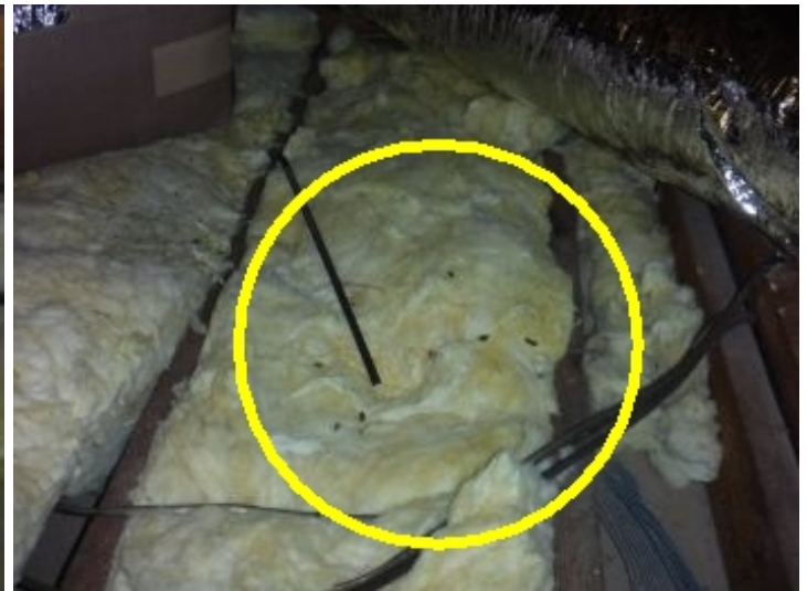
Attic Insulation Condition
