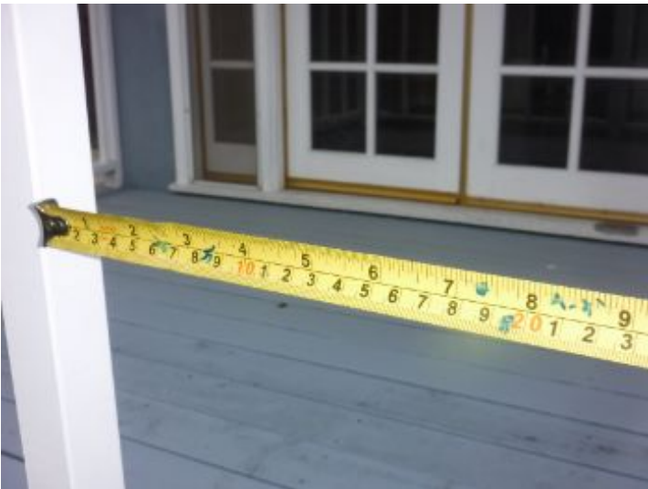
Foundations and Floors Patio and Porch Deck
