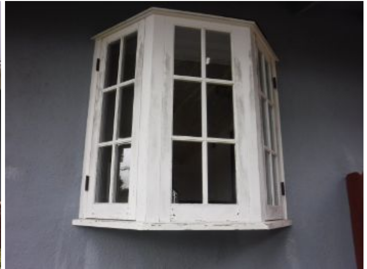
Exterior Areas Window Condition
