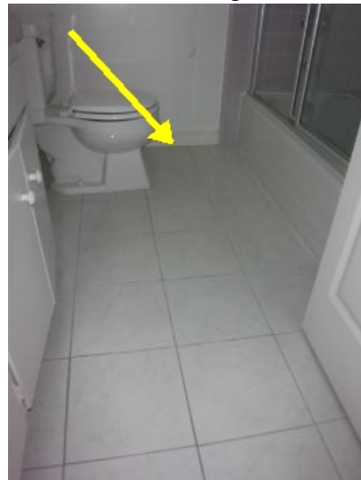
Interior Areas Walls/Ceilings/Floors Condition
