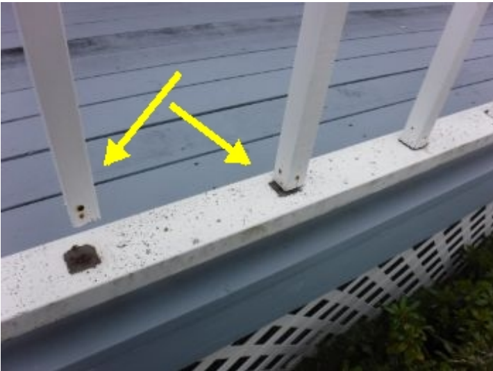
Foundations and Floors Patio and Porch Deck
