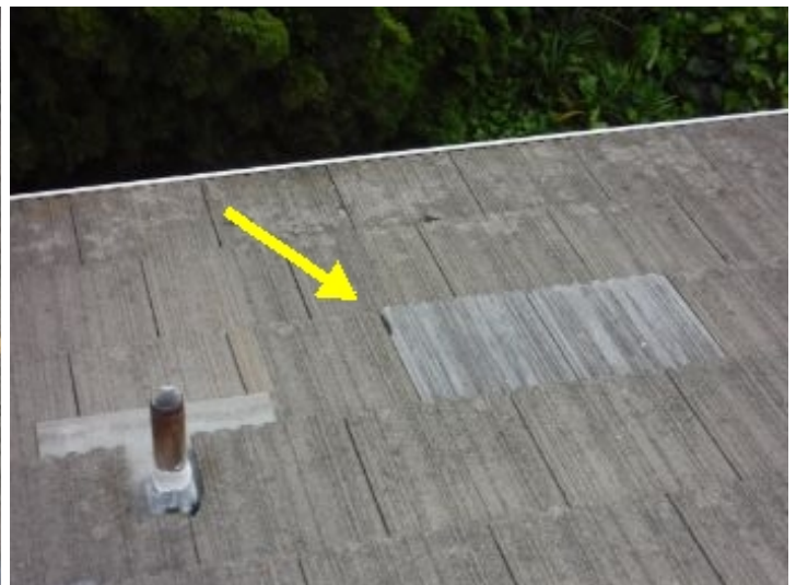
Roof Roof Condition
