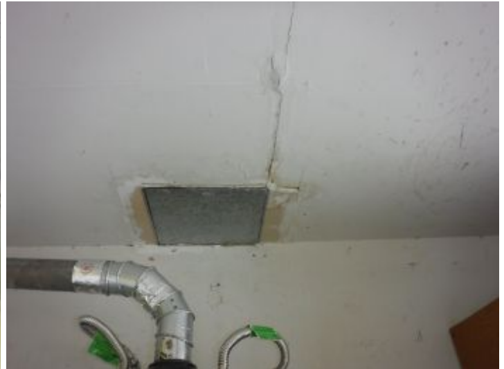
Garage Rafters & Ceiling
