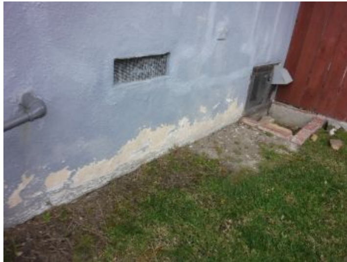
Exterior Areas Siding Condition
