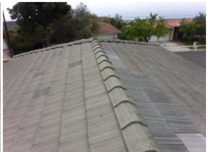
Roof Roof Condition
