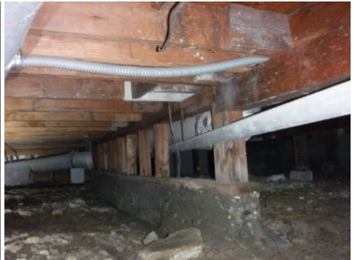
Foundation Cripple Walls
