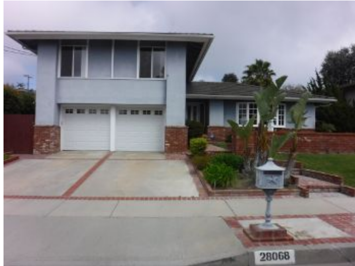
Foundations and Floors Driveway and Walkway Condition
