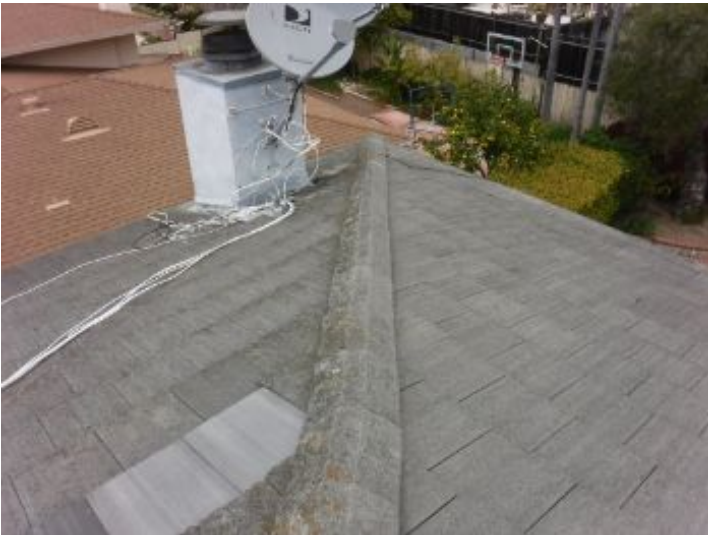
Roof Roof Condition
