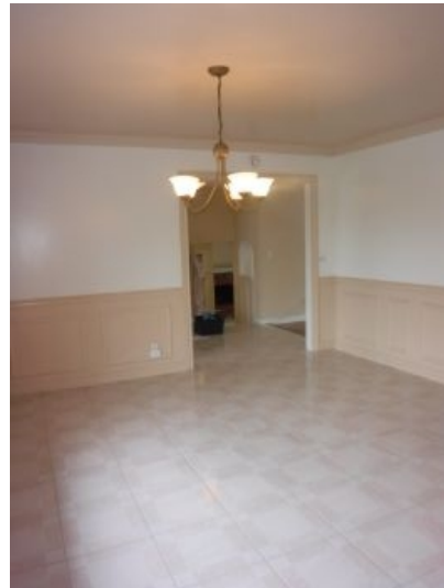
Interior Areas Walls/Ceilings/Floors Condition
