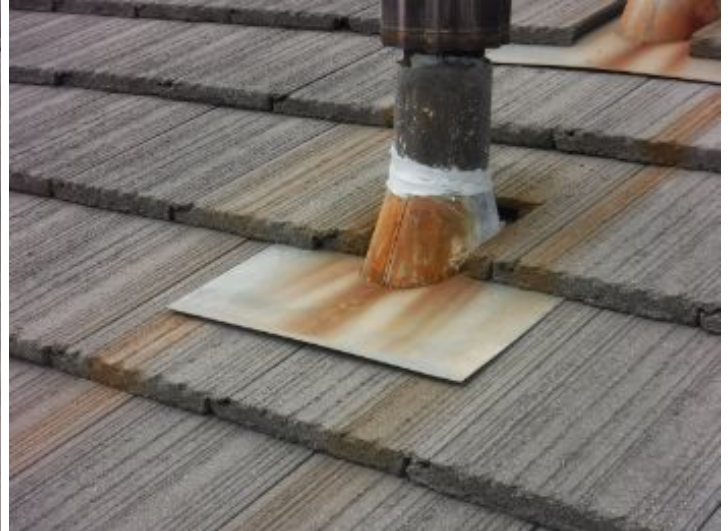
Roof Flashing
