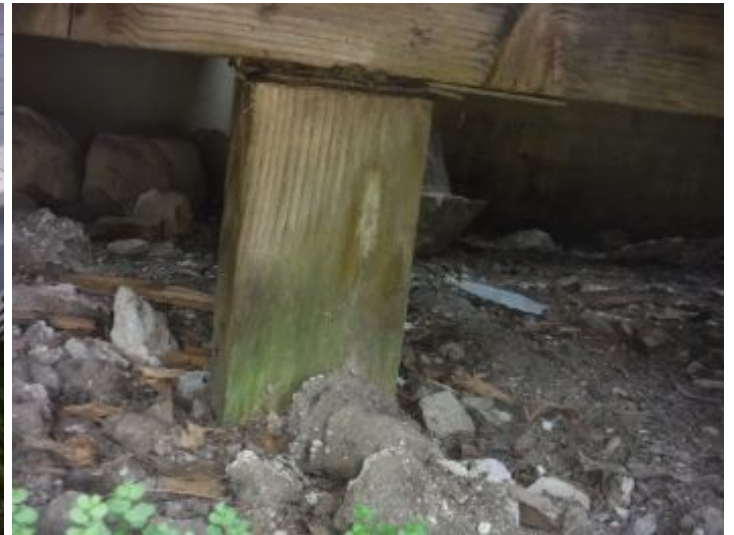
Foundations and Floors Patio and Porch Deck
