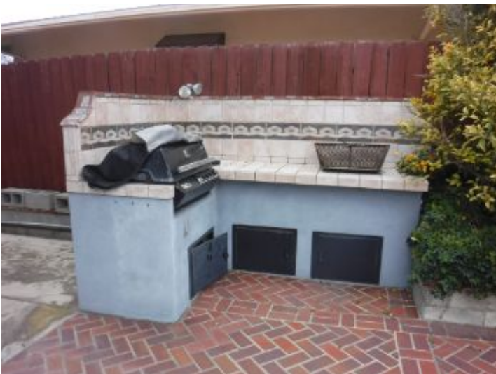
Foundations and Floors Patio and Porch Deck
