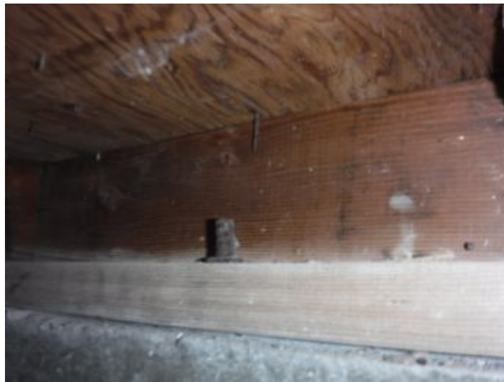
Foundation Anchor Bolts
