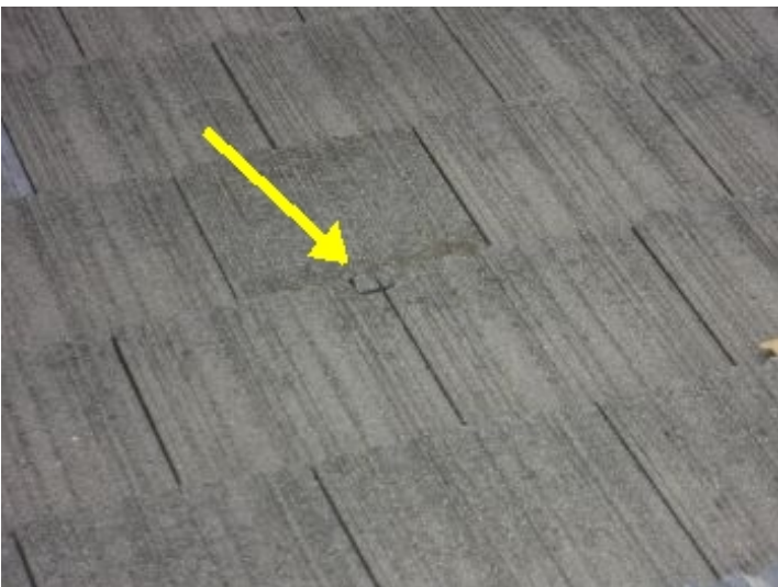
Roof Roof Condition
