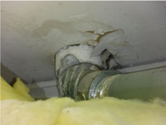
Garage Rafters & Ceiling
