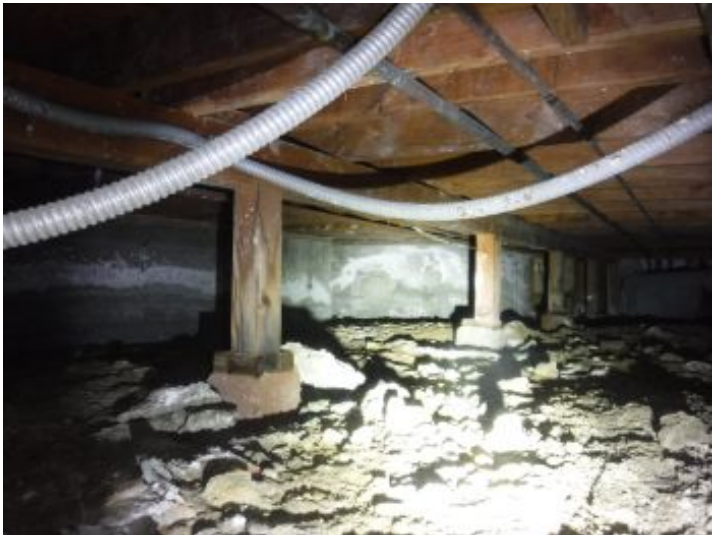
Foundation Post and Girders
