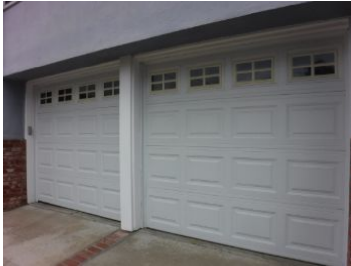
Garage Garage Door Condition
