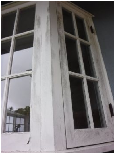
Exterior Areas Window Condition
