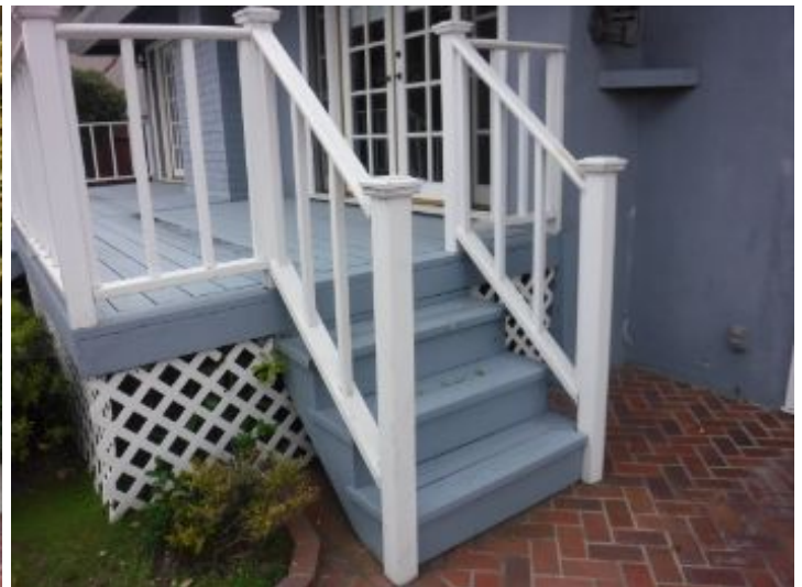
Foundations and Floors Patio and Porch Deck
