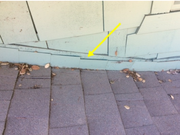
There is flashing but no counter flashing where a portion of the roof abuts the house, and moisture intrusion would be possible. Therefore, this connection will need to be monitored and serviced as necessary.
