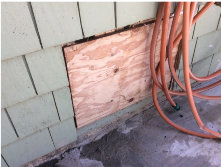
The house wall finish is generally in acceptable condition but has a unfinished repair that should be serviced.
