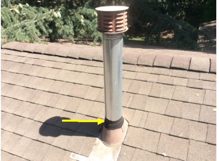
A rain-collar is missing on a heat vent which you may wish to have installed.
