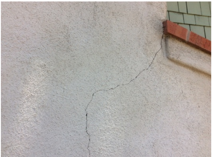
There are small cracks in the stucco around some of the windows and doors that result from movement, and are quite common. Stress fractures can reappear after they have been repaired, and particularly if they have not been repaired correctly.
