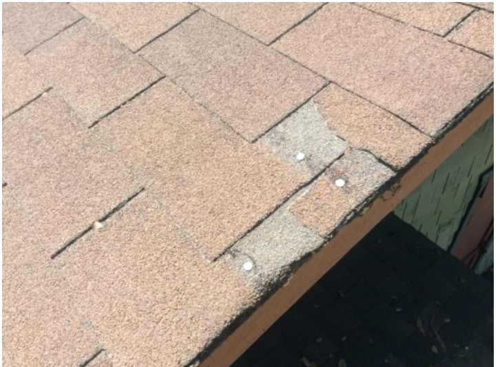
The roof has one or more damaged or missing shingles that should be repaired by a licensed roofing contractor.
