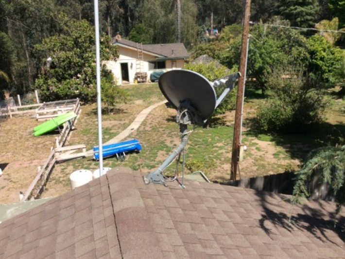
The roof includes a satellite dish that has been installed by bolting through the roof, which can be a common point of leaks and should be monitored.
