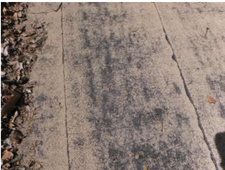
8. ● Roof is weathered and deteriorated. @@ garage & bonus room - See example at photo page) X 2
