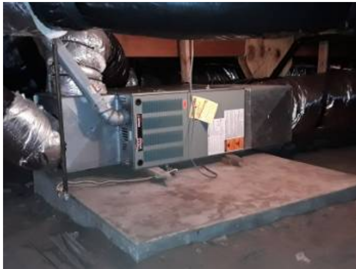
Central heat is provided by a forced-air furnace that is located in in the crawlspace.
