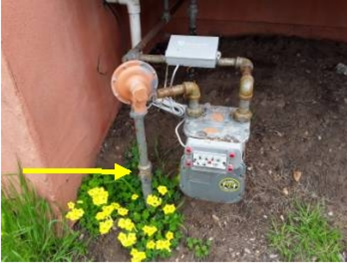
The gas main shut-off is located on right side of the home, unit or building.
