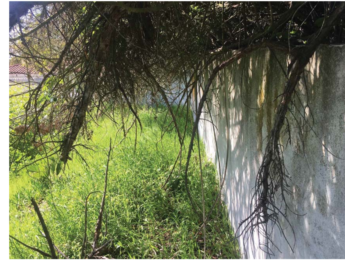
4 NORTH-EAST CORNER LOOKING INTO BACK YARD
