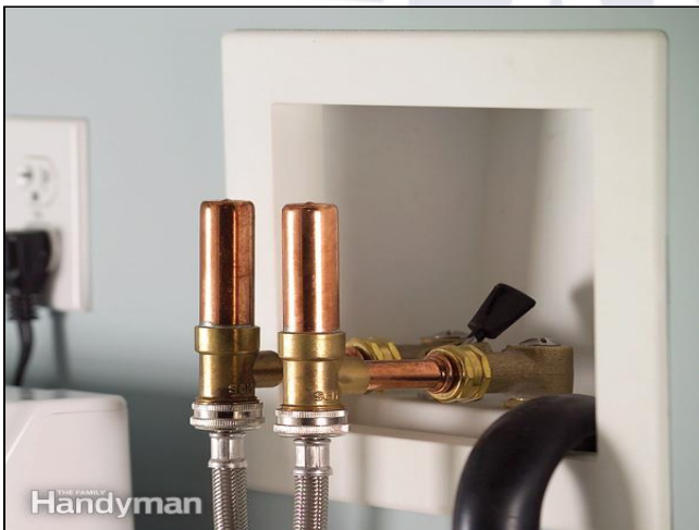
7.6 Item 1(Picture) HV
