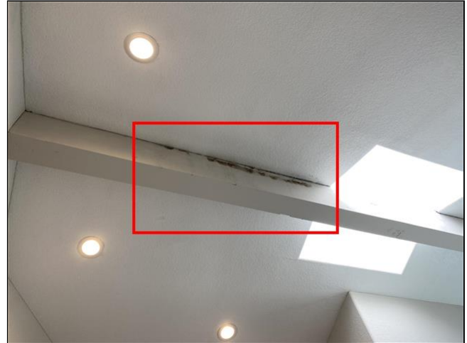
8.1 Item 2(Picture) Interiors
