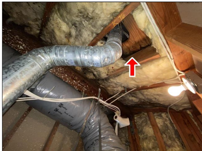
Item 5 - Item 2(Picture) Structural Components
