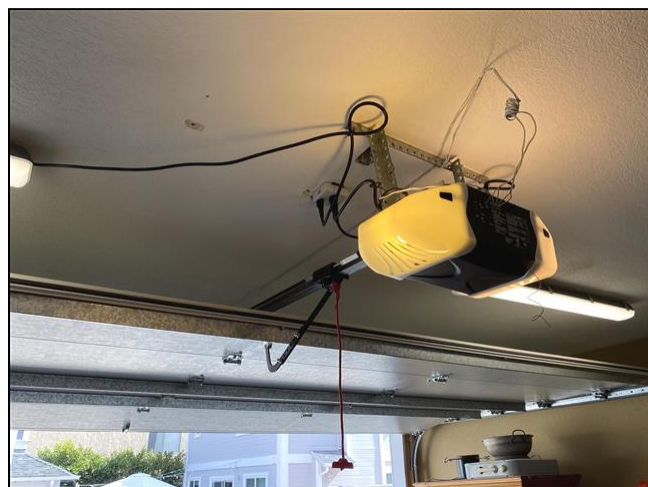
9.2 Item 1(Picture) Garage
