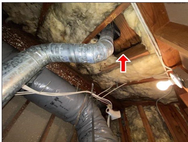
3.5 Item 2(Picture) Structural Components
