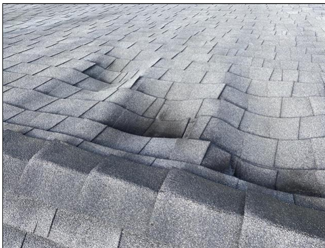
Item 1 - Item 4(Picture) Roofing
