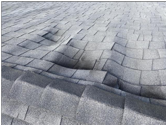
1.0 Item 4(Picture) Roofing
