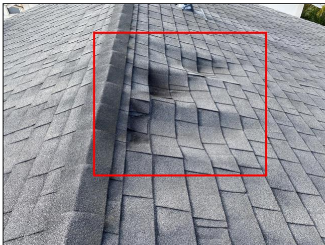
Item 1 - Item 3(Picture) Roofing
