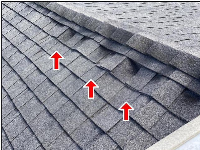
Item 1 - Item 1(Picture) Roofing
