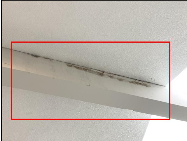
8.1 Item 1(Picture) Interiors
