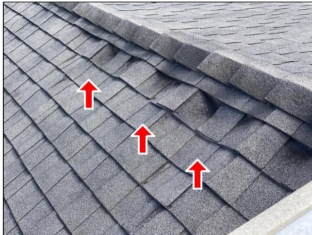
1.0 Item 1(Picture) Roofing
