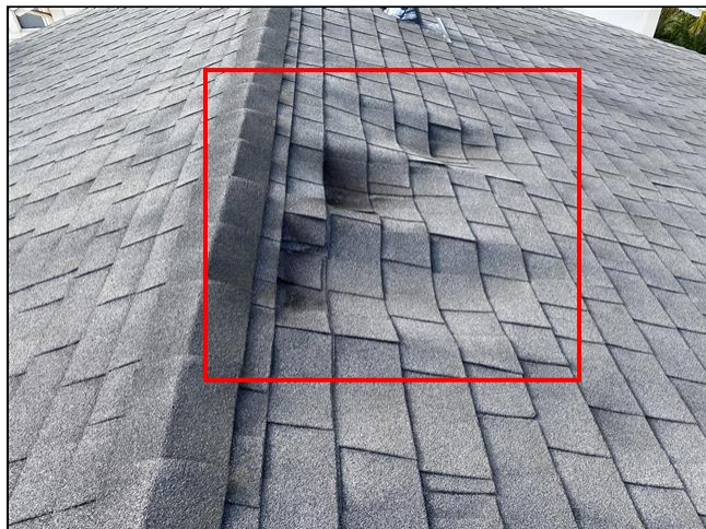
1.0 Item 3(Picture) Roofing
