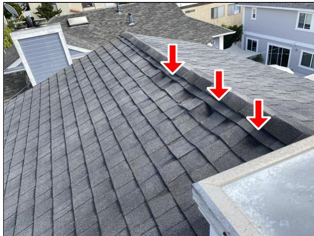
Item 1 - Item 2(Picture) Roofing
