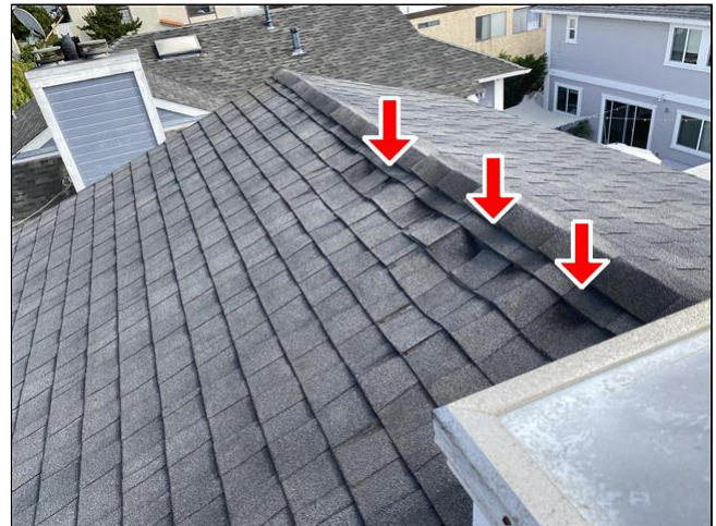
1.0 Item 2(Picture) Roofing
