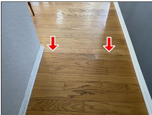
8.2 Item 1(Picture) Interiors
