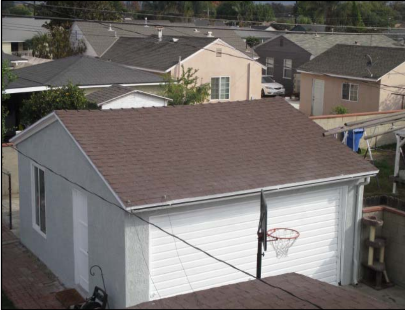
Comments: View of garage roof
