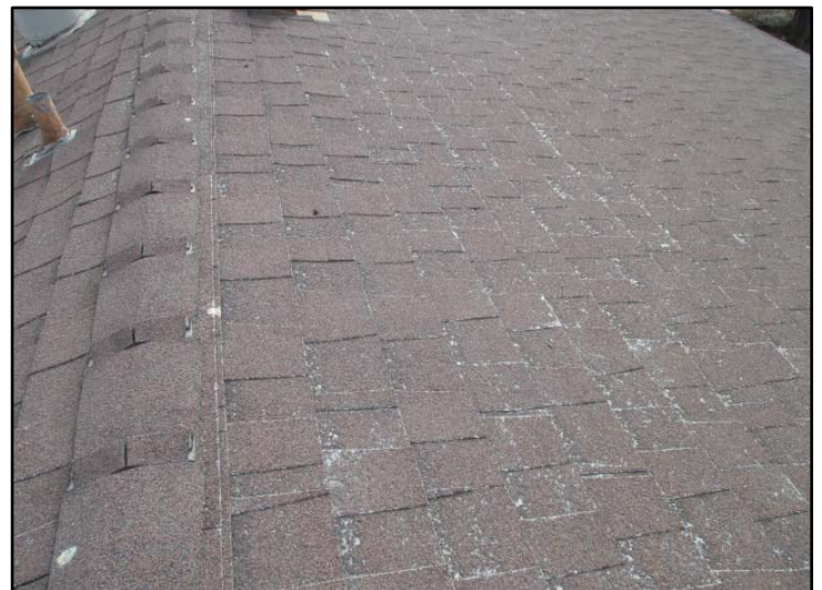
Comments: View of roof material, showing signs of weathering, further evaluation is needed
