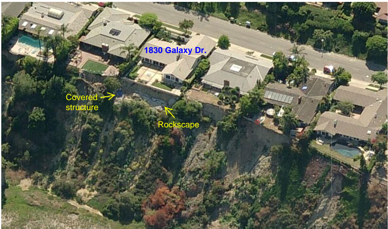
Photo 26: An aerial photo from June 22, 2005, following heavy winter rains. A large slope failure has occurred on the bluff behind several homes. Note that the rockscape and covered structure have fallen down the bluff.
