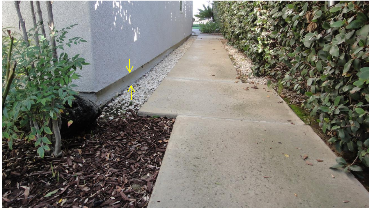
Photo 13: An overview of the right side yard. There is good clearance between the weep screed and the ground elevation. DSC00022.JPG
