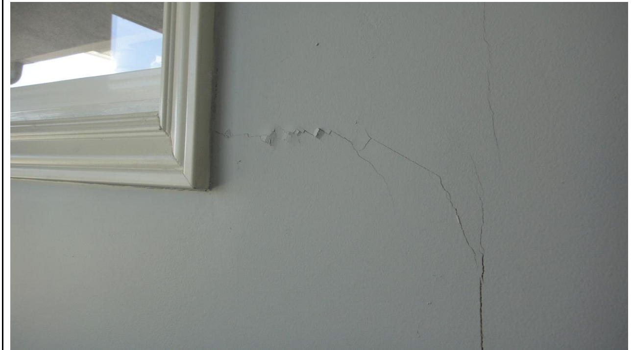
Photo 6: A closer view of the cracking. DSC00060.JPG
