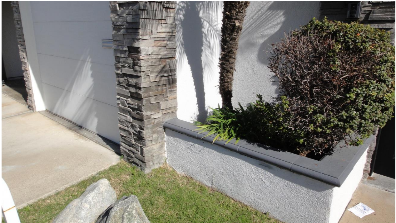
Photo 12: The raised planter at the front right corner of the garage. Water is intruding into the garage from the planter. DSC00083.JPG
