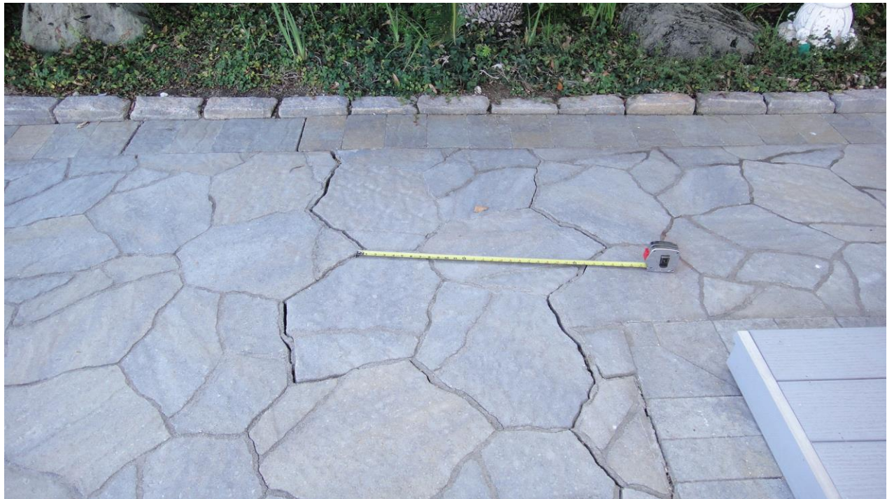
Photo 24: Patio separations at the right side of the patio. These separations also indicate movement toward the bluff.
