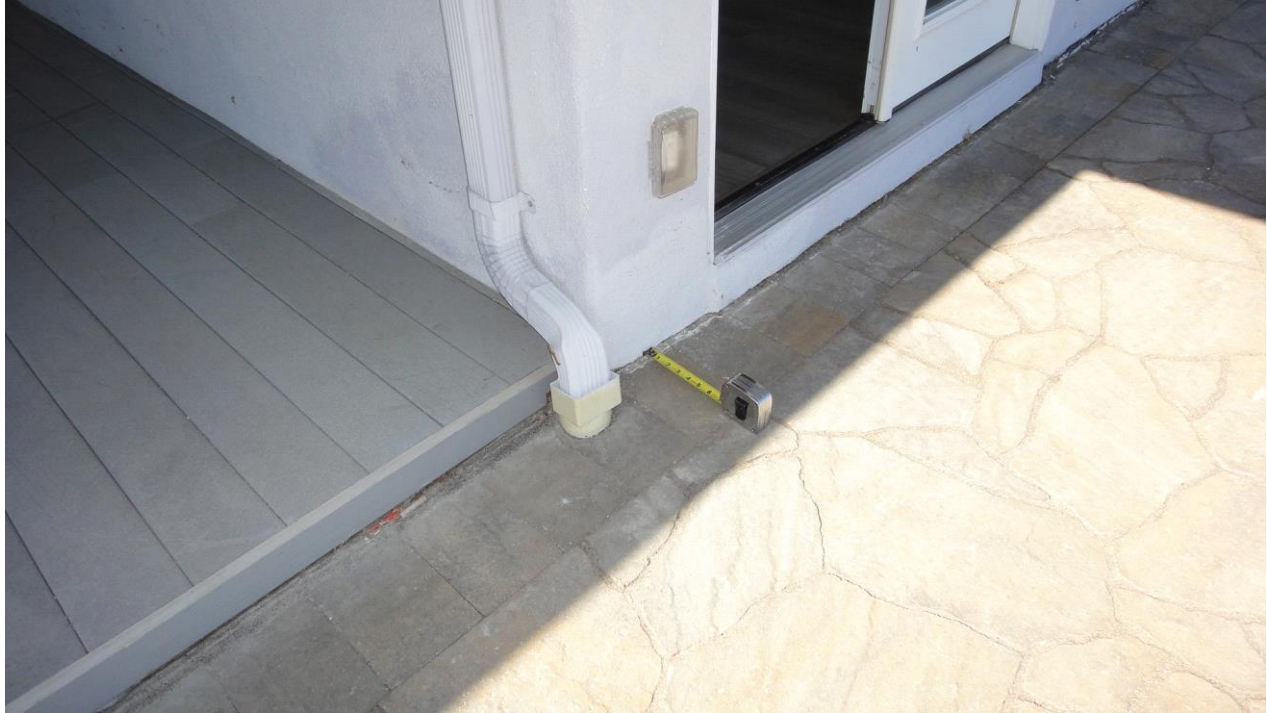
Photo 19: A view of the patio where it meets the rear of the residence. The patio has moved toward the bluff.
