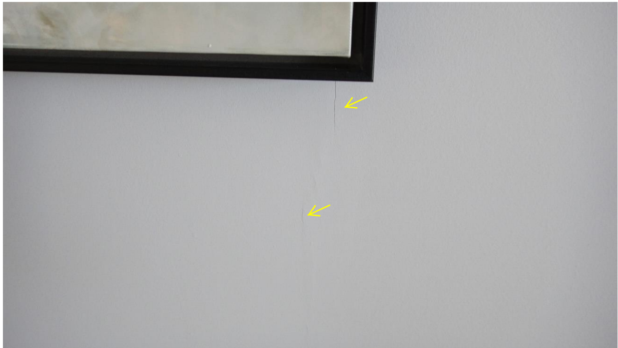
Photo 4: A closer view of the hairline wall cracking.
