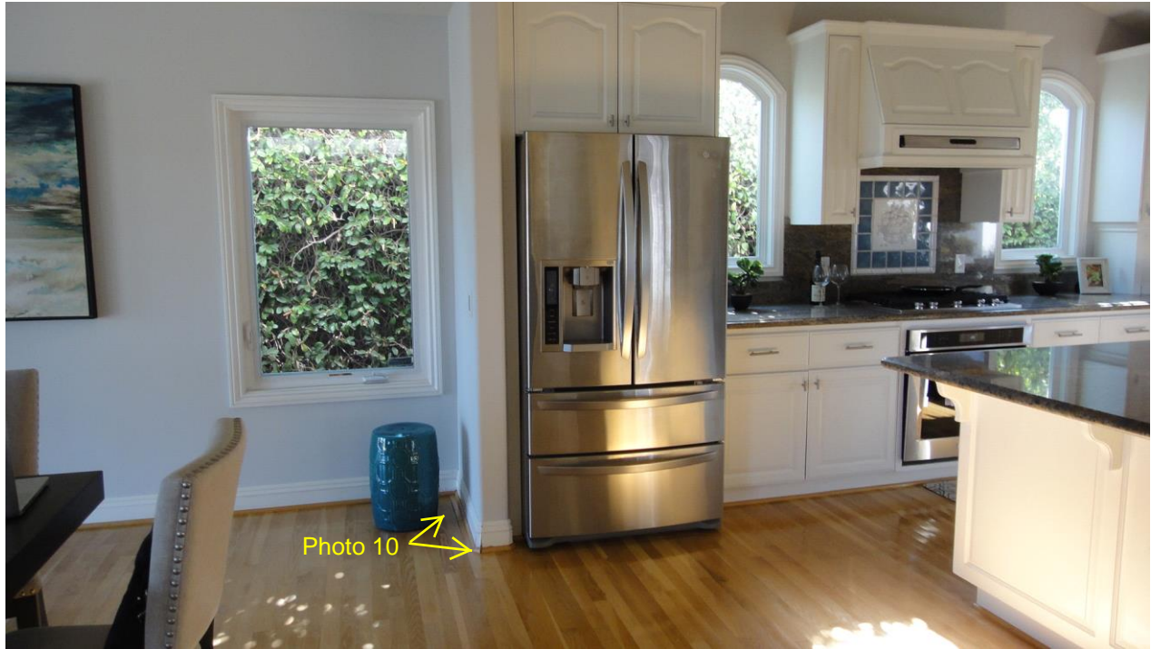
Photo 9: A view of the right side of the kitchen. There are baseboard and floor separations next to the refrigerator, likely due to a past leak. DSC00065.JPG
