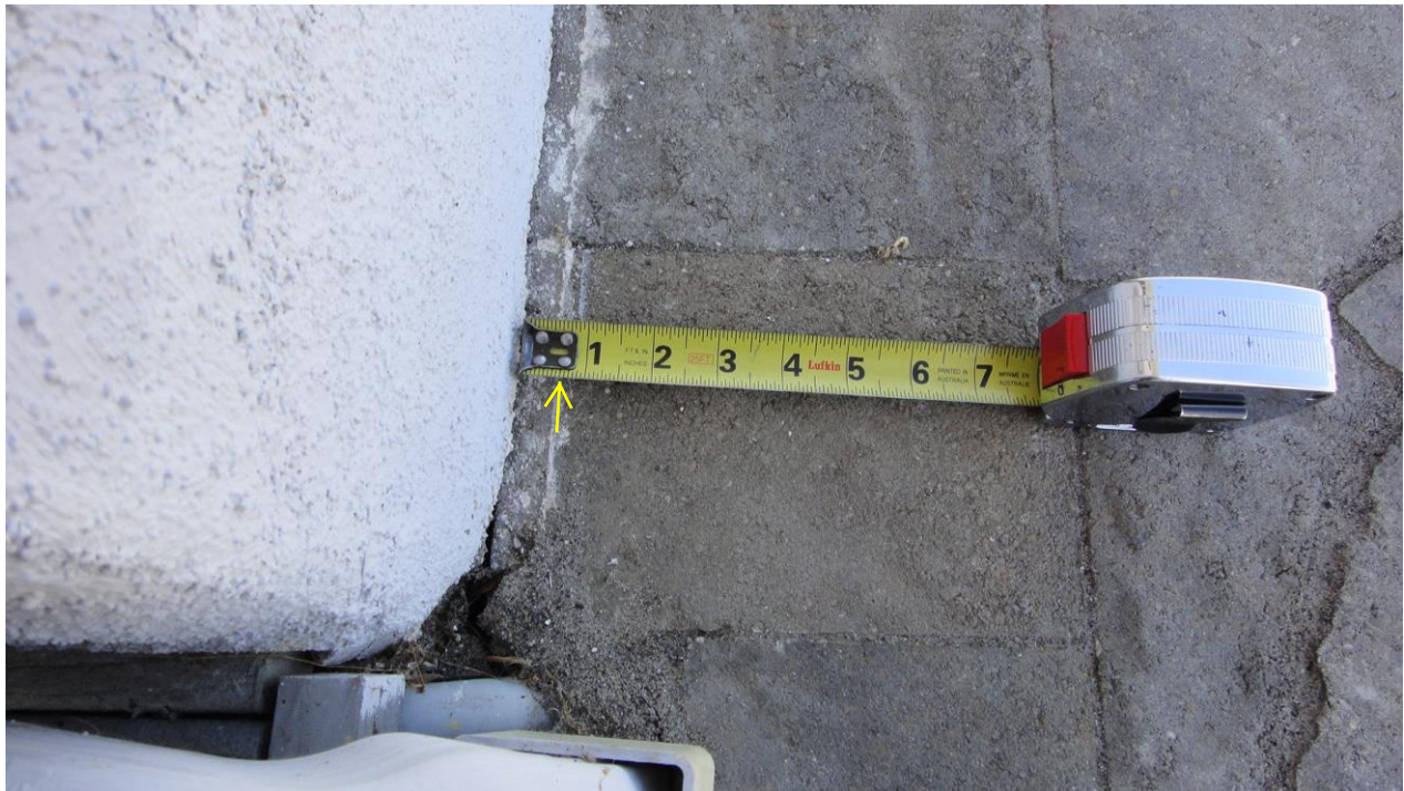
Photo 20: A closer view of patio movement toward the bluff, measuring about 1/2 of an inch.
