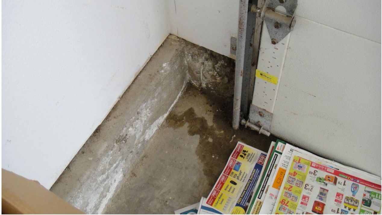
Photo 11: Water intrusion and efflorescence (white salt deposits) at the front right corner of the garage. DSC05242.JPG
