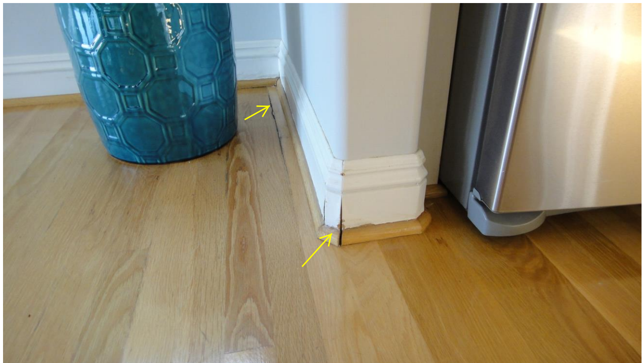
Photo 10: A closer view of the baseboard and floor separations. DSC00066.JPG
