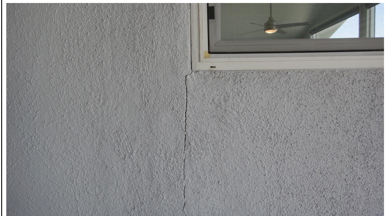
Photo 18: A closer view of the stucco cracking. DSC00055.JPG
