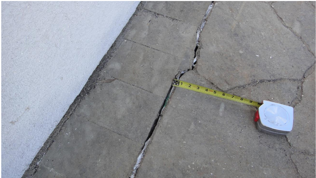
Photo 22: Another patio separation at the rear of the residence. This separation is also indicative of movement toward the bluff.
