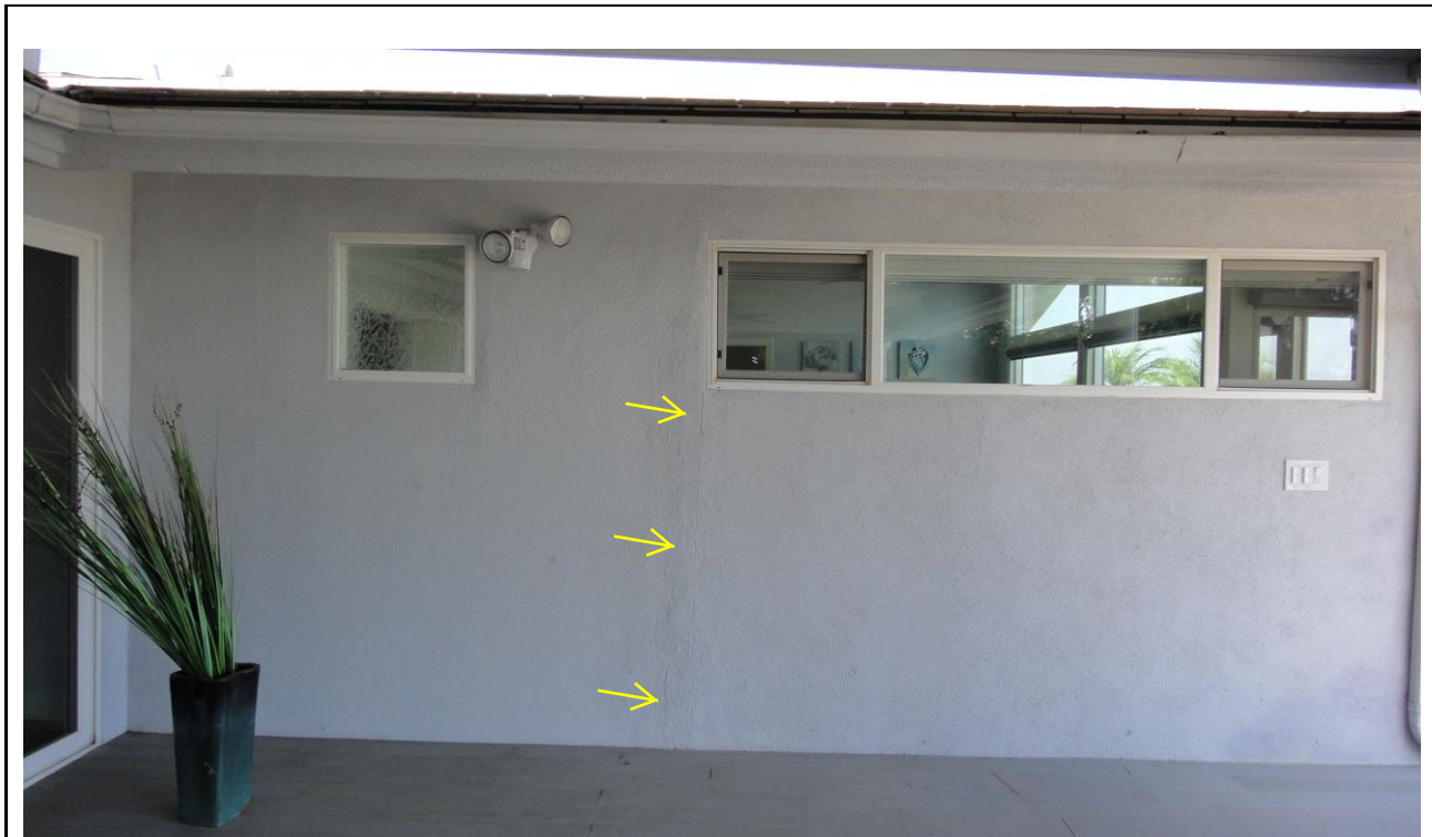
Photo 17: A view of the exterior wall of the master bedroom. There is stucco cracking where a sliding glass door used to be (see Photo 5). DSC00031.JPG
