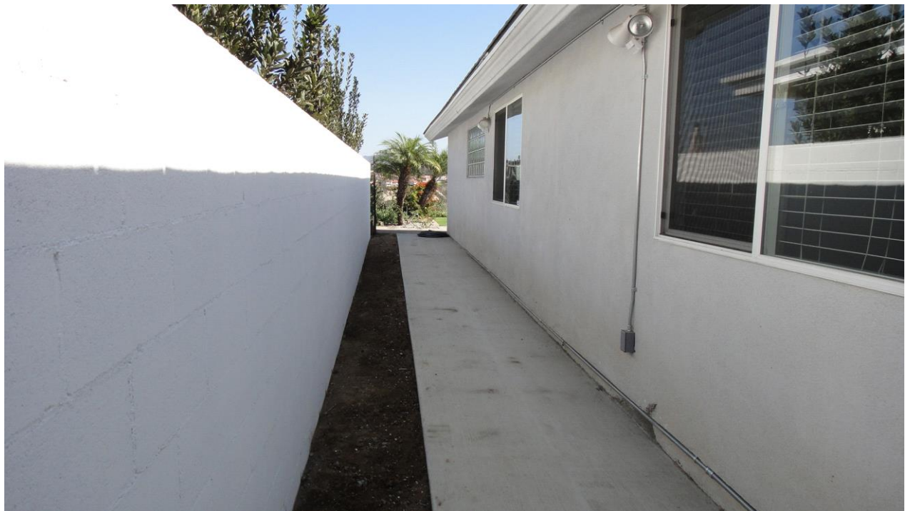
Photo 14: An overview of the left side yard. The side yard concrete is sloped to drain toward the street. DSC05200.JPG
