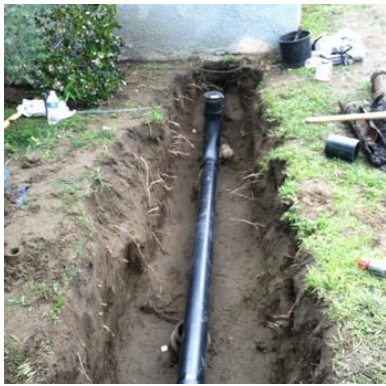
ABS (Acrylonitrile Butadiene Styrene) Color: Usually black Life Expectancy: 50 to 70+ years
