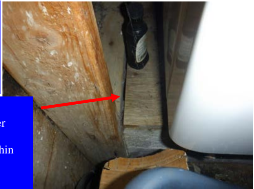
The HVAC system's return air chamber is filthy and this area communicates with the framing cavity below the clothes dryer...
