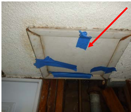
...and the improper ceiling access hatch
