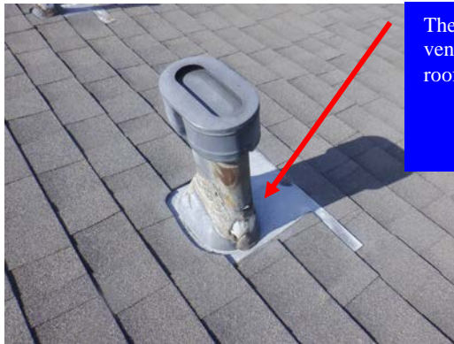
...where a 'storm collar' is needed (sample photo)
