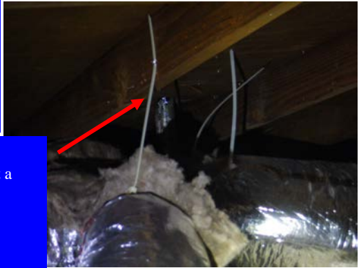
The master bath exhaust fan is discharging to the attic and is adjacent to an open electrical box
