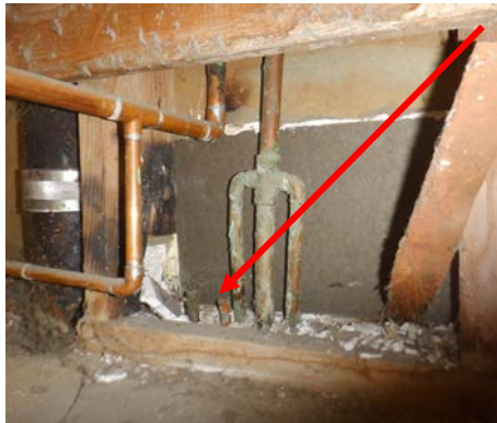
Inspection of the return air chamber also revealed abandoned copper water supply piping embedded within the slab
