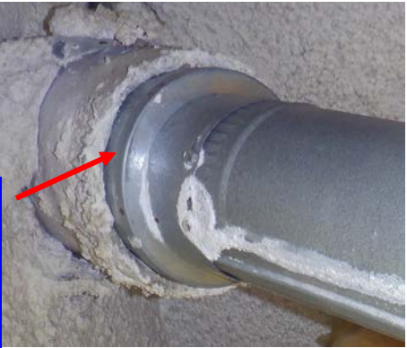
...where a 'vent increaser' fitting is needed (sample photo)
