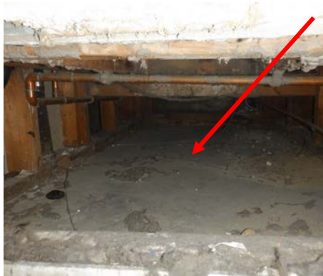
The HVAC system's return air chamber is filthy and this area communicates with the framing cavity below the clothes dryer...
