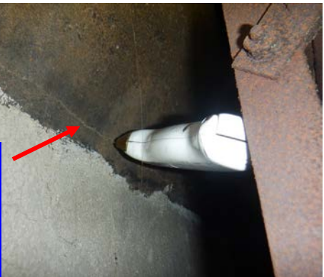
The pre-cast concrete fireplace has developed a horizontal crack across the 'insulation plate'
