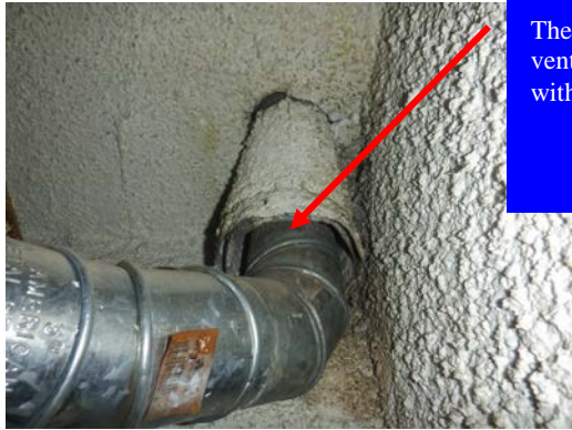
...where a 'vent increaser' fitting is needed (sample photo)
