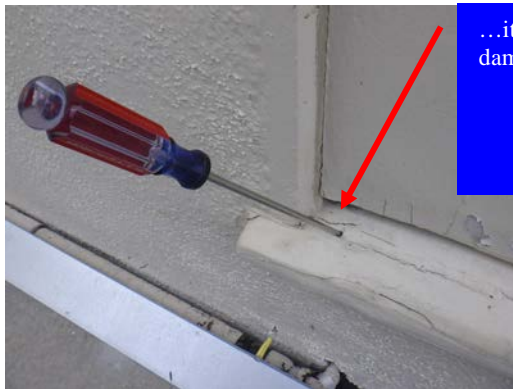
...damage was also noted at the garage exterior service door trim...
