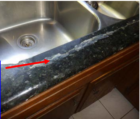
...while the sink area countertop shows extensive damage...
