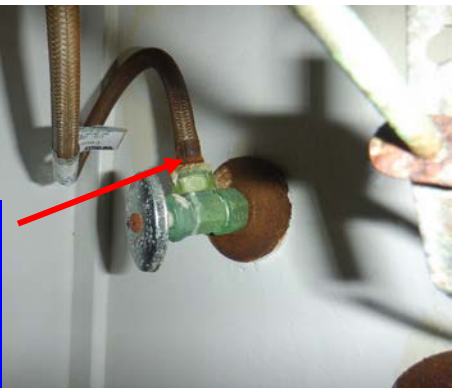
A few of the water supply connectors within the sink cabinets show corrosion
