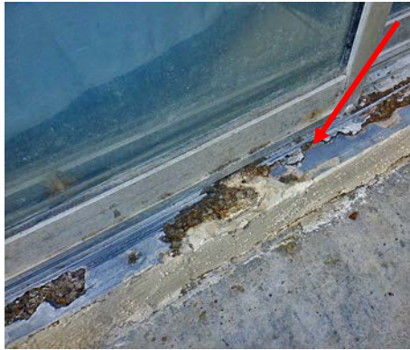
The sliding glass door is very difficult to operate and its track has nearly fully corroded away
