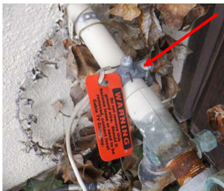
A low voltage system is grounded to the water supply piping...
