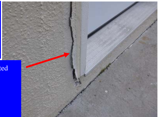
...its door sill is damaged...
