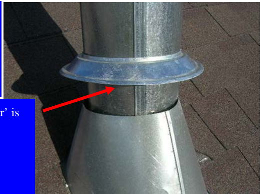
The water heater exhaust vent pipe is sealed to the rooftop flashing cone...
