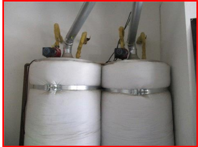
Water Heaters - Improper Seismic Strap Installation
