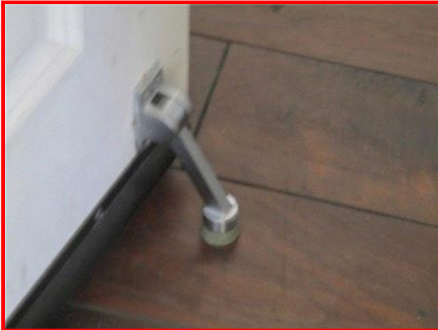
Improper Drop Down Stopper at Garage Door
