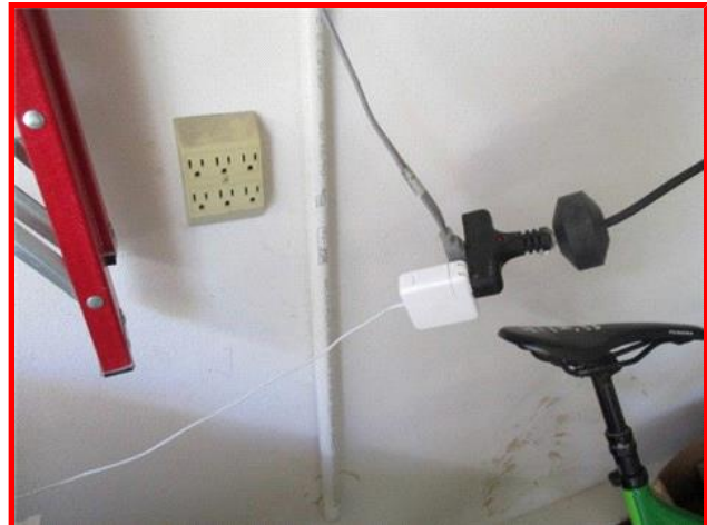
Improper Expander & Extension Cord in Garage
