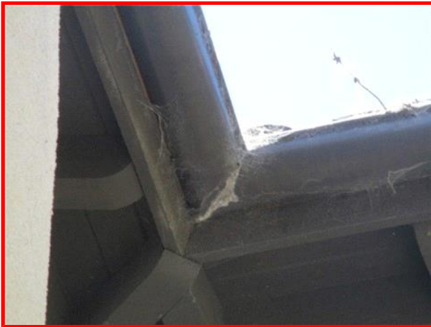
Leak at Atrium Gutter
