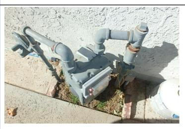
Item # 26 Automatic seismic shutoff valve is missing at the gas meter. \* (2) (4)
