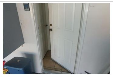
Item # 60 The garage fire door to interior is hollow core / not fire rated and has missing self-closer. \* (2) (4)
