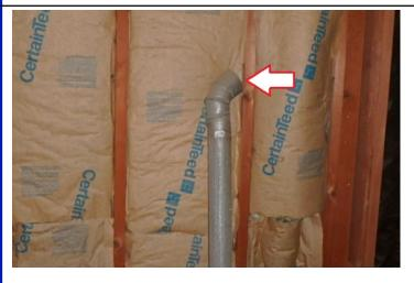
Item # 74 The ceiling exhaust fan duct terminates into the attic at bathroom D.
