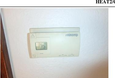
Item # 43 System A's thermostat control is operational, however is loose. \*
