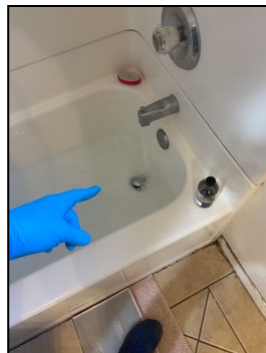
Drain operated slowly - needs to be serviced
