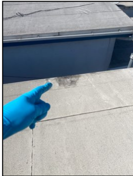
Materials appear to be nearing end of useful life - needs to be further evaluated by a licensed roofer
