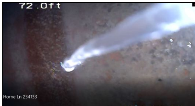
Believe to have reached main city sewer line at 72.0 feet
