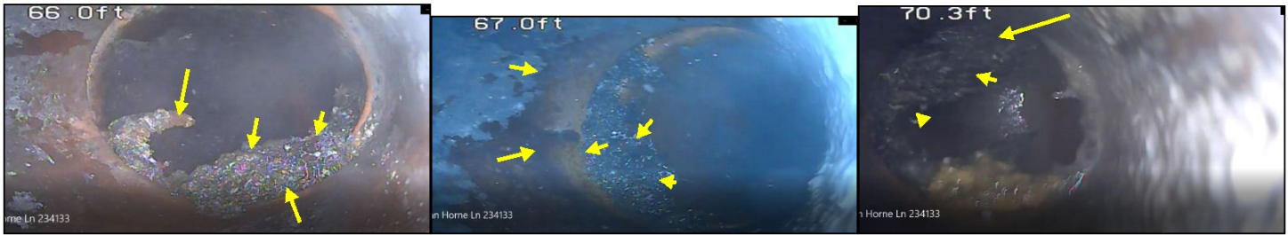
Root intrusion present at 66.0 feet Offset and root intrusion present at 67.0 feet Root intrusion present at 70.3 feet
