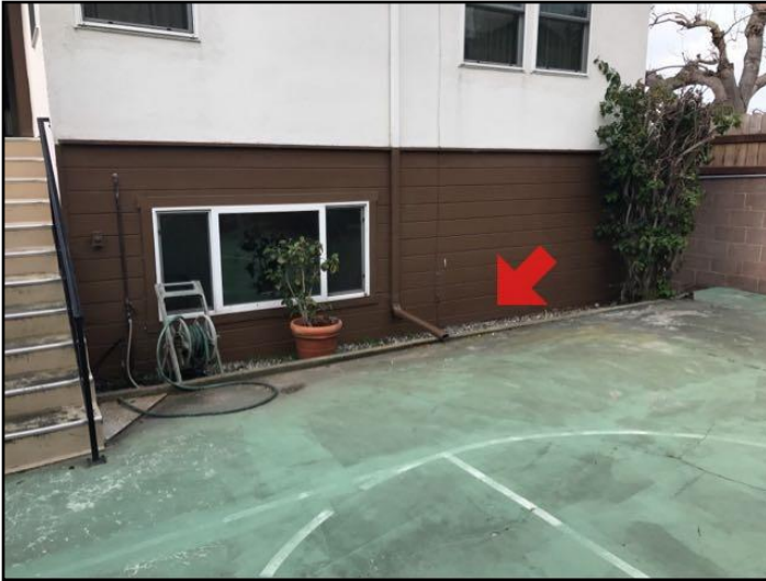
19. Improper slope or drainage
