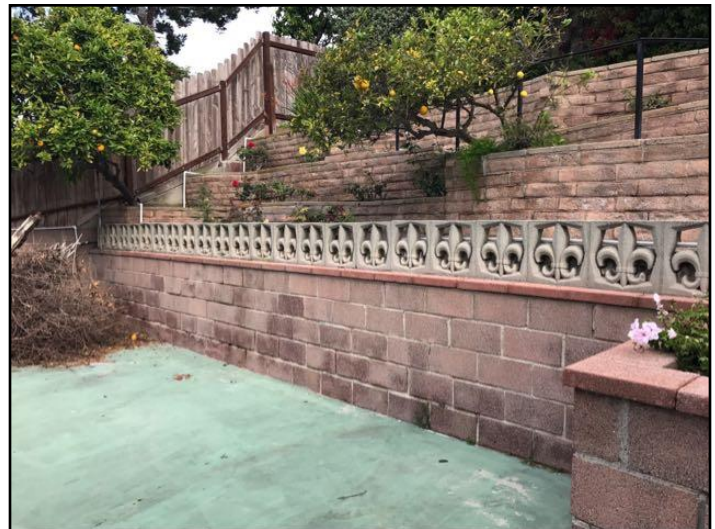
23. Drainage system missing
