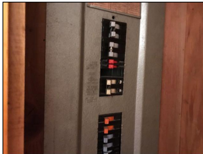
38. Unprotected openings
