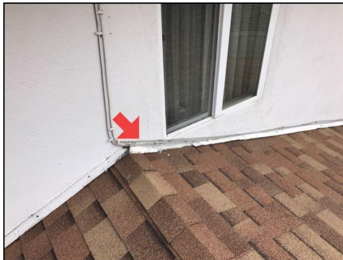
3. Damage, loose, open seams, patched
