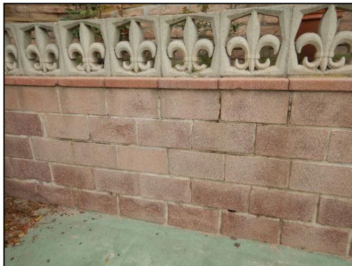
21. Mortar - deteriorated, missing
