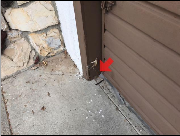
29. Water damage
