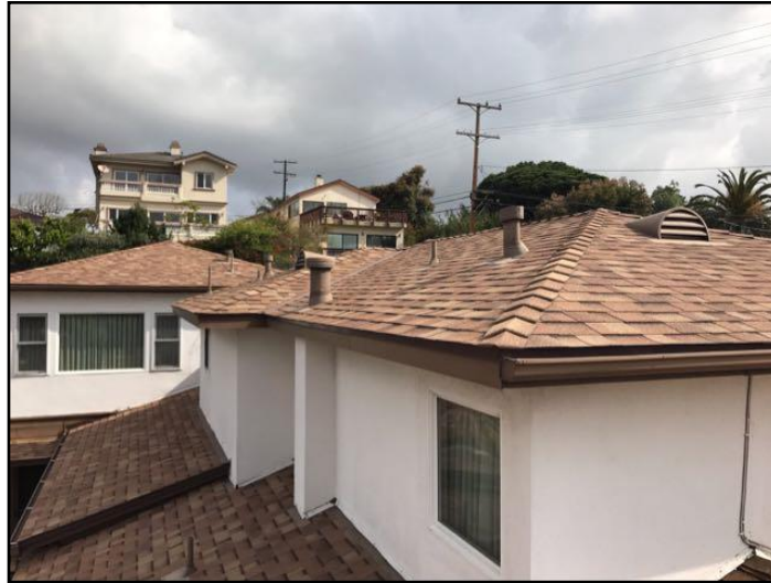
1. Asphalt shingles
