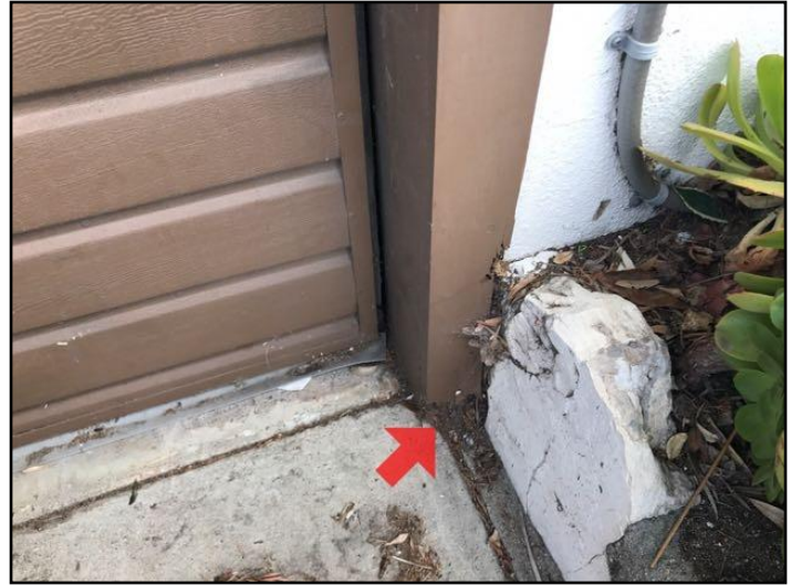
30. Water damage
