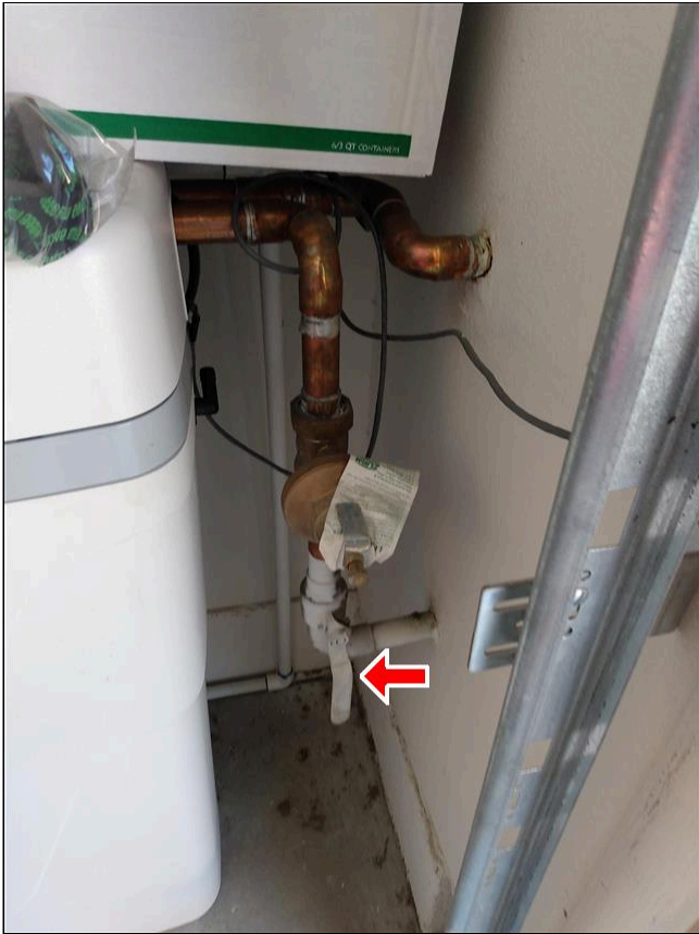
12.2 WATER SHUT-OFF VALVE (Picture 1)
