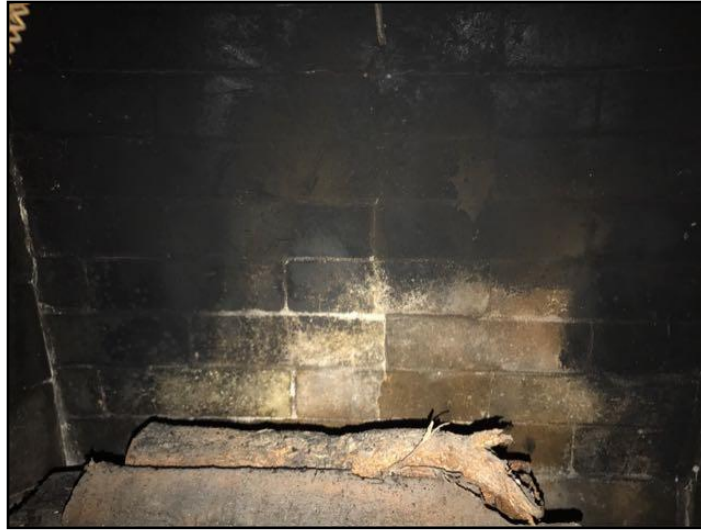
61. Cracked masonry or refractory
