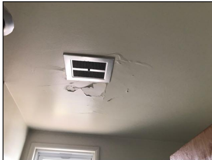
88. Water damage
