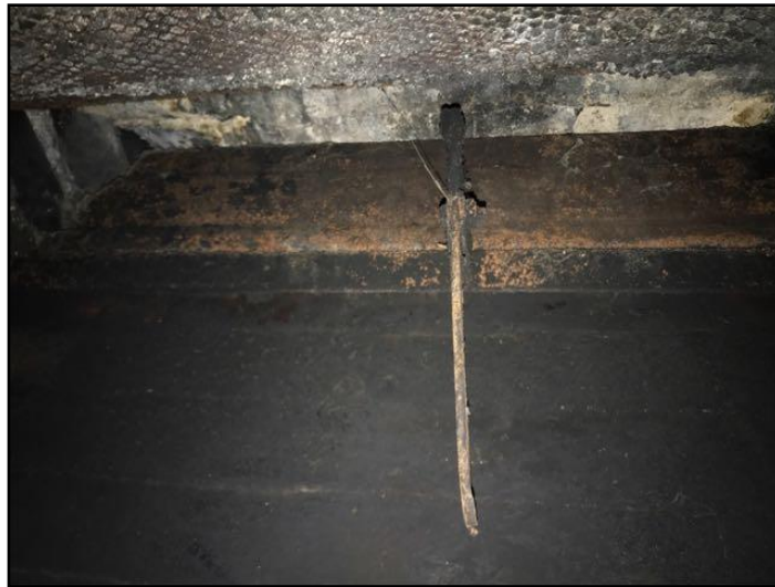
62. Damper or frame rusted
