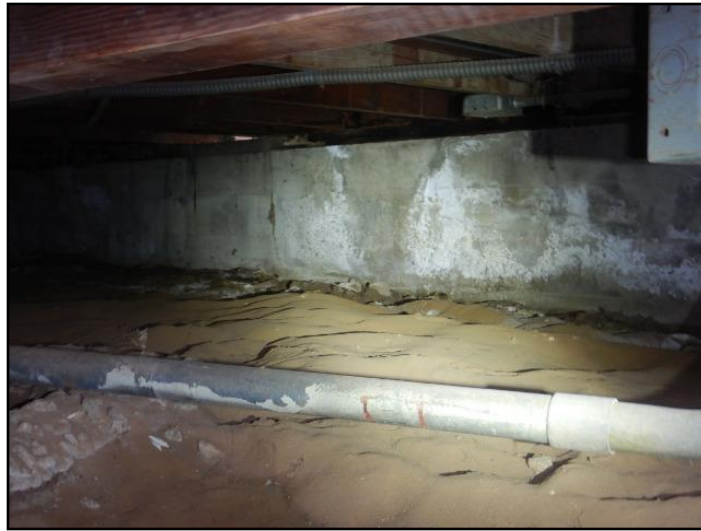
99. Dampness on floor or walls
