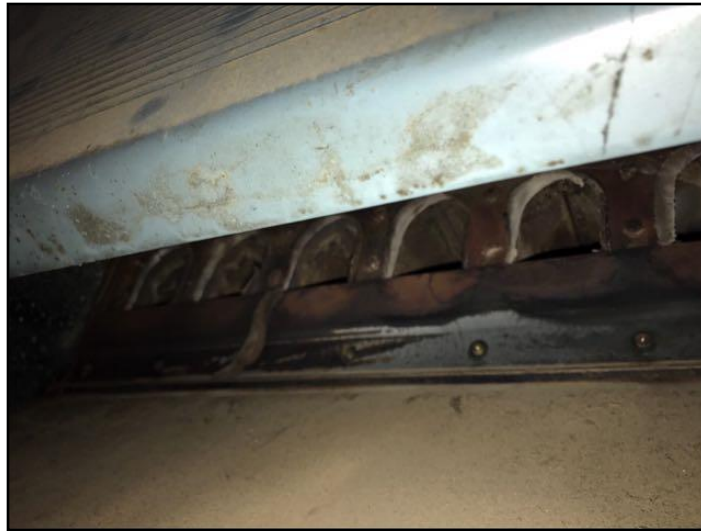
59. Draft hood spillage or backdraft
