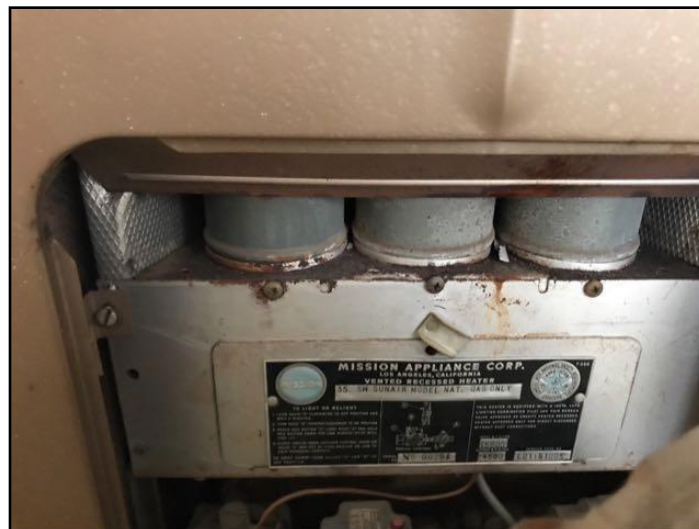
58. Draft hood spillage or backdraft
