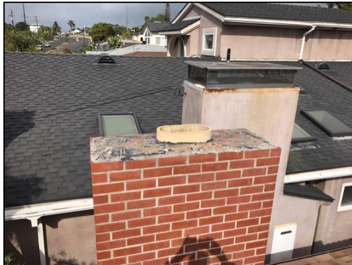
60. Screen missing or damaged
