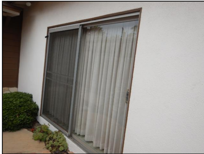
98. Safety glass not installed
