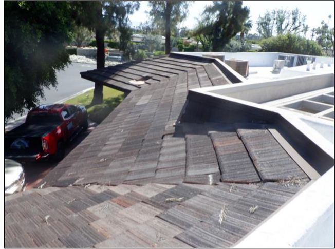
1.0 Item 8(Picture) Tile Roof Covering
