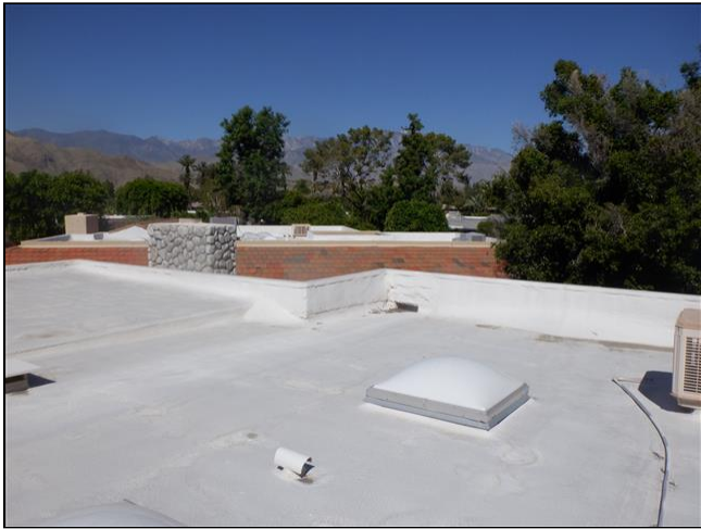
1.0 Item 18(Picture) Flat Roof Covering
