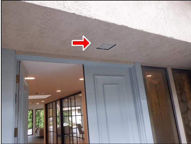
2.8 Item 1(Picture) Courtyard Light Fixture Not Functioning
