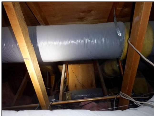
10.4.A Item 1(Picture) HVAC Ducting
