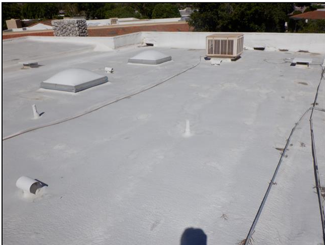
1.0 Item 14(Picture) Flat Roof Covering
