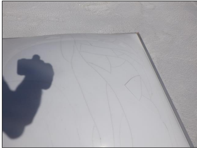
1.2 Item 7(Picture) Skylight 6 Cracked
