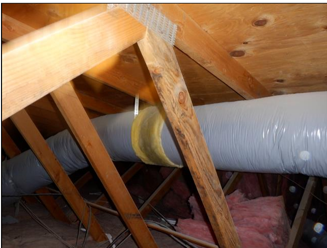
1.5 Item 5(Picture) Roof Framing/Roof Decking
