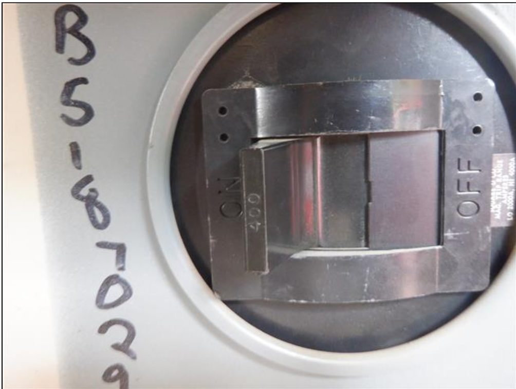
9.1 Item 5(Picture) Main Electrical Panel Disconnect 400 Amp
