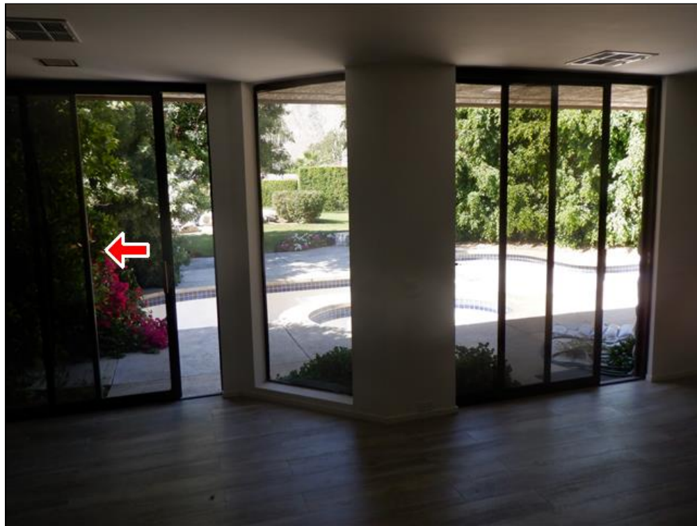
2.2 Item 1(Picture) Master Bedroom Slider Bad Seal
