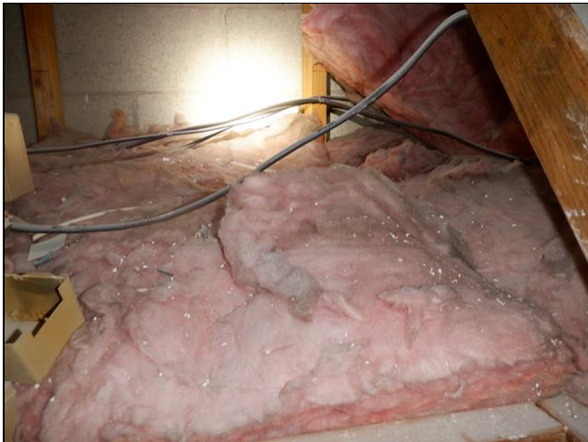
1.6 Item 5(Picture) Attic Insulation
