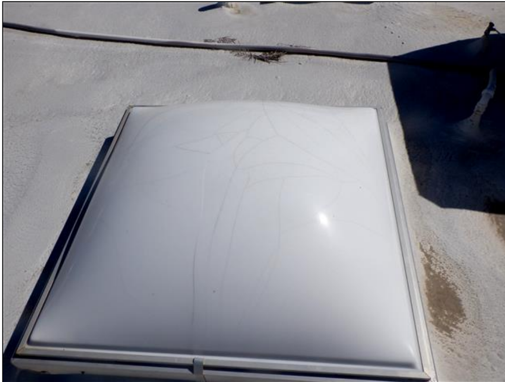
1.2 Item 6(Picture) Skylight 5 Cracked
