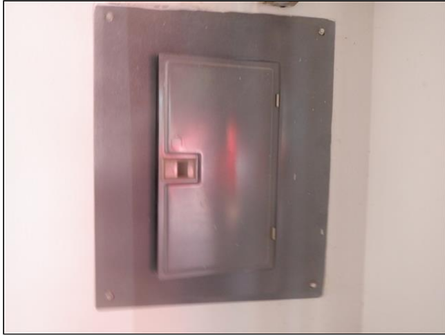
9.1 Item 6(Picture) Electrical Sub Panel
