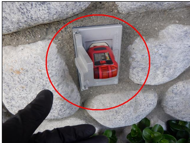
2.7 Item 7(Picture) West Patio Outlet No Power
