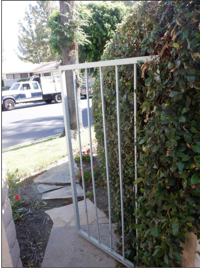
2.10 Item 1(Picture) Gate To Backyard
