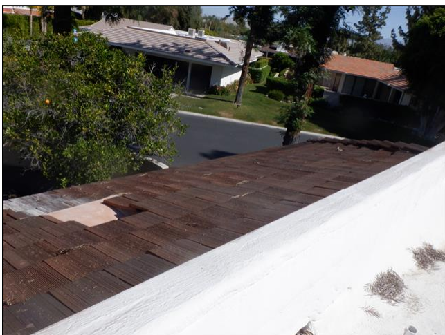
1.0 Item 5(Picture) Tile Roof Covering
