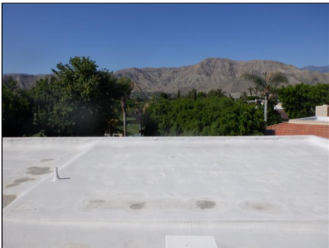
1.0 Item 20(Picture) Flat Roof Covering
