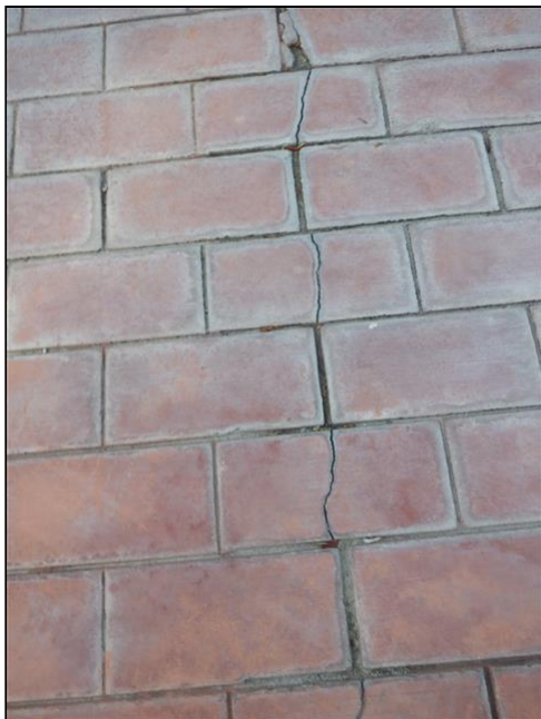
2.4 Item 5(Picture) Driveway Cracked Bricks
