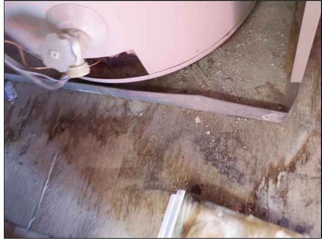
10.3.A Item 3(Picture) Moisture Stains Furnace Landing
