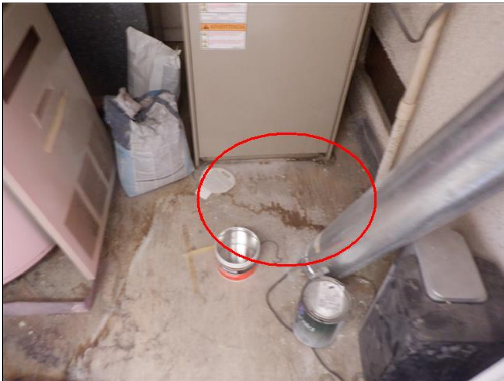
10.3.A Item 1(Picture) Moisture Stains Furnace Landing
