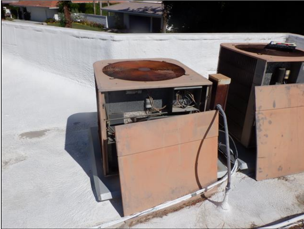
10.8.A Item 1(Picture) Cooling Units
