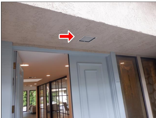
2.8 Item 1(Picture) Courtyard Light Fixture Not Functioning
