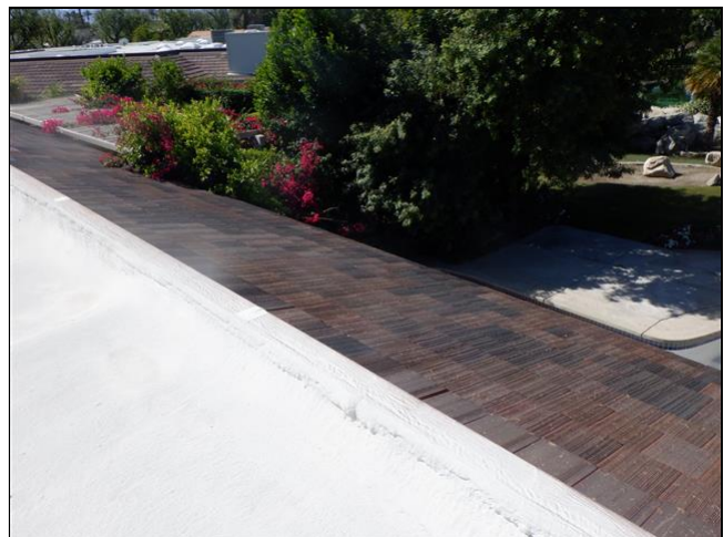
1.0 Item 4(Picture) Tile Roof Covering
