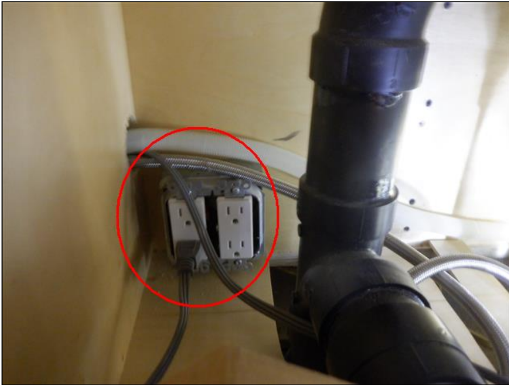
4.7 Item 1(Picture) Missing Outlet Cover Plate
