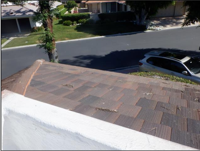
1.0 Item 7(Picture) Tile Roof Covering
