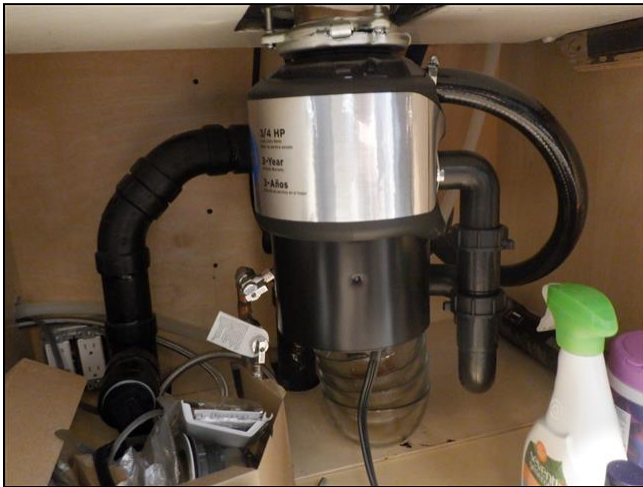
4.11 Item 1(Picture) Disposer No Activation Switch
