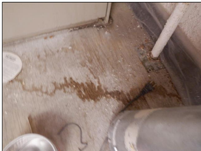
10.3.A Item 2(Picture) Moisture Stains Furnace Landing
