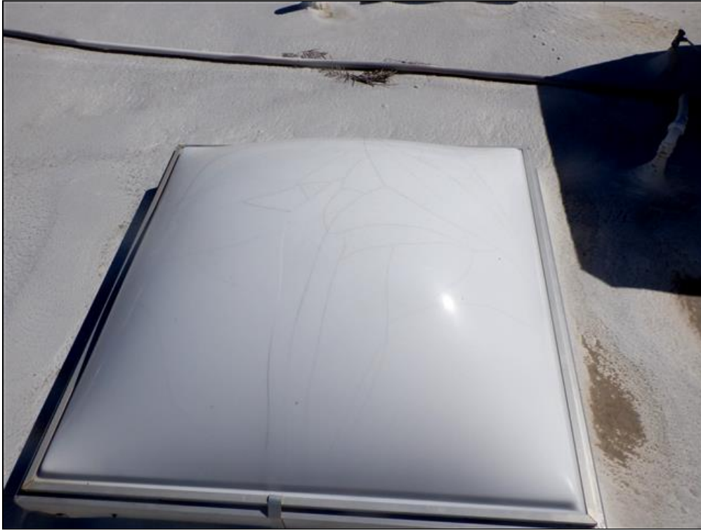
1.2 Item 6(Picture) Skylight 5 Cracked
