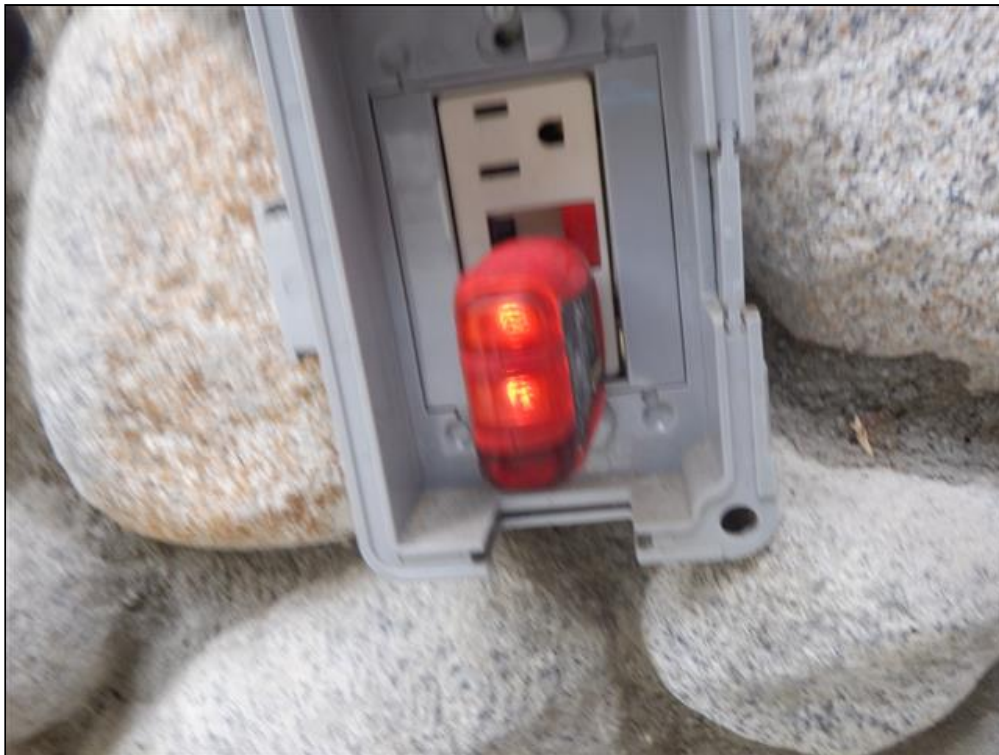
2.7 Item 2(Picture) GFCI Outlet Failed To Trip
