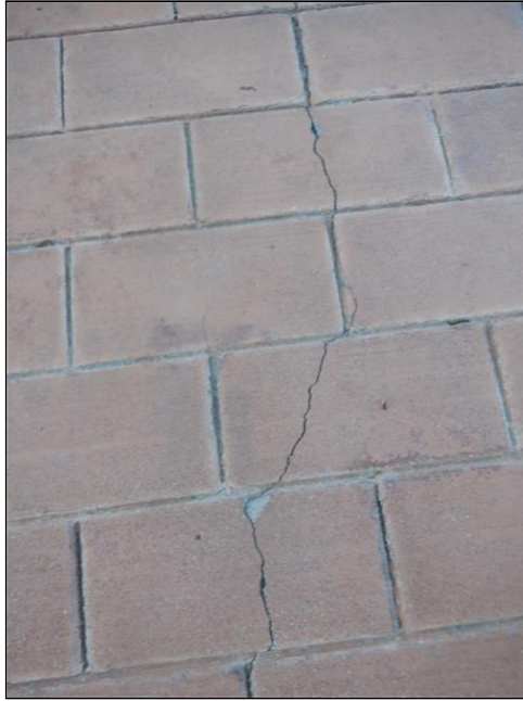
2.4 Item 4(Picture) Driveway Cracked Bricks
