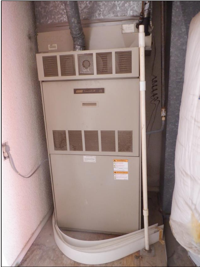
10.0.A Item 1(Picture) Heating Unit 1
