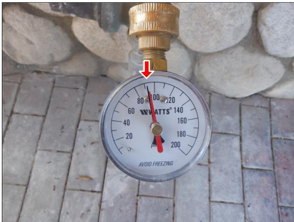
8.5 Item 1(Picture) Water Pressure 92 psi
