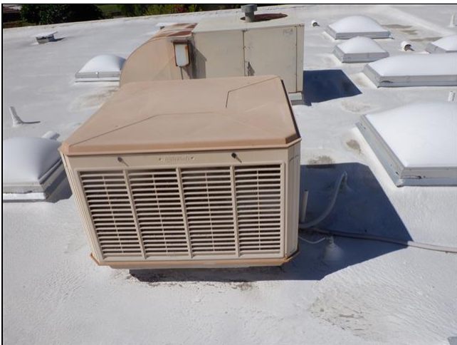
10.4.B Item 1(Picture) Evaporative Cooler 1
