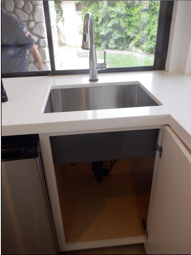
4.15 Item 1(Picture) Bar Sink Faucet
