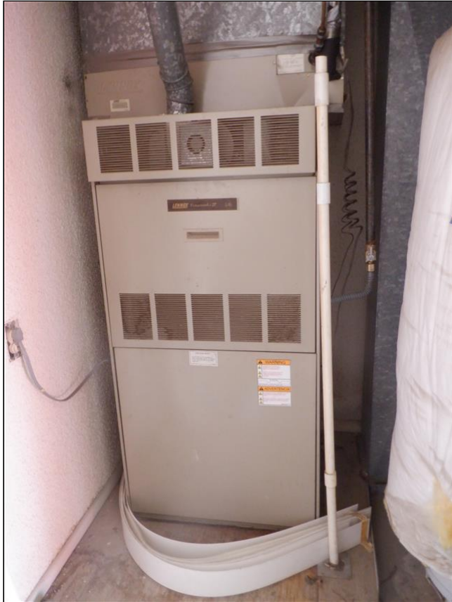
10.0.A Item 1(Picture) Heating Unit 1
