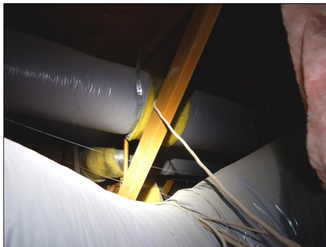
10.4.A Item 2(Picture) HVAC Ducting
