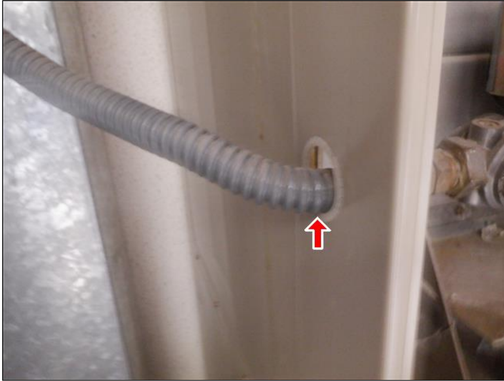
10.0.A Item 6(Picture) Heating Unit 2 Flex Fuel Line
