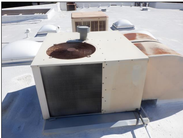
10.0.B Item 1(Picture) Heating Unit 1 Flex Fuel Line
