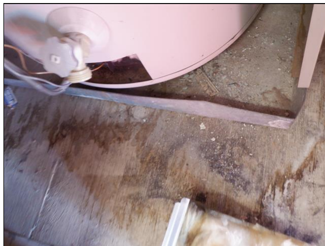
10.3.A Item 3(Picture) Moisture Stains Furnace Landing
