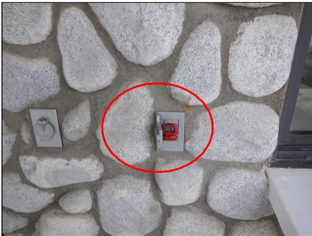
2.7 Item 5(Picture) North Patio Outlet No Power
