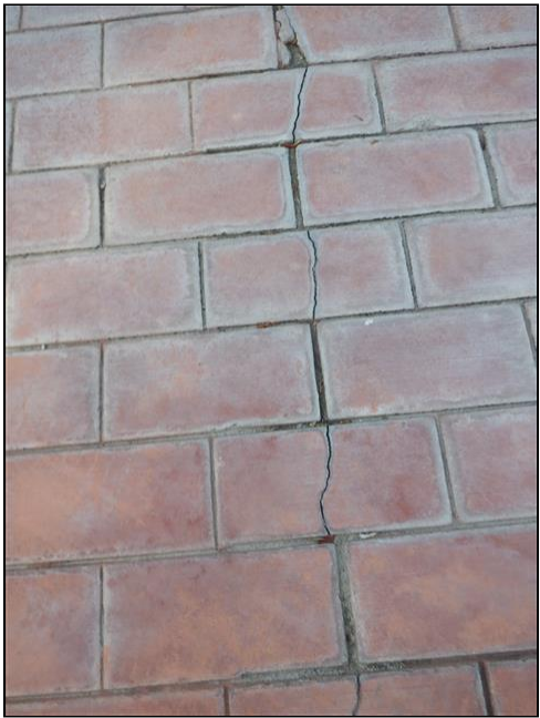
2.4 Item 5(Picture) Driveway Cracked Bricks
