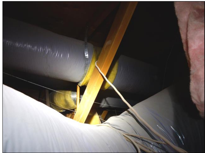
10.4.A Item 2(Picture) HVAC Ducting
