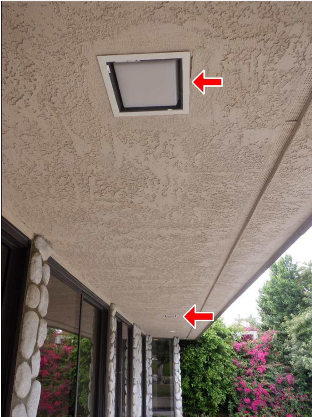
2.8 Item 2(Picture) Patio Light Fixtures Not Functioning
