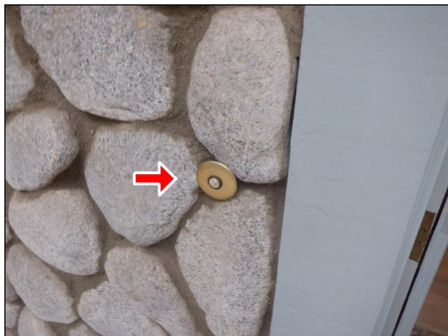
2.9 Item 1(Picture) Door Bell Not Functioning
