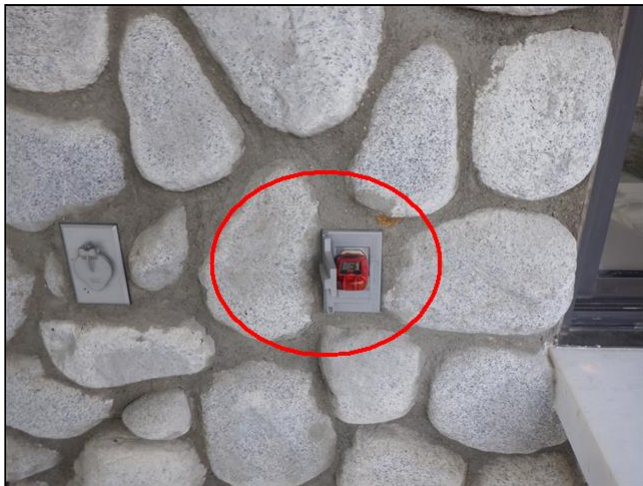
2.7 Item 5(Picture) North Patio Outlet No Power
