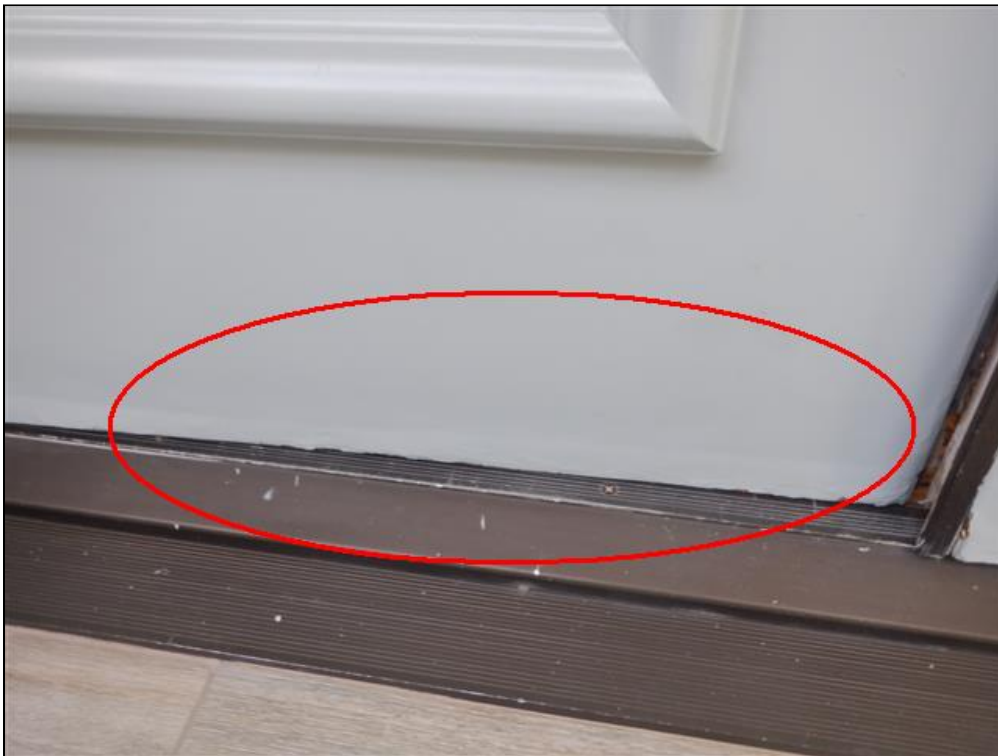
2.1 Item 3(Picture) Front Doors Weathered
