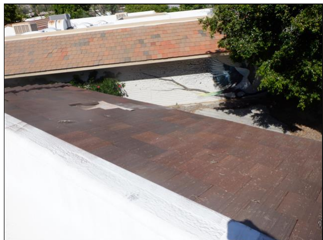
1.0 Item 6(Picture) Tile Roof Covering
