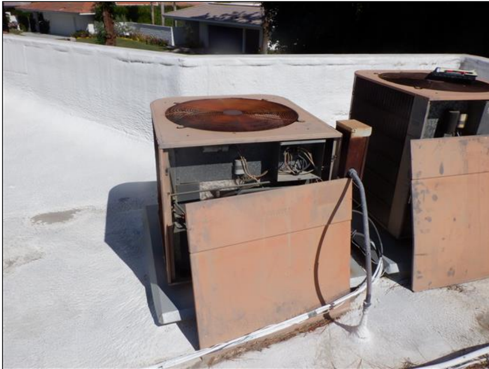
10.8.A Item 1(Picture) Cooling Units
