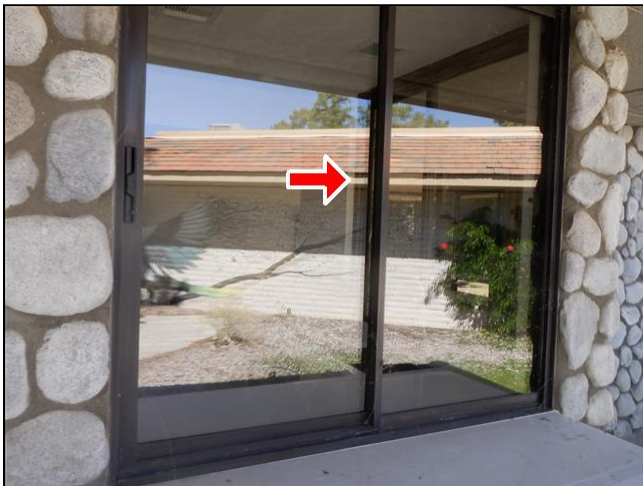
2.2 Item 4(Picture) Bar Window Inoperative
