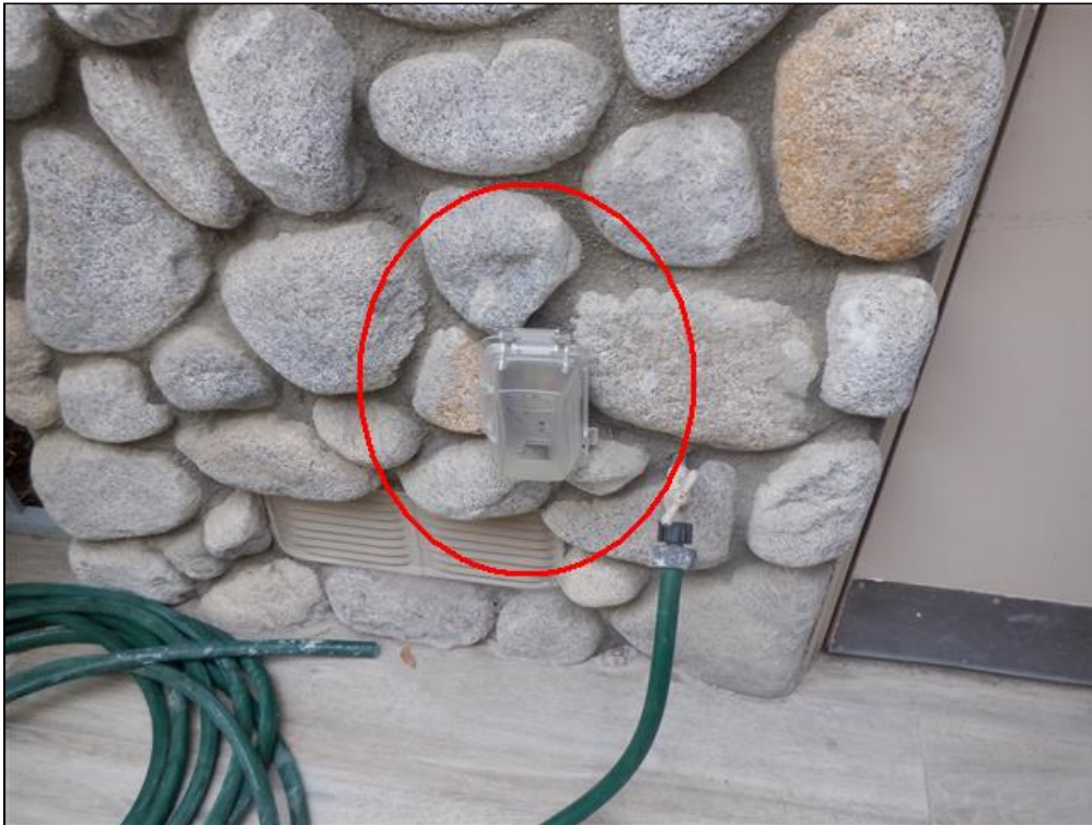
2.7 Item 1(Picture) GFCI Outlet Failed To Trip
