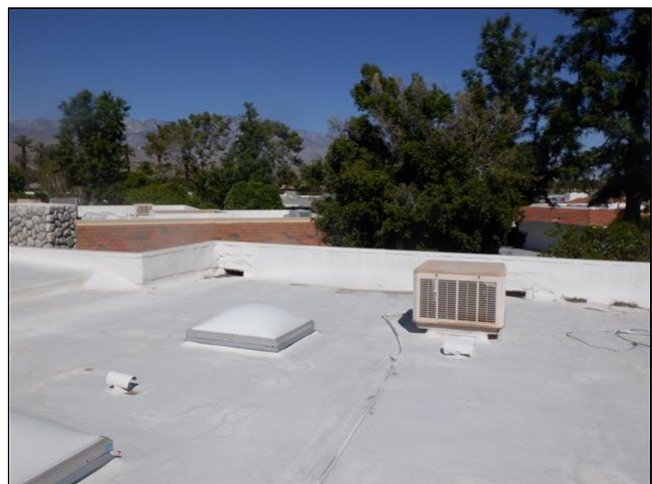
1.0 Item 17(Picture) Flat Roof Covering
