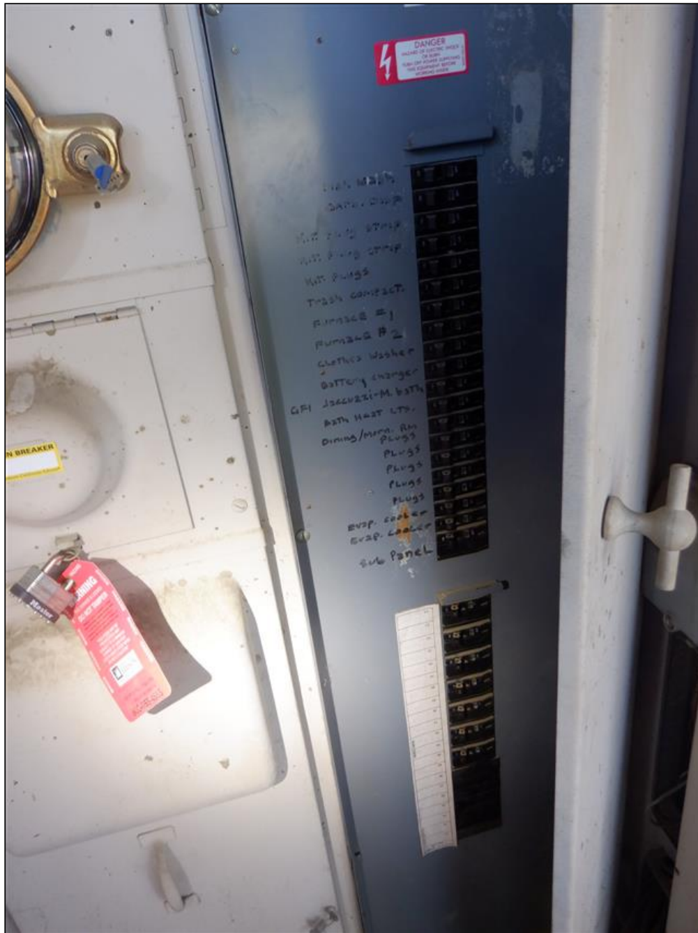
9.1 Item 2(Picture) Main Electrical Panel Distribution
