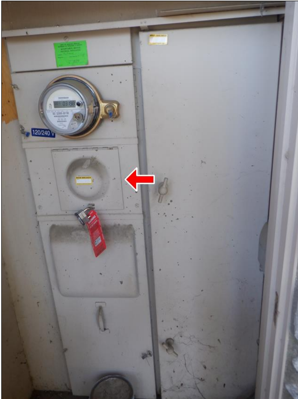
9.1 Item 1(Picture) Main Electrical Panel Disconnect 400 Amp
