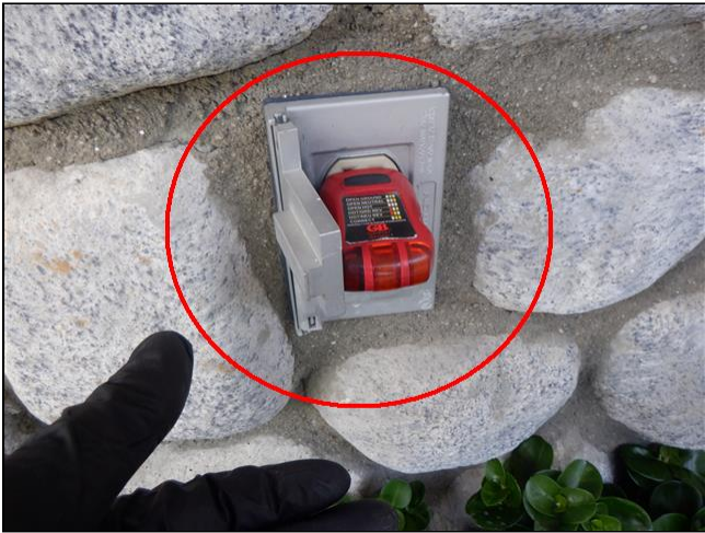
2.7 Item 7(Picture) West Patio Outlet No Power
