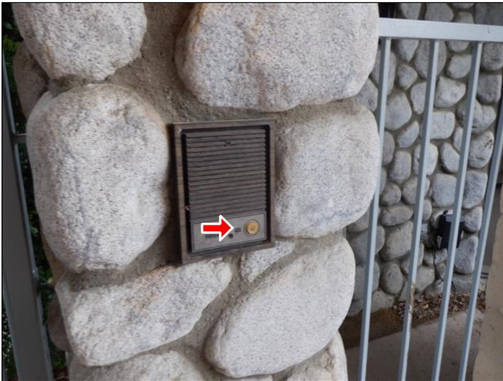
2.9 Item 2(Picture) Door Bell Not Functioning
