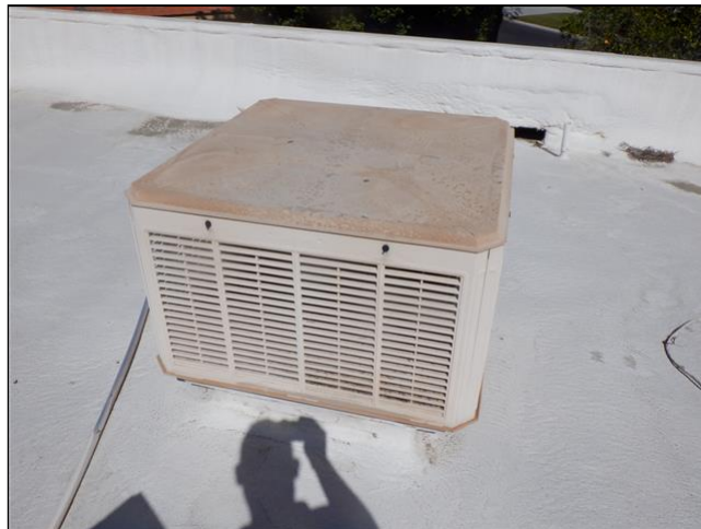
10.4.B Item 2(Picture) Evaporative Cooler 2
