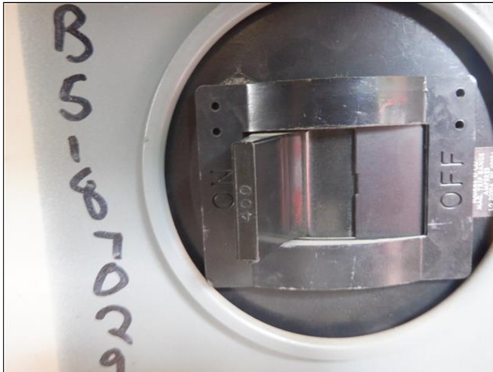
9.1 Item 5(Picture) Main Electrical Panel Disconnect 400 Amp
