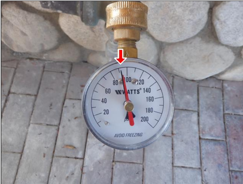
8.5 Item 1(Picture) Water Pressure 92 psi
