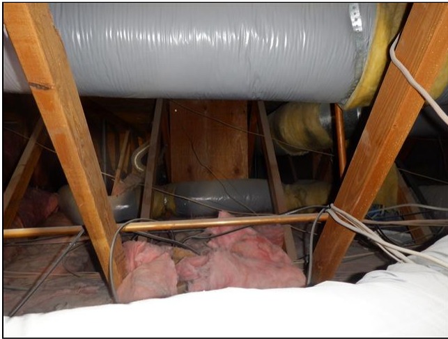
1.6 Item 1(Picture) Attic Insulation
