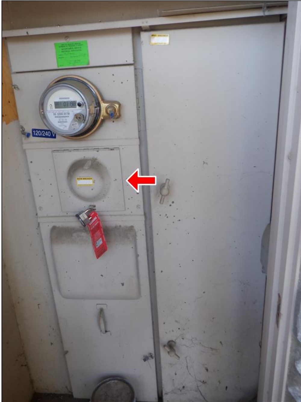
9.1 Item 1(Picture) Main Electrical Panel Disconnect 400 Amp
