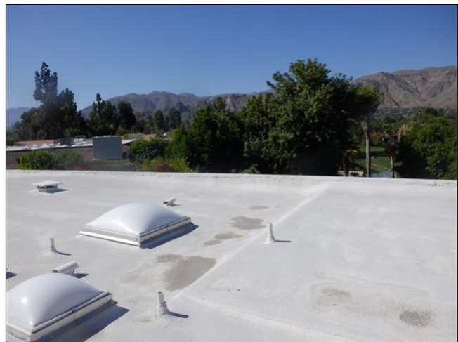
1.0 Item 21(Picture) Flat Roof Covering
