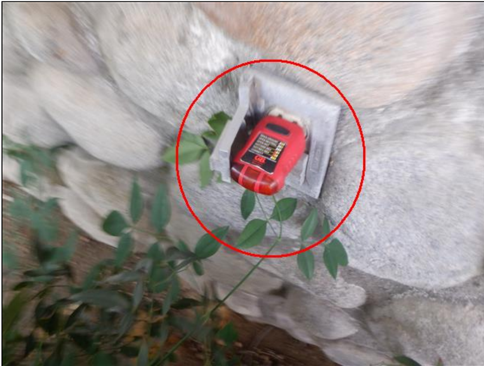
2.7 Item 4(Picture) North Patio Outlet No Power
