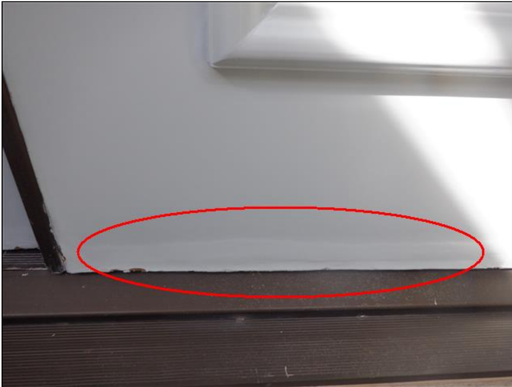
2.1 Item 2(Picture) Front Doors Weathered
