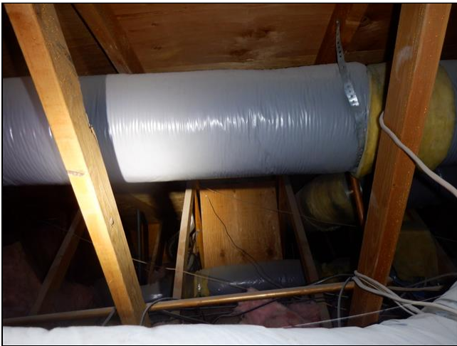
10.4.A Item 1(Picture) HVAC Ducting
