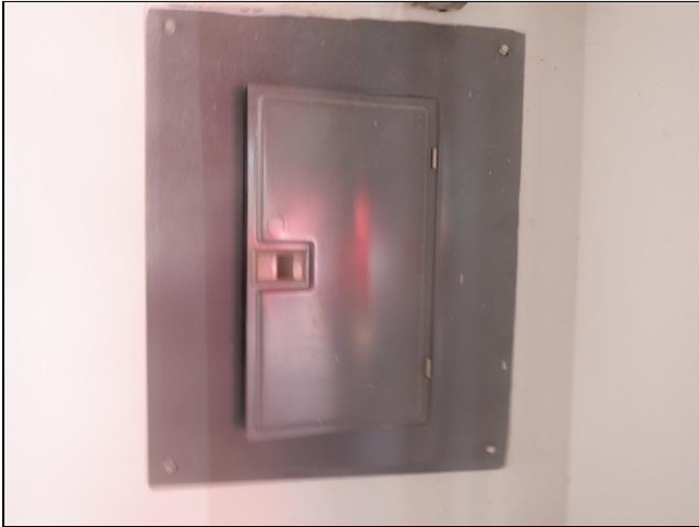
9.1 Item 6(Picture) Electrical Sub Panel
