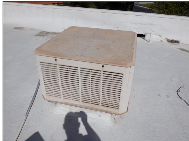
10.4.B Item 2(Picture) Evaporative Cooler 2
