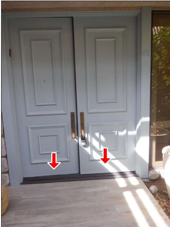
2.1 Item 1(Picture) Front Doors Weathered
