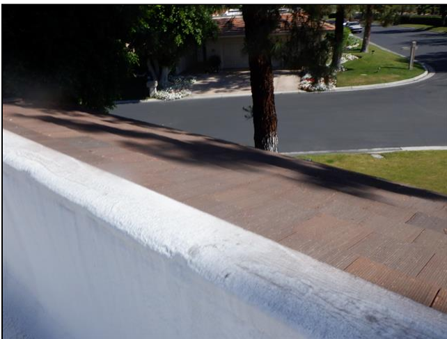
1.0 Item 11(Picture) Tile Roof Covering
