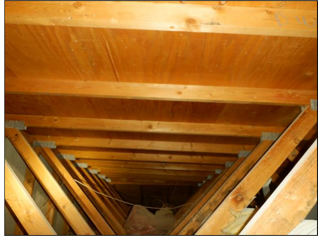
1.5 Item 2(Picture) Roof Framing/Roof Decking
