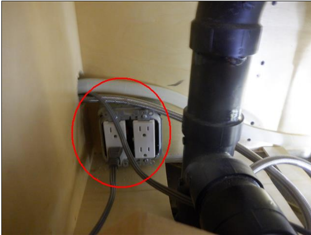
4.7 Item 1(Picture) Missing Outlet Cover Plate
