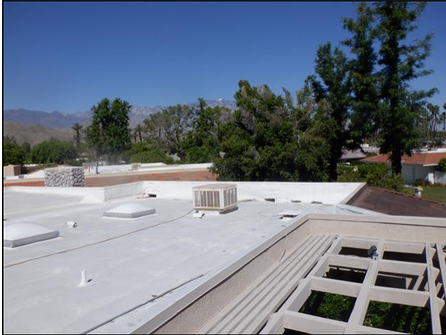
1.0 Item 12(Picture) Flat Roof Covering
