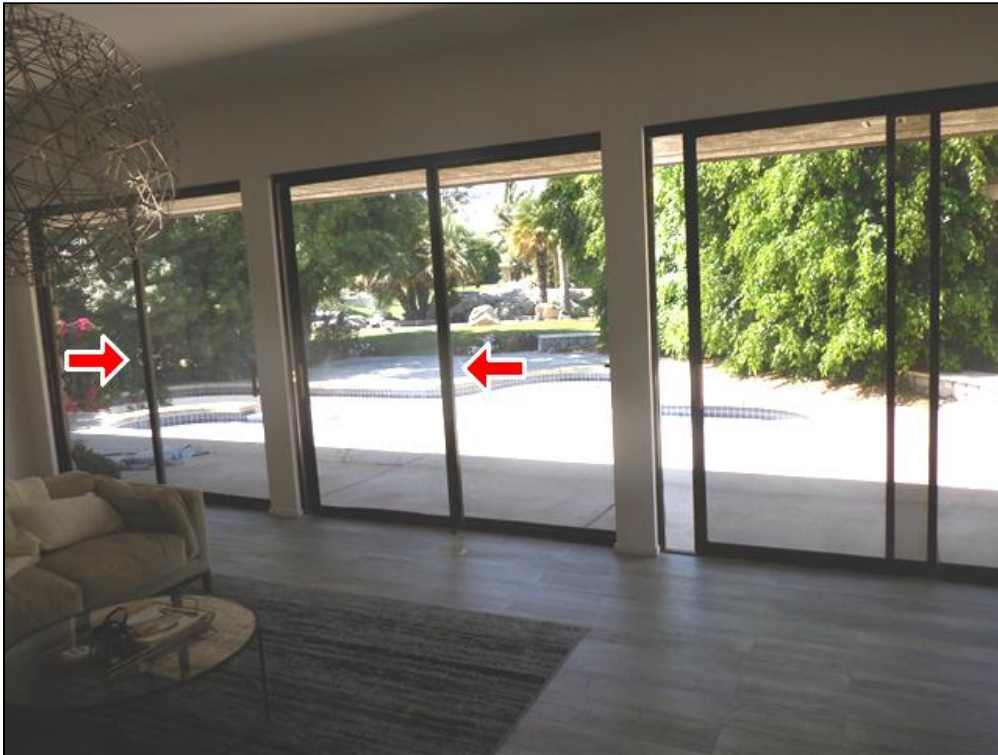
2.2 Item 3(Picture) Living Room Sliders Hard To Operate/Inoperable
