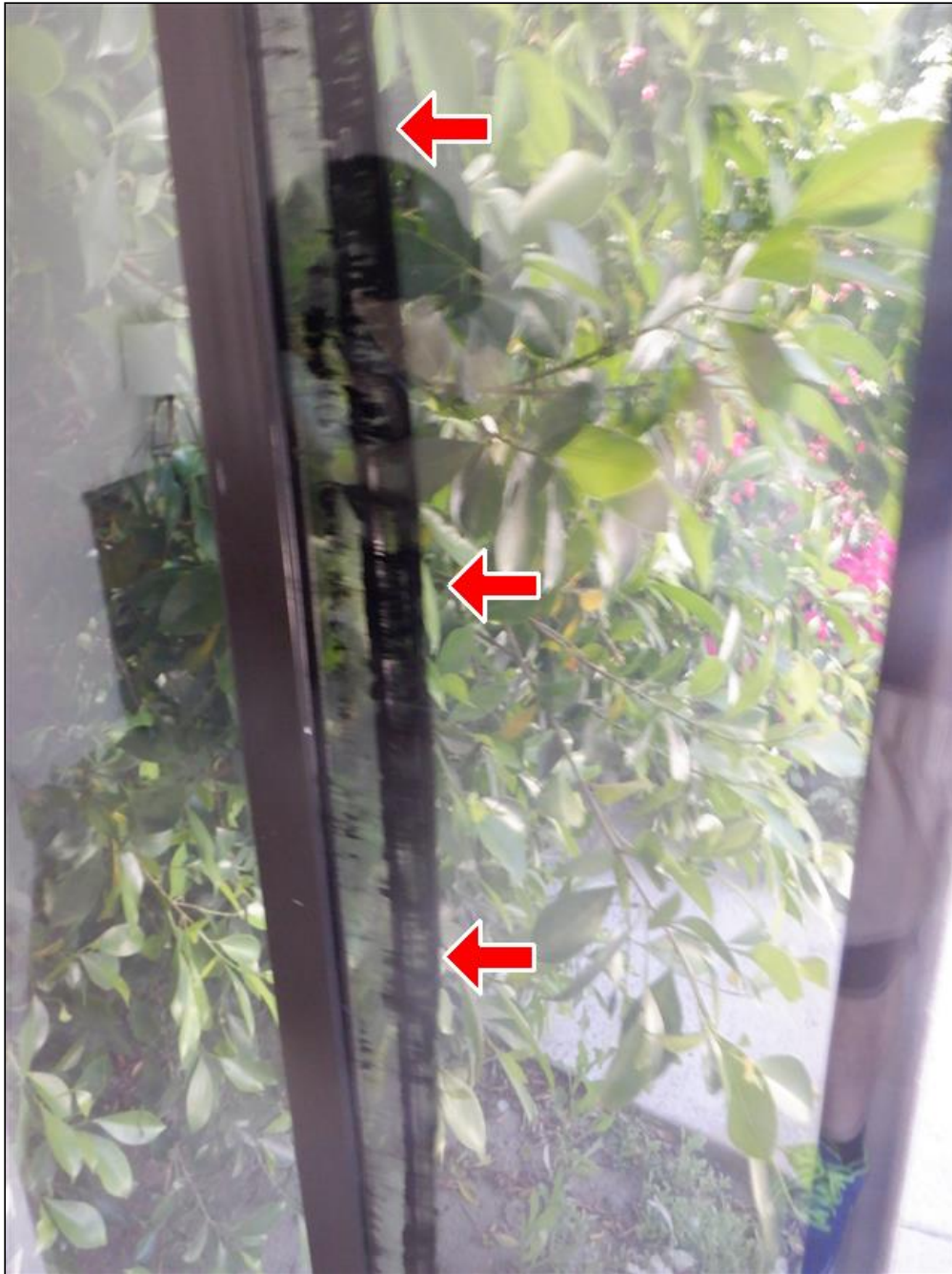
2.2 Item 2(Picture) Master Bedroom Slider Bad Seal
