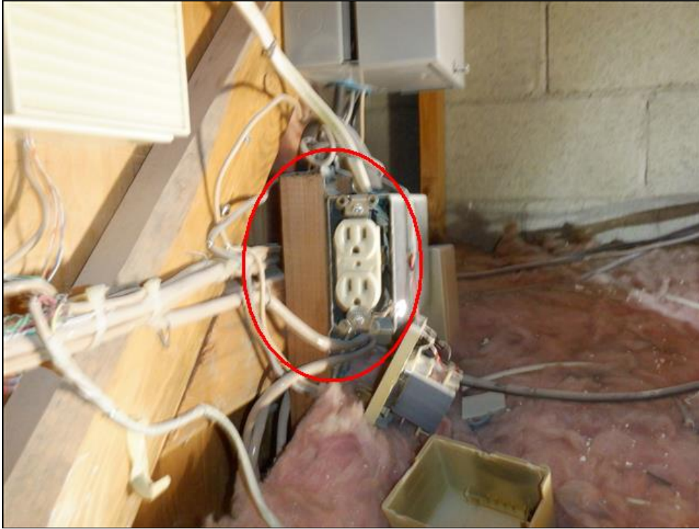
1.7 Item 1(Picture) Attic Electrical Outlet Missing Cover Plate
