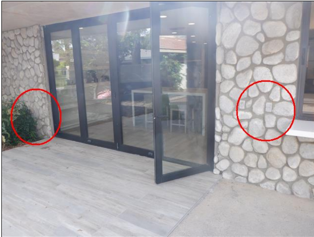
2.7 Item 3(Picture) North Patio Outlet No Power
