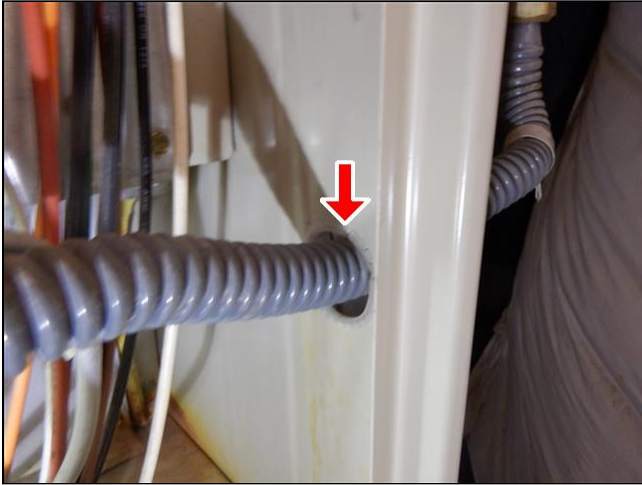
10.0.A Item 3(Picture) Heating Unit 1 Flex Fuel Line
