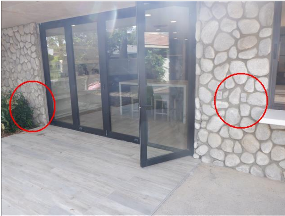
2.7 Item 3(Picture) North Patio Outlet No Power
