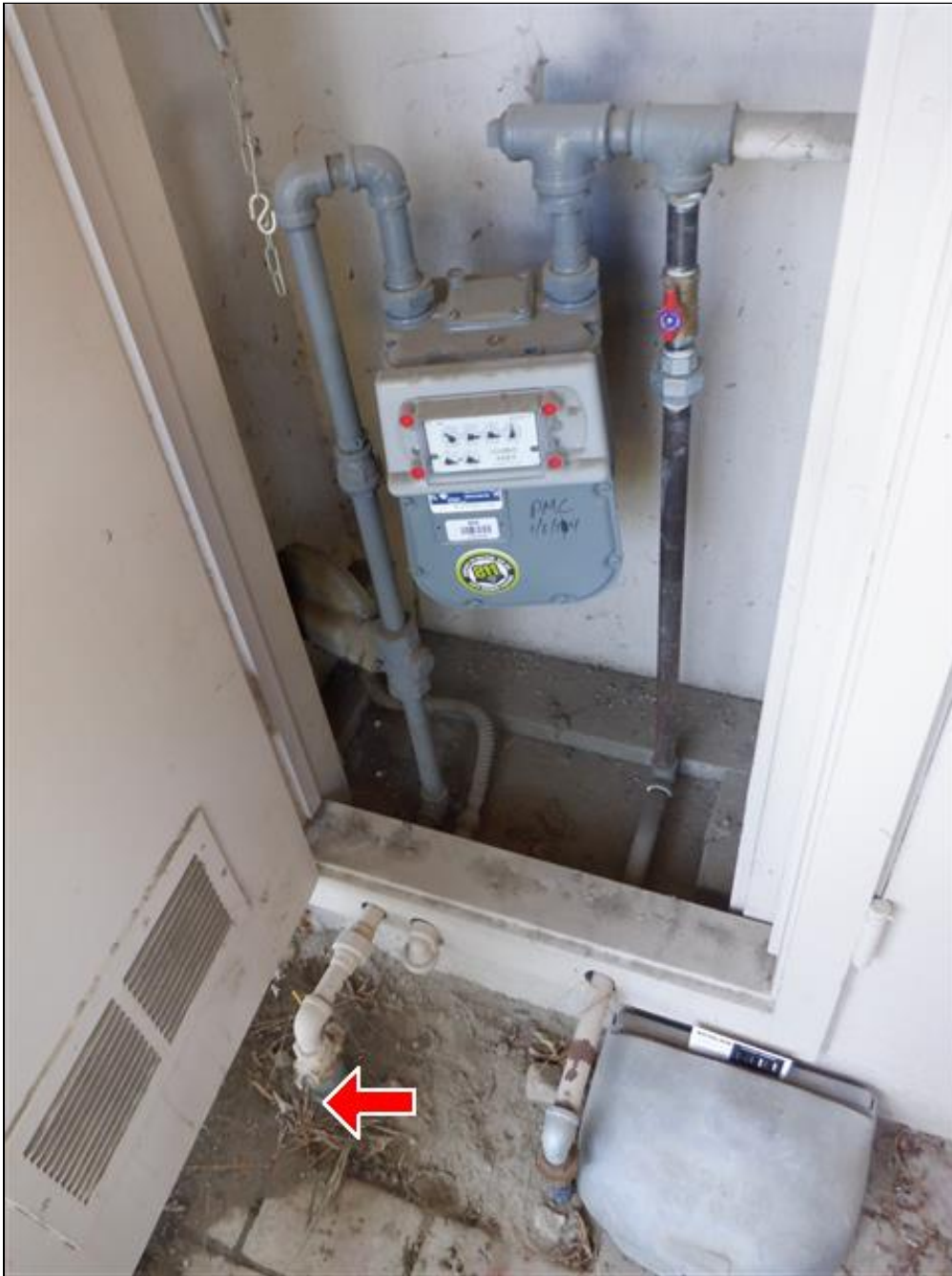
8.6 Item 1(Picture) Main Gas Shut Off
