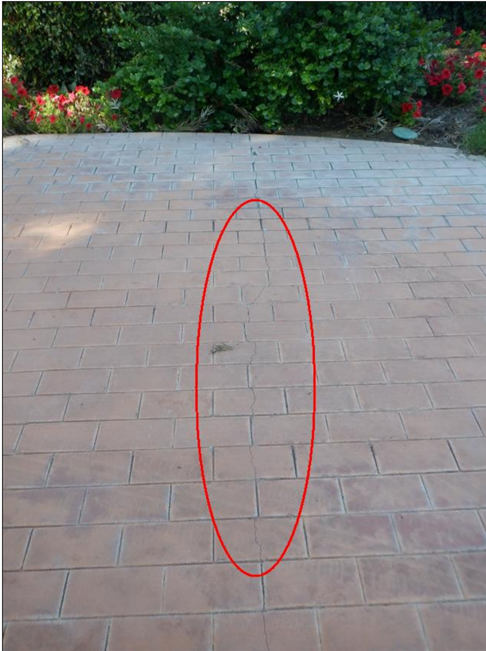
2.4 Item 2(Picture) Driveway Cracked Bricks
