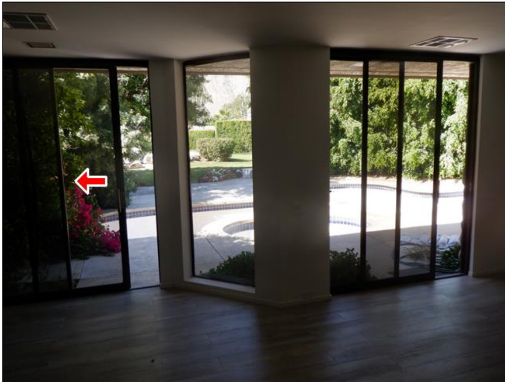
2.2 Item 1(Picture) Master Bedroom Slider Bad Seal
