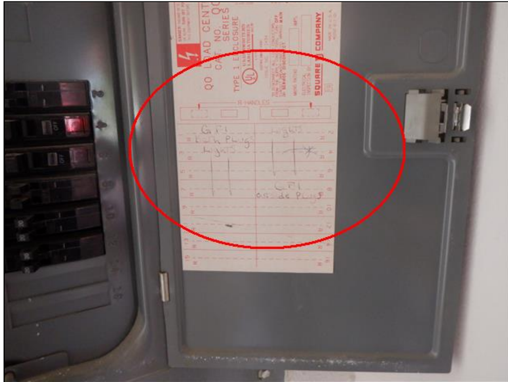
9.1 Item 7(Picture) Electrical Sub Panel Breakers Not Clearly Labeled
