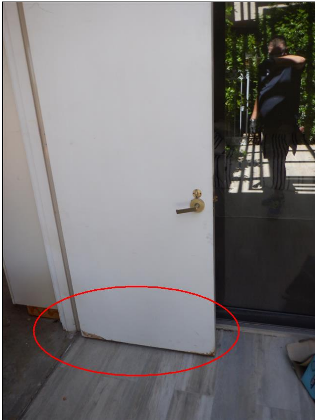
3.7 Item 1(Picture) Garage Man Door Stained/Weathered
