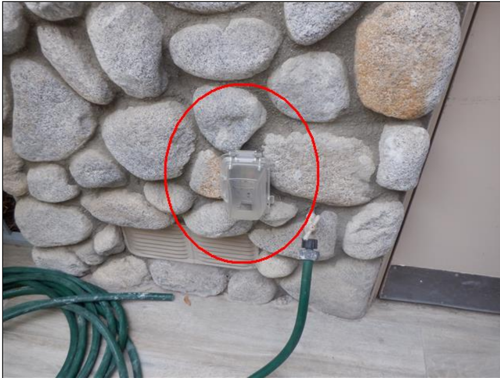
2.7 Item 1(Picture) GFCI Outlet Failed To Trip
