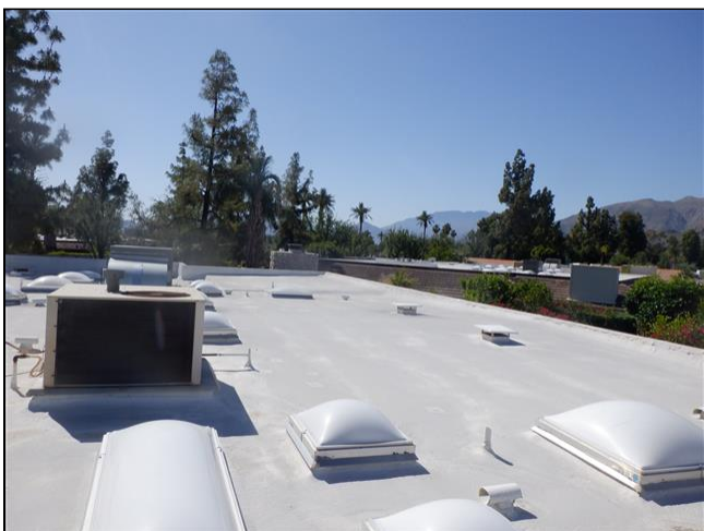
1.0 Item 22(Picture) Flat Roof Covering
