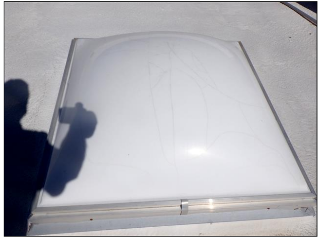
1.2 Item 8(Picture) Skylight 7 Cracked
