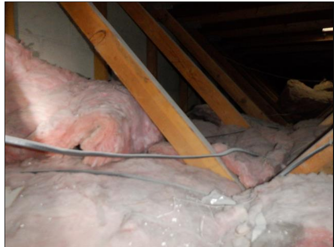
1.6 Item 6(Picture) Attic Insulation
