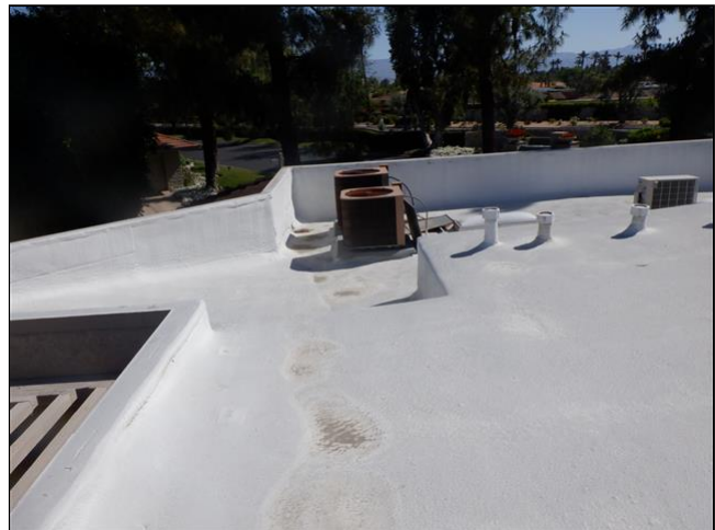
1.0 Item 15(Picture) Flat Roof Covering
