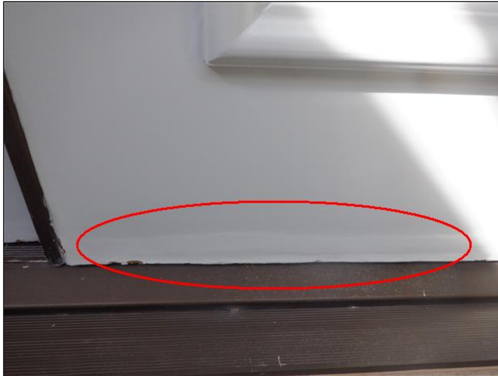
2.1 Item 2(Picture) Front Doors Weathered
