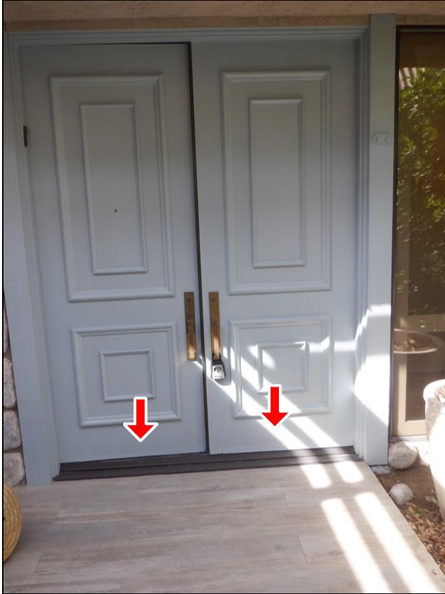
2.1 Item 1(Picture) Front Doors Weathered
