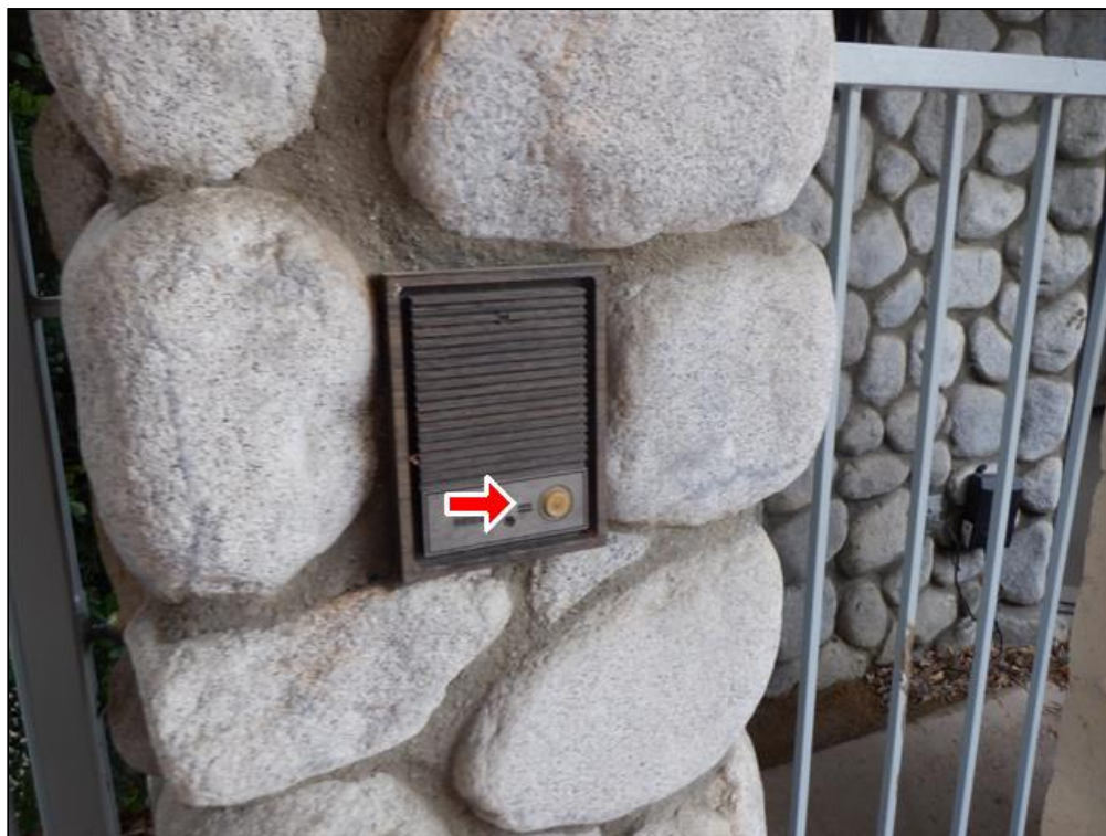
2.9 Item 2(Picture) Door Bell Not Functioning
