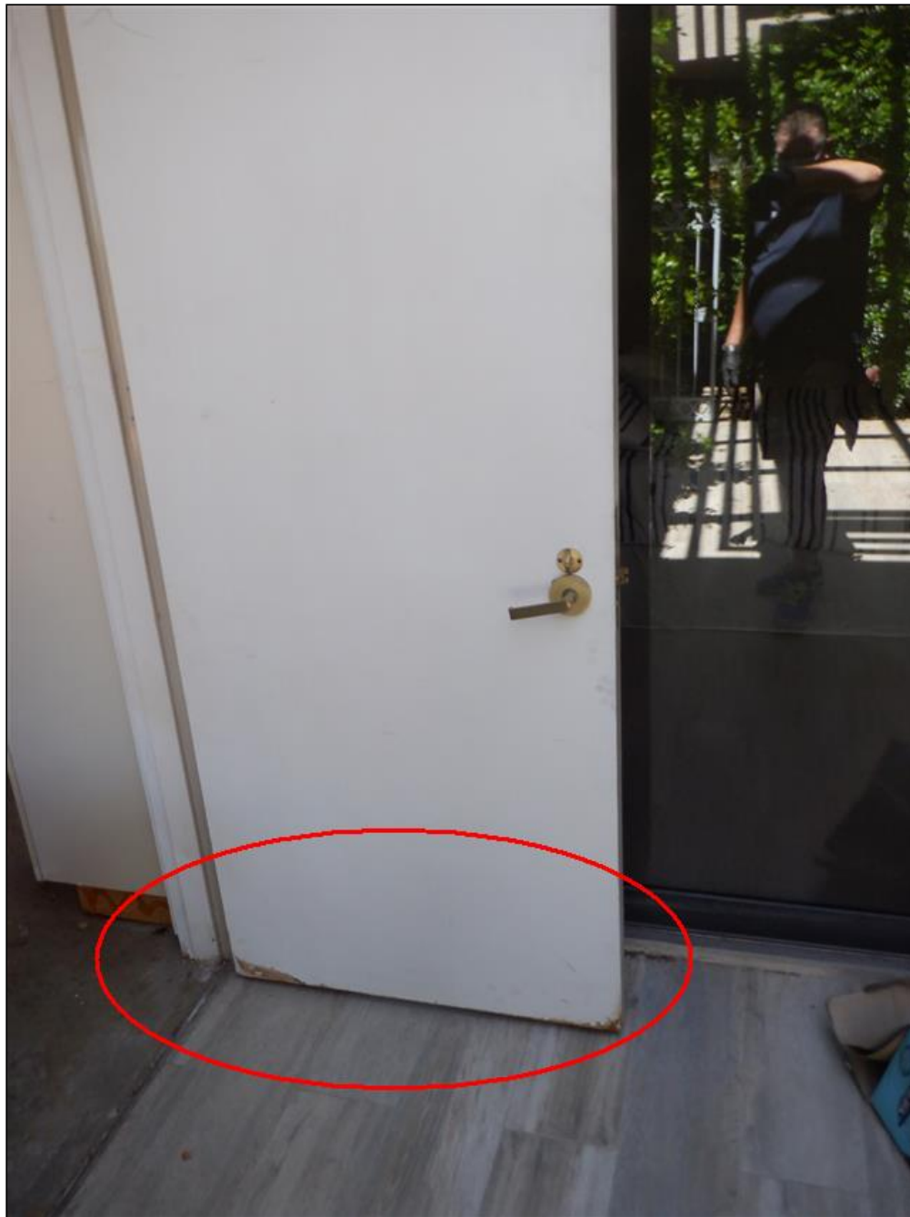
3.7 Item 1(Picture) Garage Man Door Stained/Weathered
