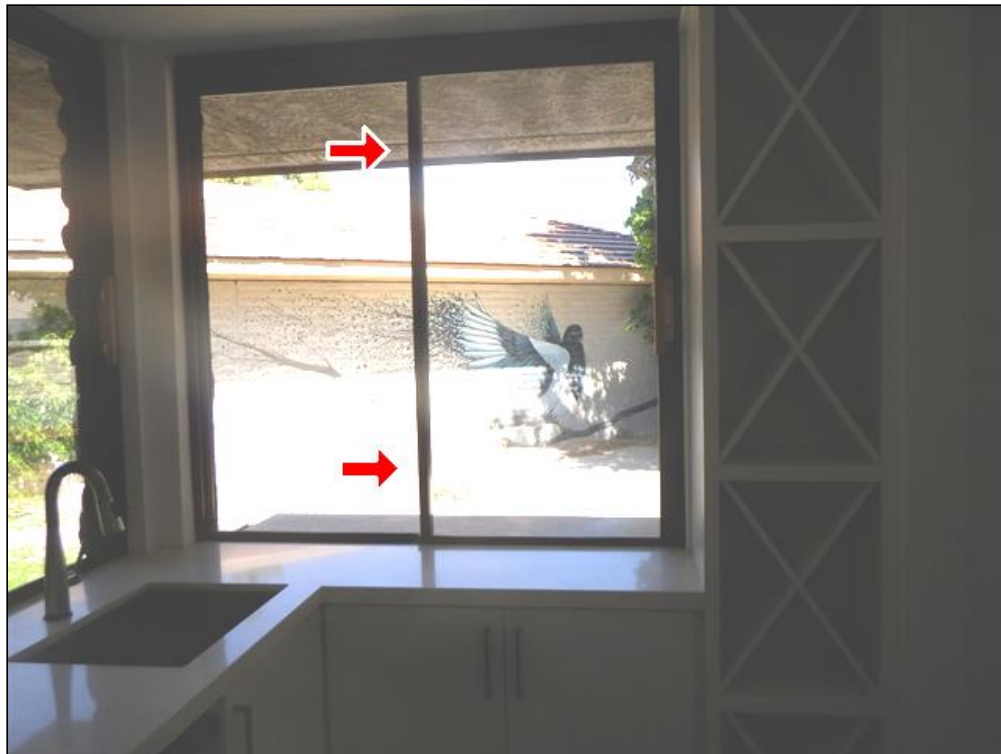
2.2 Item 5(Picture) Bar Window Inoperative
