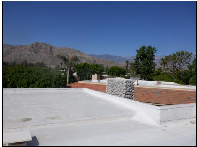
1.0 Item 19(Picture) Flat Roof Covering
