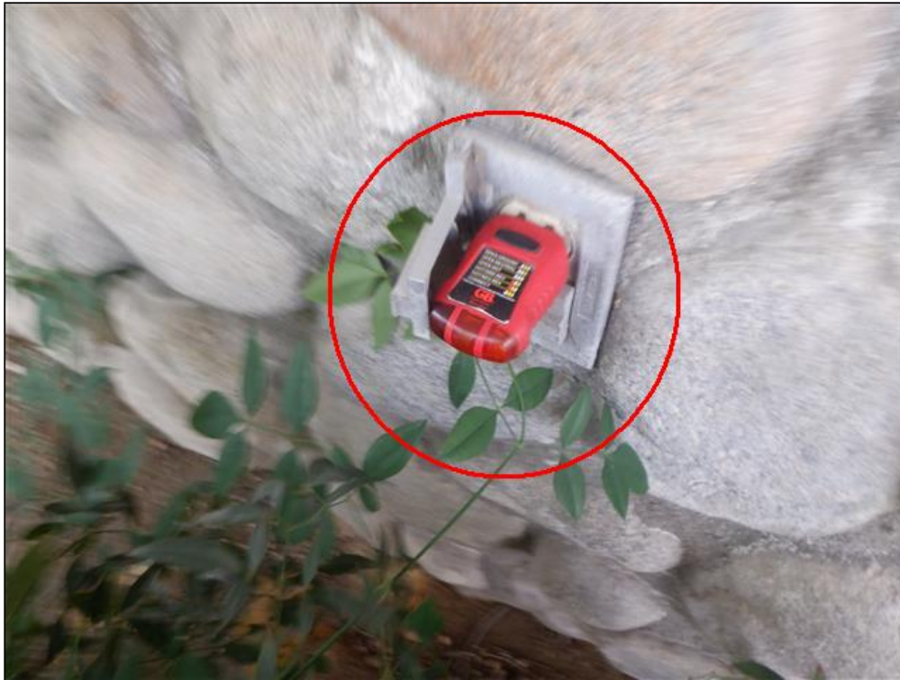
2.7 Item 4(Picture) North Patio Outlet No Power
