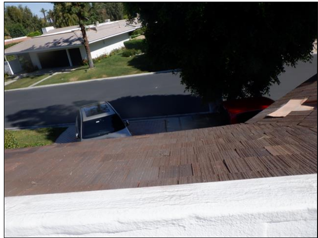
1.0 Item 10(Picture) Tile Roof Covering
