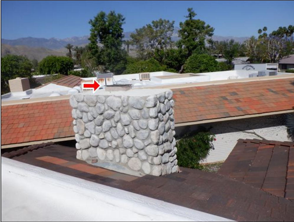
1.2 Item 1(Picture) Chimney Missing Rain Cap
