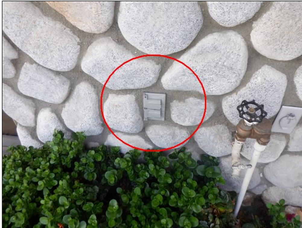
2.7 Item 6(Picture) West Patio Outlet No Power
