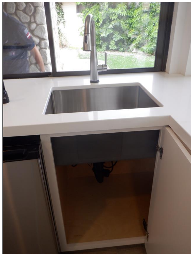
4.15 Item 1(Picture) Bar Sink Faucet
