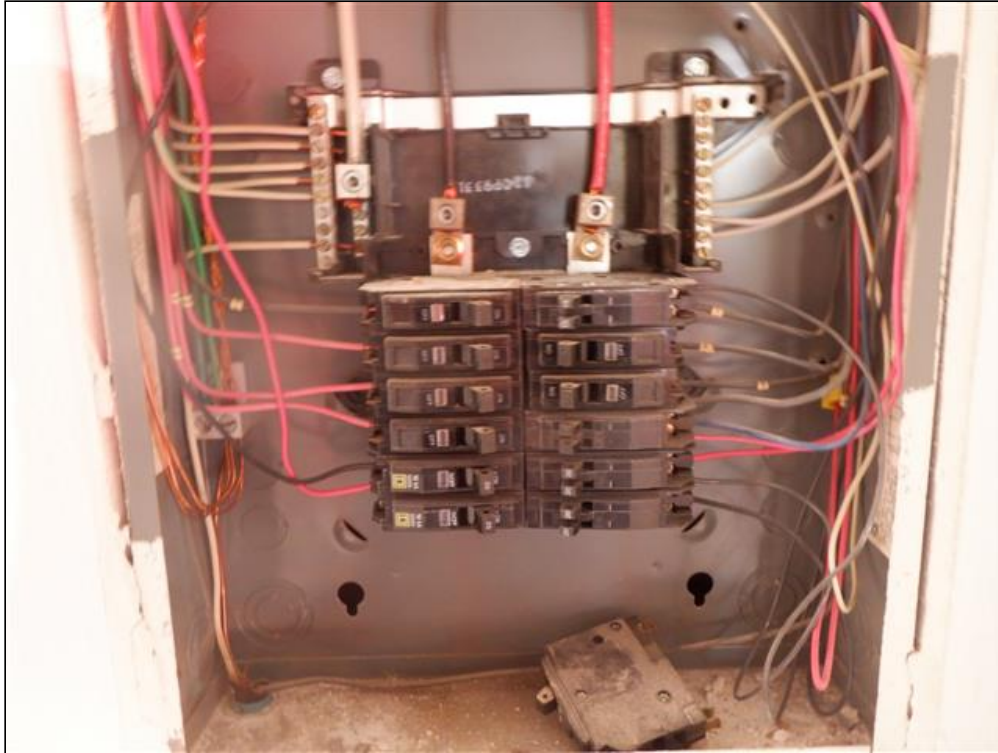
9.1 Item 9(Picture) Electrical Sub Panel Breakers/Conductors
