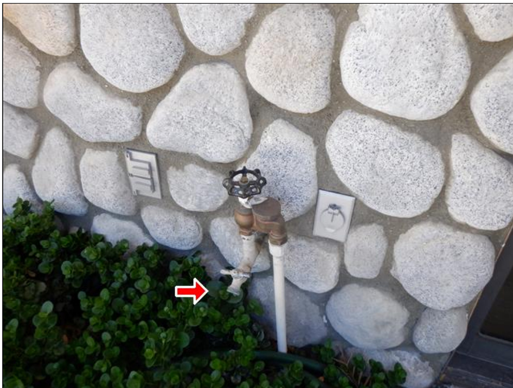
2.6 Item 1(Picture) Hose Bib Leak
