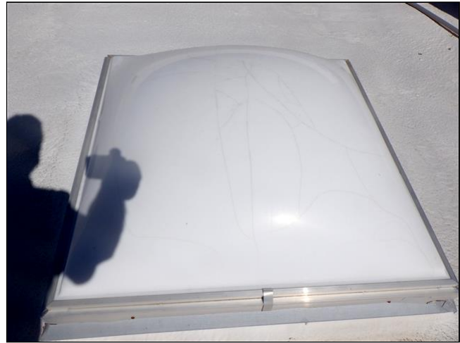
1.2 Item 8(Picture) Skylight 7 Cracked
