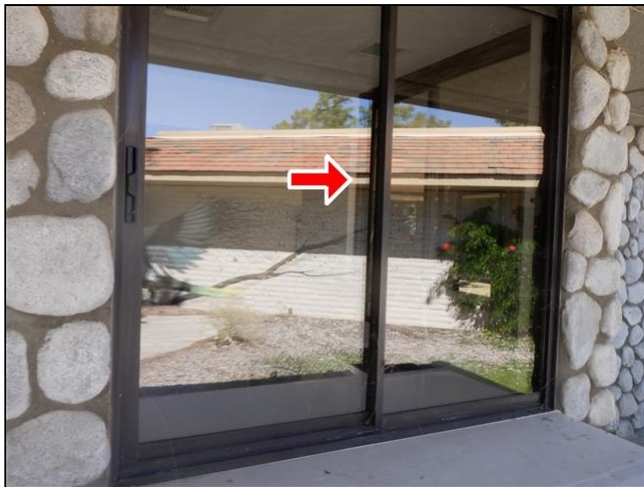
2.2 Item 4(Picture) Bar Window Inoperative
