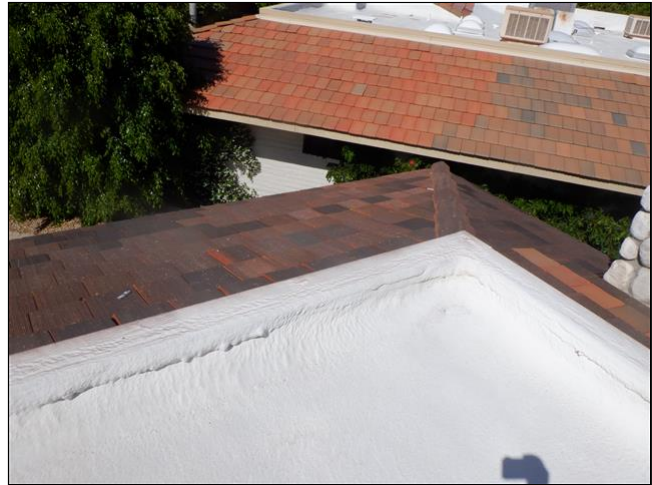
1.0 Item 2(Picture) Tile Roof Covering
