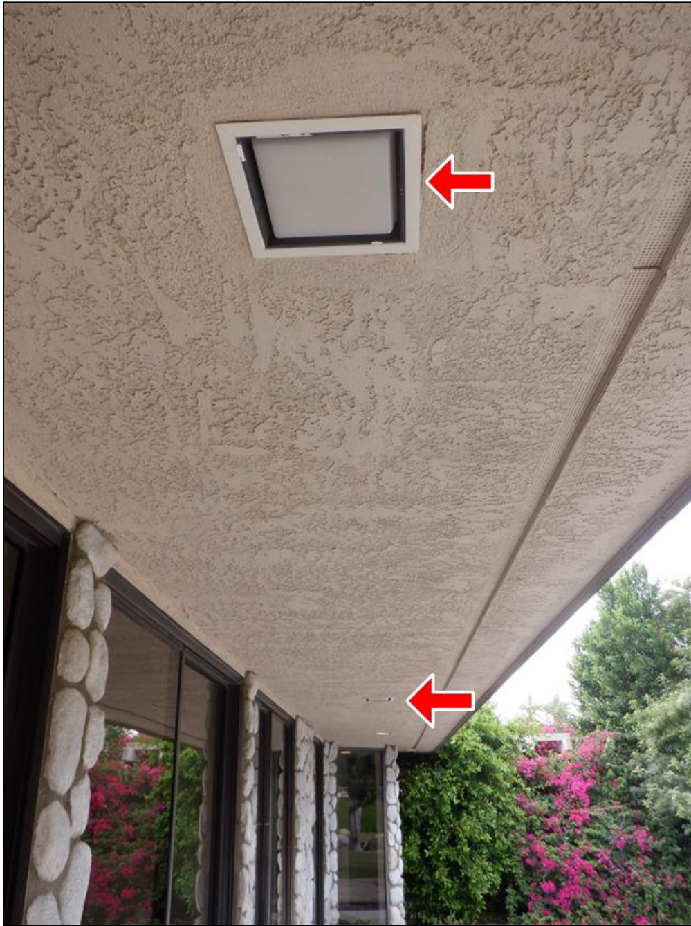
2.8 Item 2(Picture) Patio Light Fixtures Not Functioning
