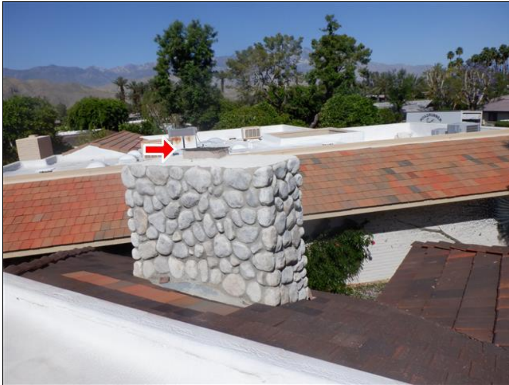
1.2 Item 1(Picture) Chimney Missing Rain Cap
