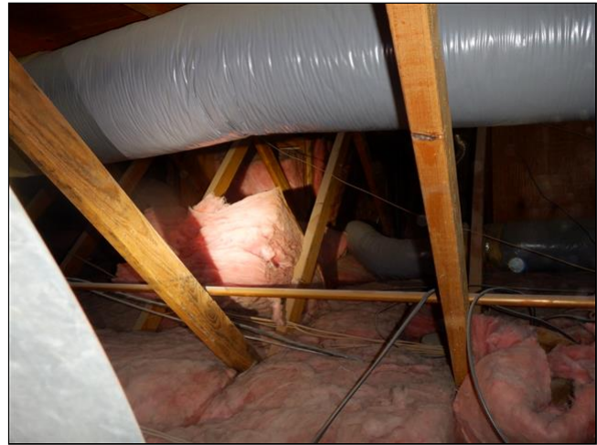
1.6 Item 2(Picture) Attic Insulation
