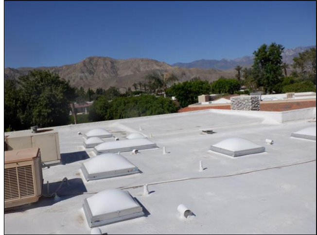
1.0 Item 13(Picture) Flat Roof Covering
