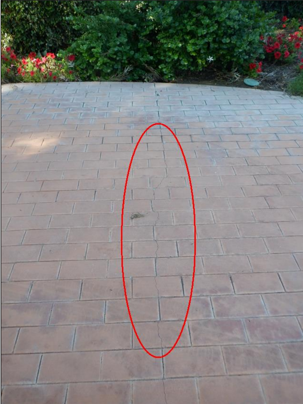
2.4 Item 2(Picture) Driveway Cracked Bricks
