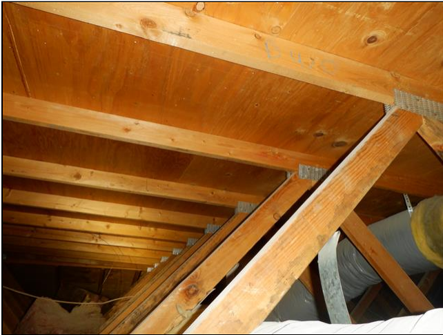
1.5 Item 3(Picture) Roof Framing/Roof Decking
