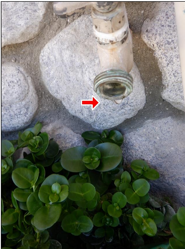
2.6 Item 2(Picture) Hose Bib Leak
