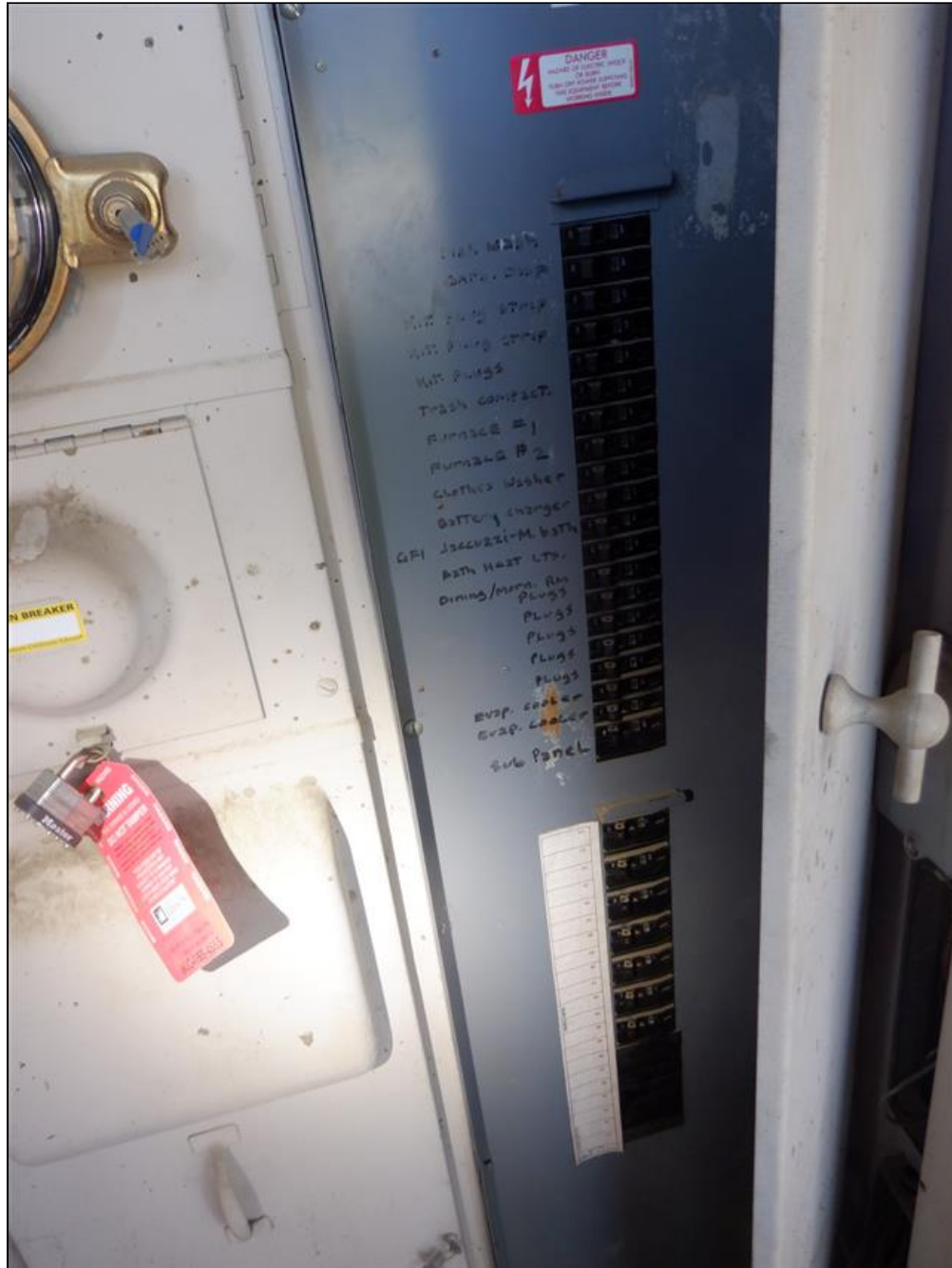
9.1 Item 2(Picture) Main Electrical Panel Distribution
