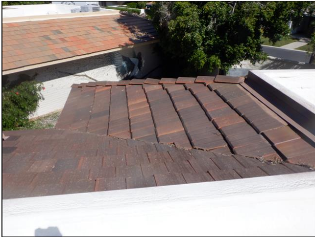
1.0 Item 1(Picture) Tile Roof Covering
