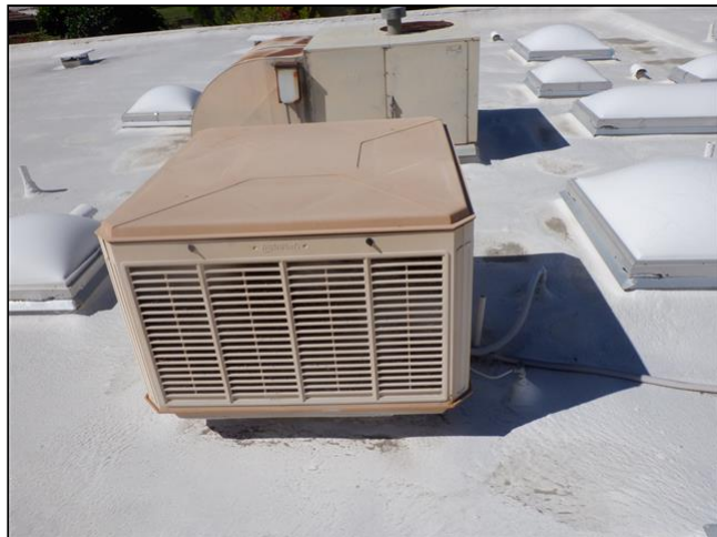
10.4.B Item 1(Picture) Evaporative Cooler 1
