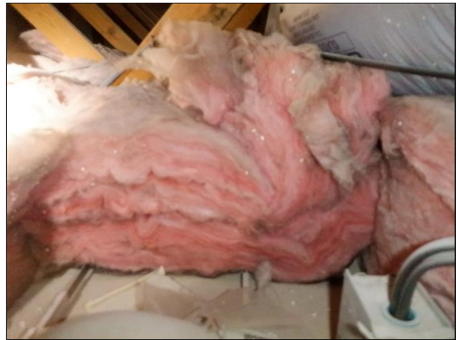
1.6 Item 4(Picture) Attic Insulation
