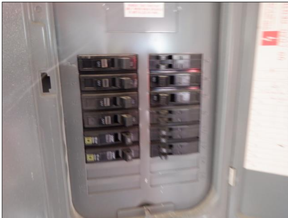
9.1 Item 8(Picture) Electrical Sub Panel Distribution
