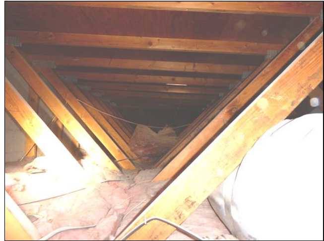
1.5 Item 4(Picture) Roof Framing/Roof Decking
