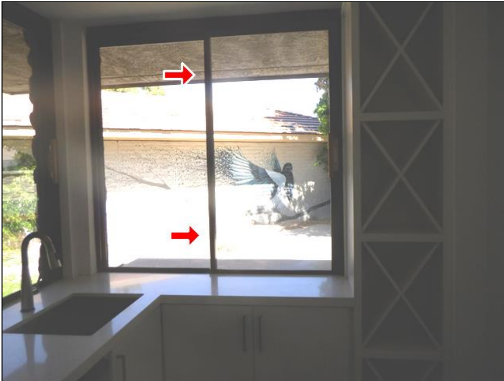
2.2 Item 5(Picture) Bar Window Inoperative
