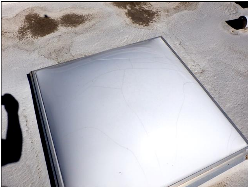
1.2 Item 2(Picture) Skylight 1 Cracked
