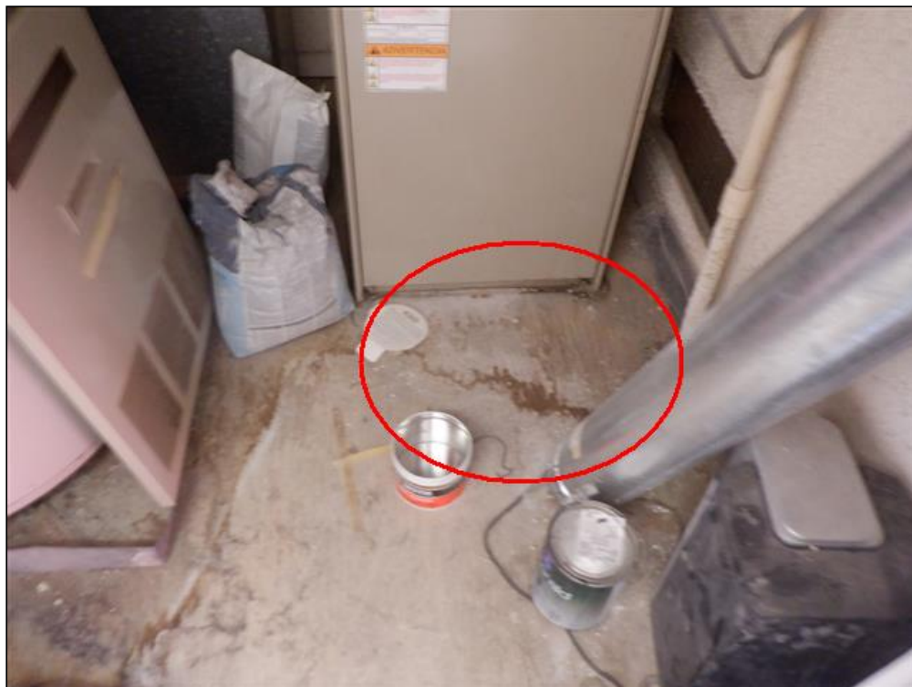
10.3.A Item 1(Picture) Moisture Stains Furnace Landing
