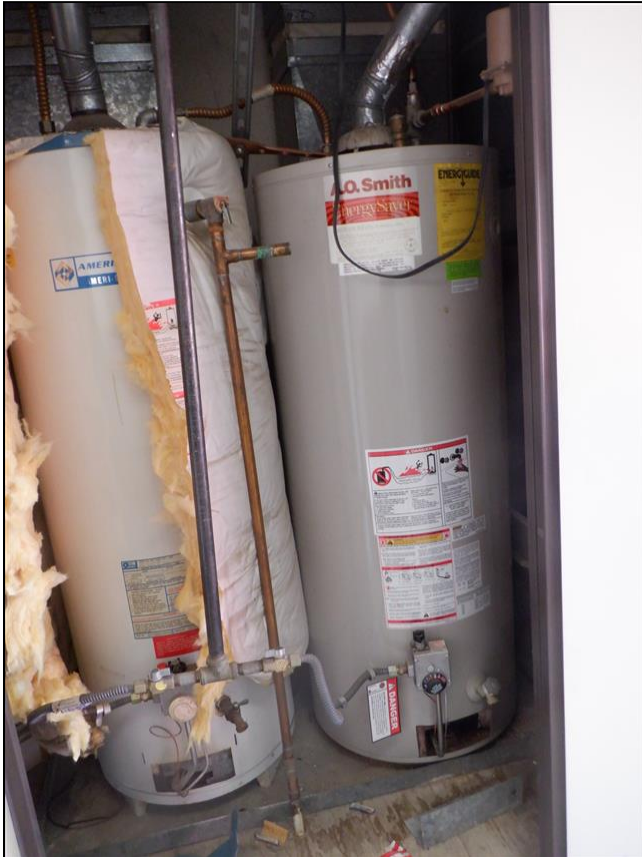
8.2 Item 1(Picture) Water Heaters
