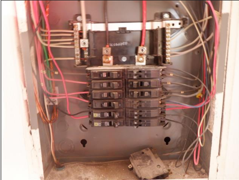
9.1 Item 9(Picture) Electrical Sub Panel Breakers/Conductors
