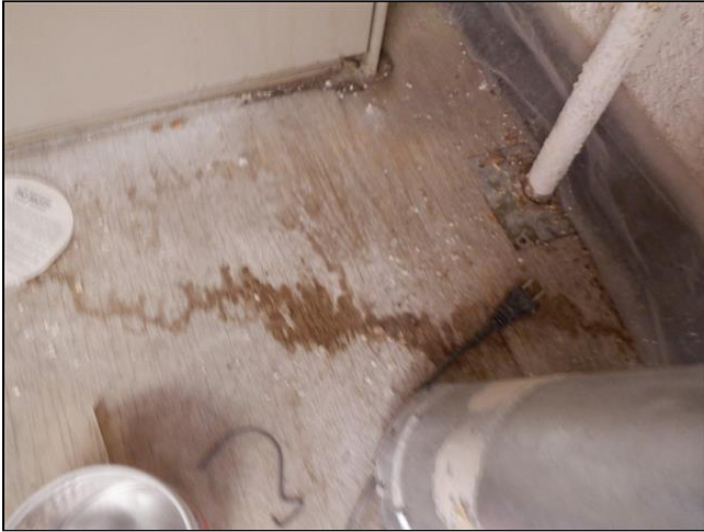
10.3.A Item 2(Picture) Moisture Stains Furnace Landing
