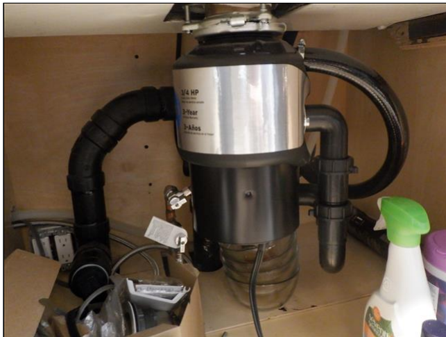
4.11 Item 1(Picture) Disposer No Activation Switch
