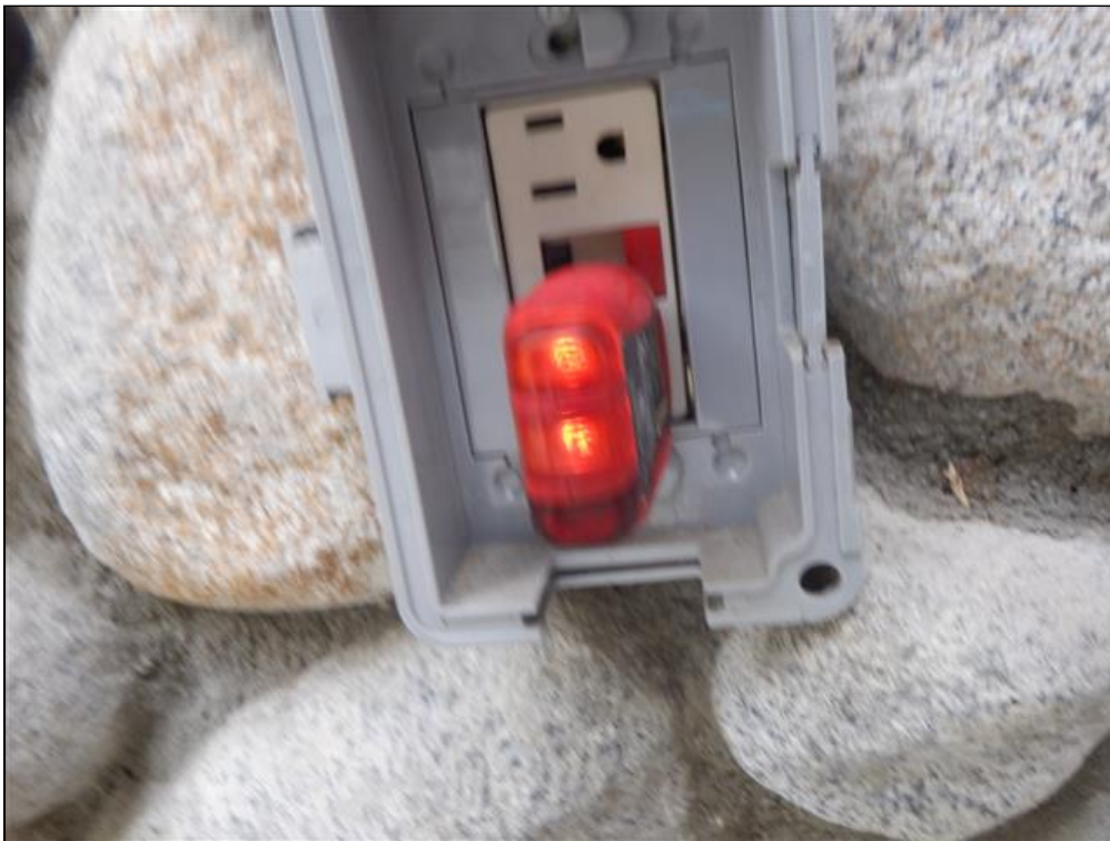
2.7 Item 2(Picture) GFCI Outlet Failed To Trip
