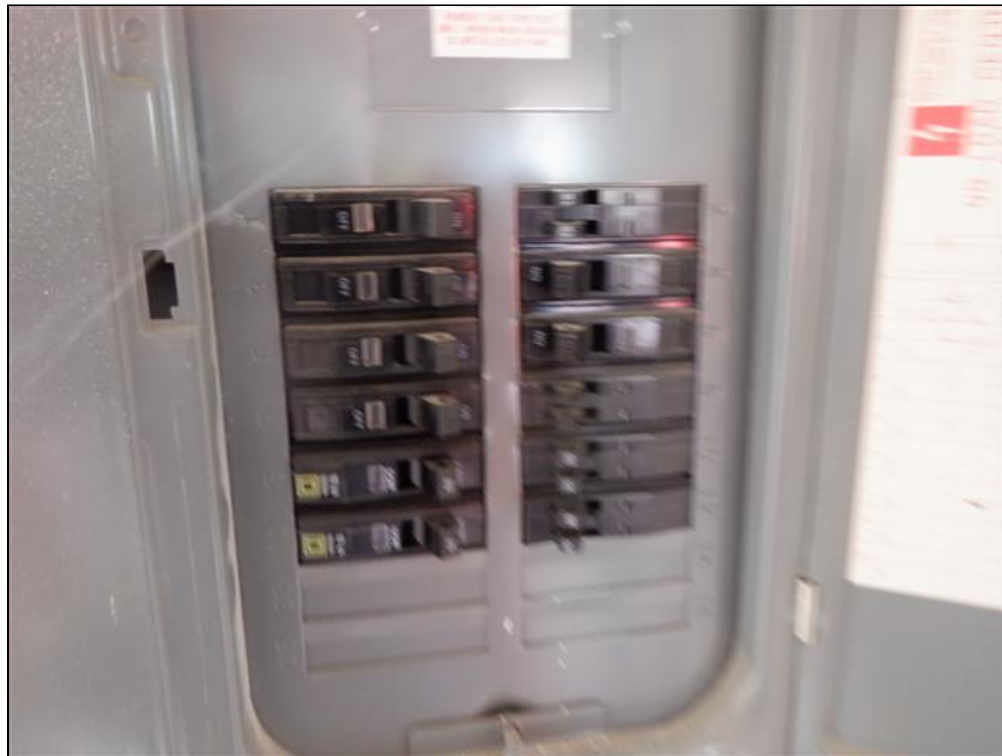
9.1 Item 8(Picture) Electrical Sub Panel Distribution
