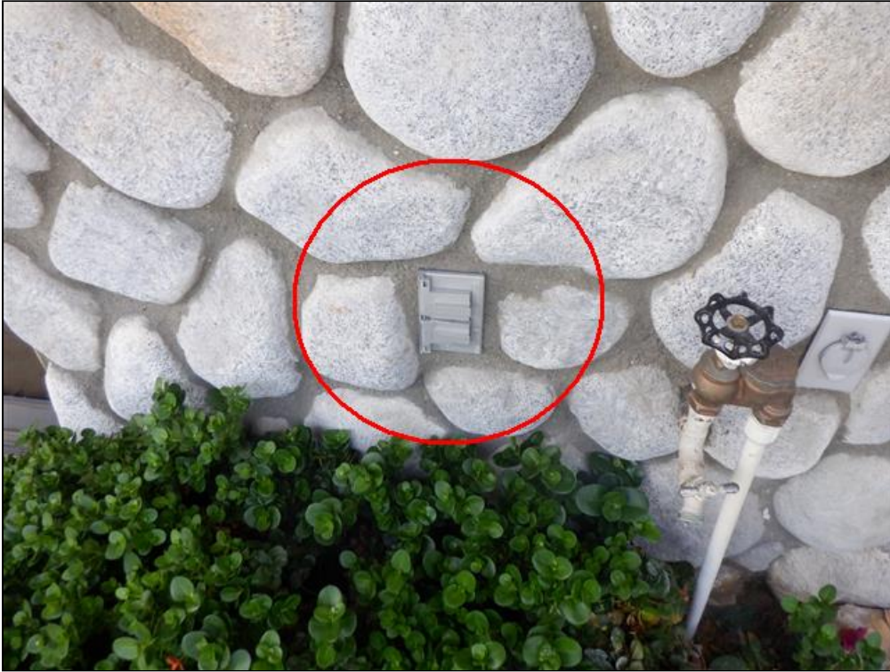
2.7 Item 6(Picture) West Patio Outlet No Power
