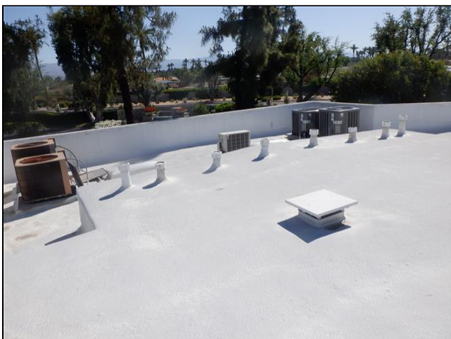
1.0 Item 16(Picture) Flat Roof Covering
