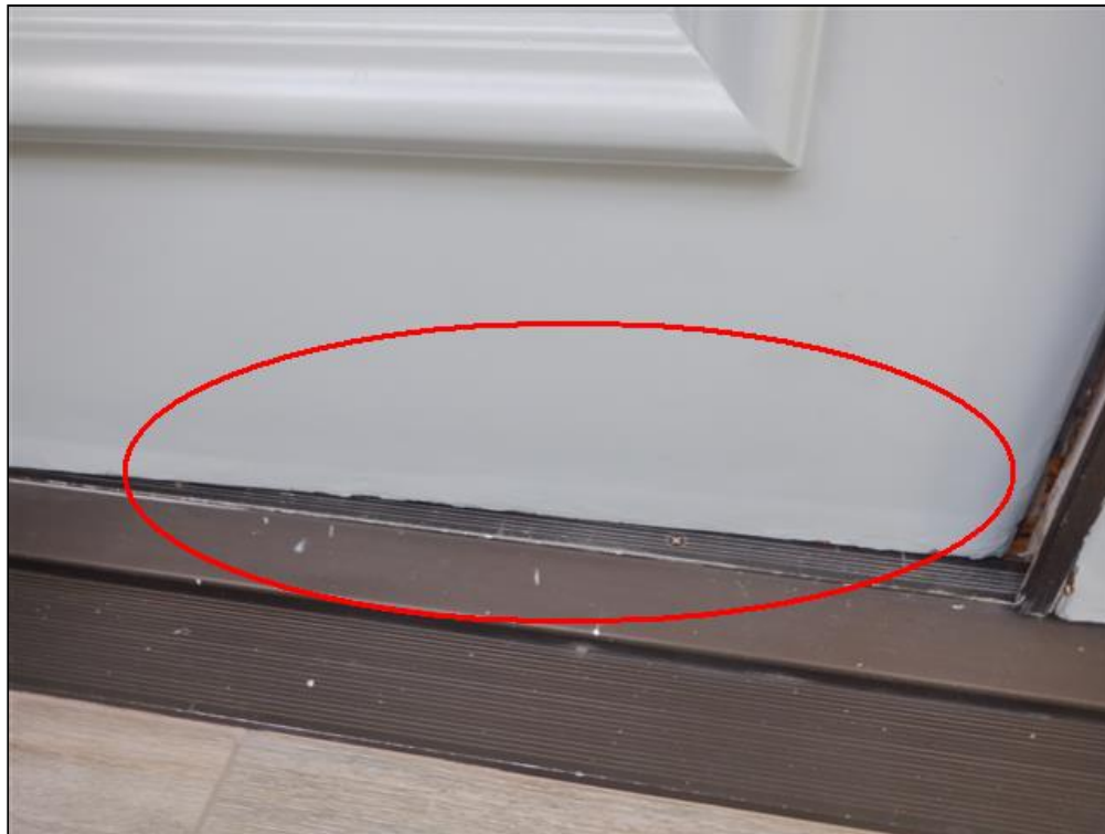
2.1 Item 3(Picture) Front Doors Weathered
