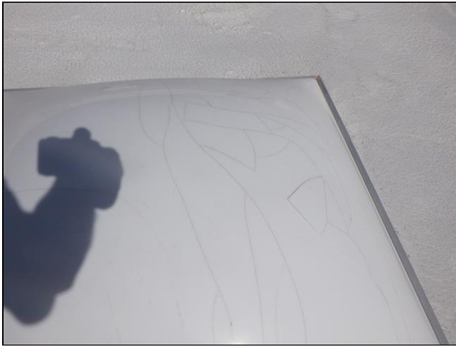
1.2 Item 7(Picture) Skylight 6 Cracked
