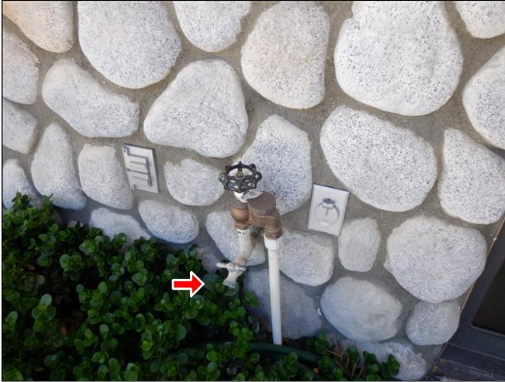
2.6 Item 1(Picture) Hose Bib Leak
