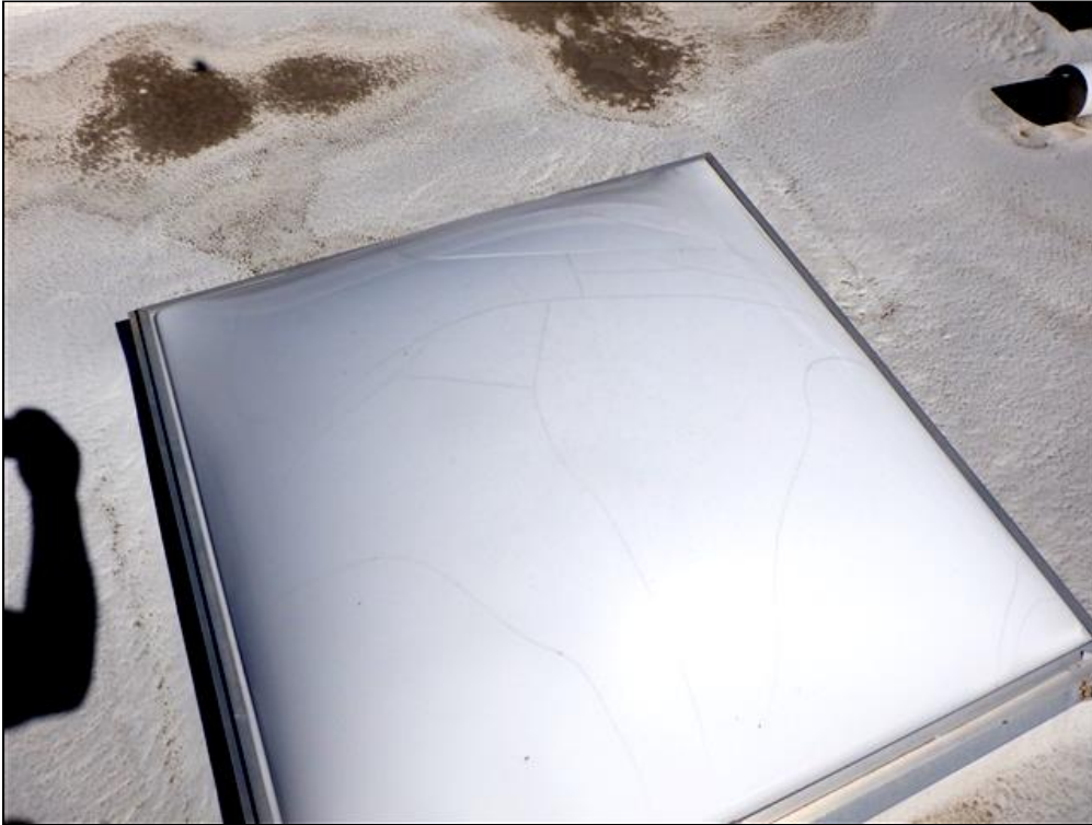
1.2 Item 2(Picture) Skylight 1 Cracked
