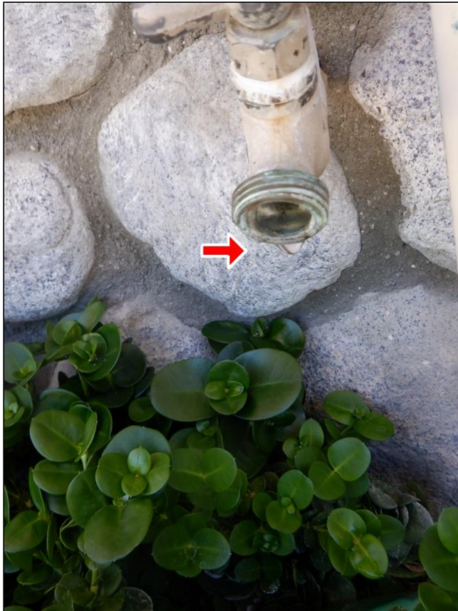
2.6 Item 2(Picture) Hose Bib Leak
