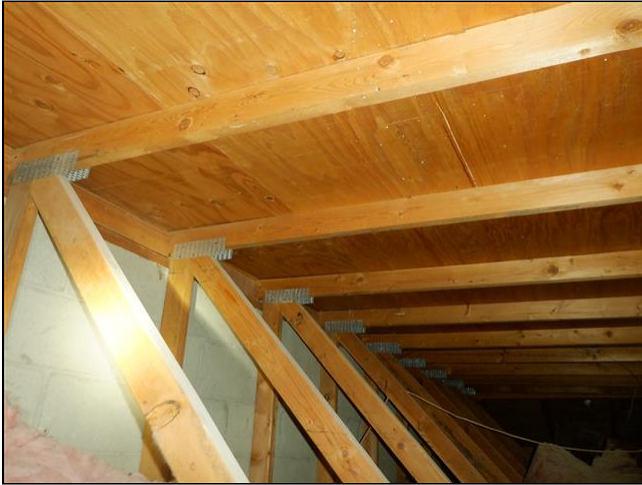
1.5 Item 1(Picture) Roof Framing/Roof Decking
