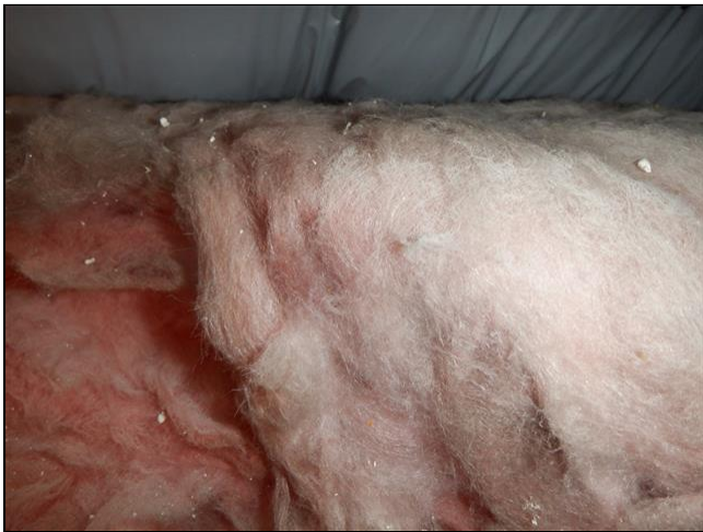
1.6 Item 3(Picture) Attic Insulation
