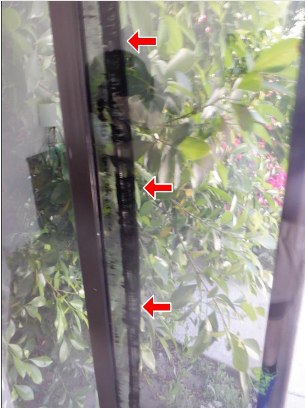
2.2 Item 2(Picture) Master Bedroom Slider Bad Seal
