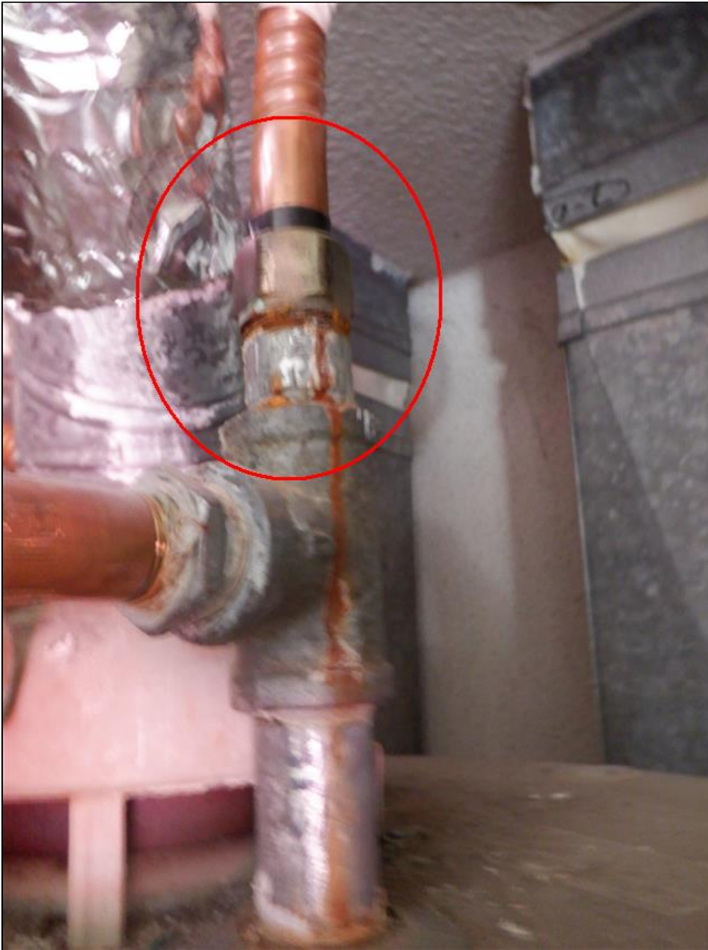
8.2 Item 5(Picture) Copper/Galvanized Pipe
