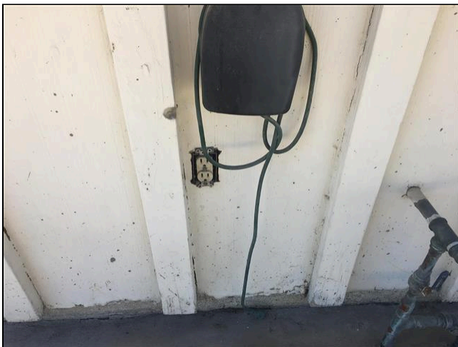
6.4 Item 1(Picture) weather cover missing
