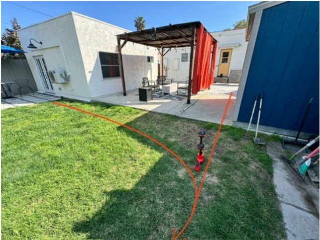
Location where front house and ADU sewer lines tie in together.
