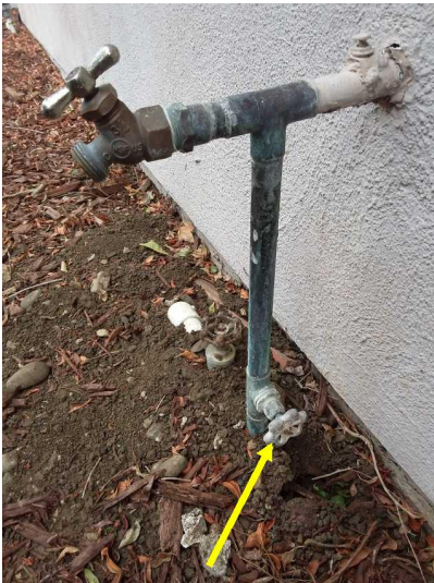
The main water shut-off valve is located at the front of the house.
