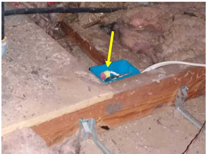
There are open electrical junction boxes, which should be sealed to contain any arcing or sparking that might occur.
