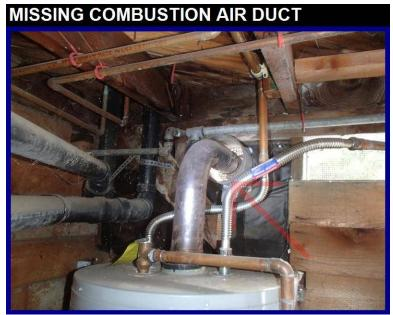
[SC] The flue vent pipe is installed with a material that was not rated for this application. We recommend replacing this material with an approved product, using approved methods for safety reasons.
