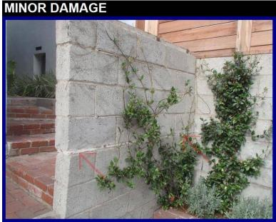
[CR] The concrete block fencing had common settlement or movement cracks. We recommend it be monitored and repaired if further damage develops
