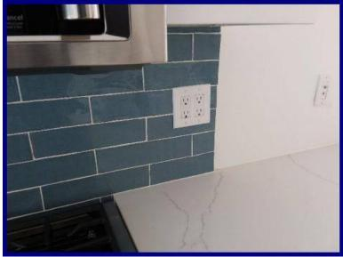
[SC] The accessible receptacles are not GFCI protected, GFCI protected outlets should have been installed at the time the building was remodeled. This is an electrical Safety Hazard. We recommend providing GFCI protection at the required locations for safety reasons.
