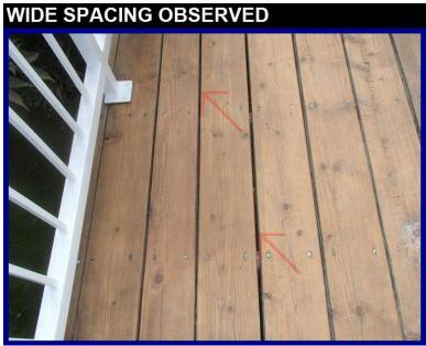
[SC] The spacing between the deck boards is installed with large gaps between the boards. This is a safety concern especially for woman with high heels. Generally industry standards dictate a gap of 1/8th of an inch between boards for the expansion and contraction of the boards as well as to vent the moisture. The current installation is a safety concern. We recommend the boards be installed with no more than an 1/8th of an inch gap for a safe walking surface.
