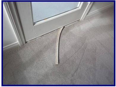
[CR] There is evidence of moisture intrusion at the base and threshold of the exterior exit door(s). We recommend locating and repairing the source and any damaged materials.
