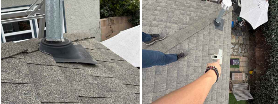
Exposed Fasteners
